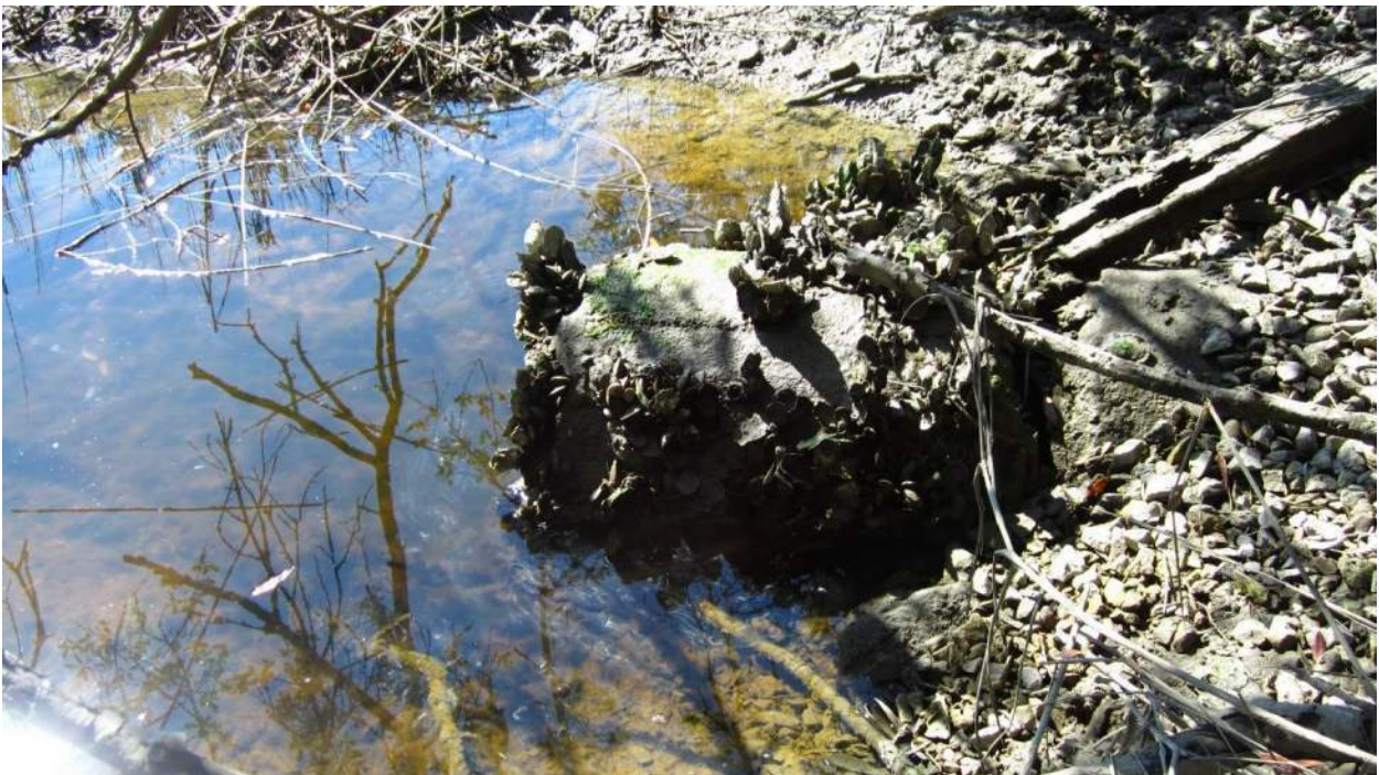
Inlet end of Spanish Moss Trail 24-in crossline pipe
