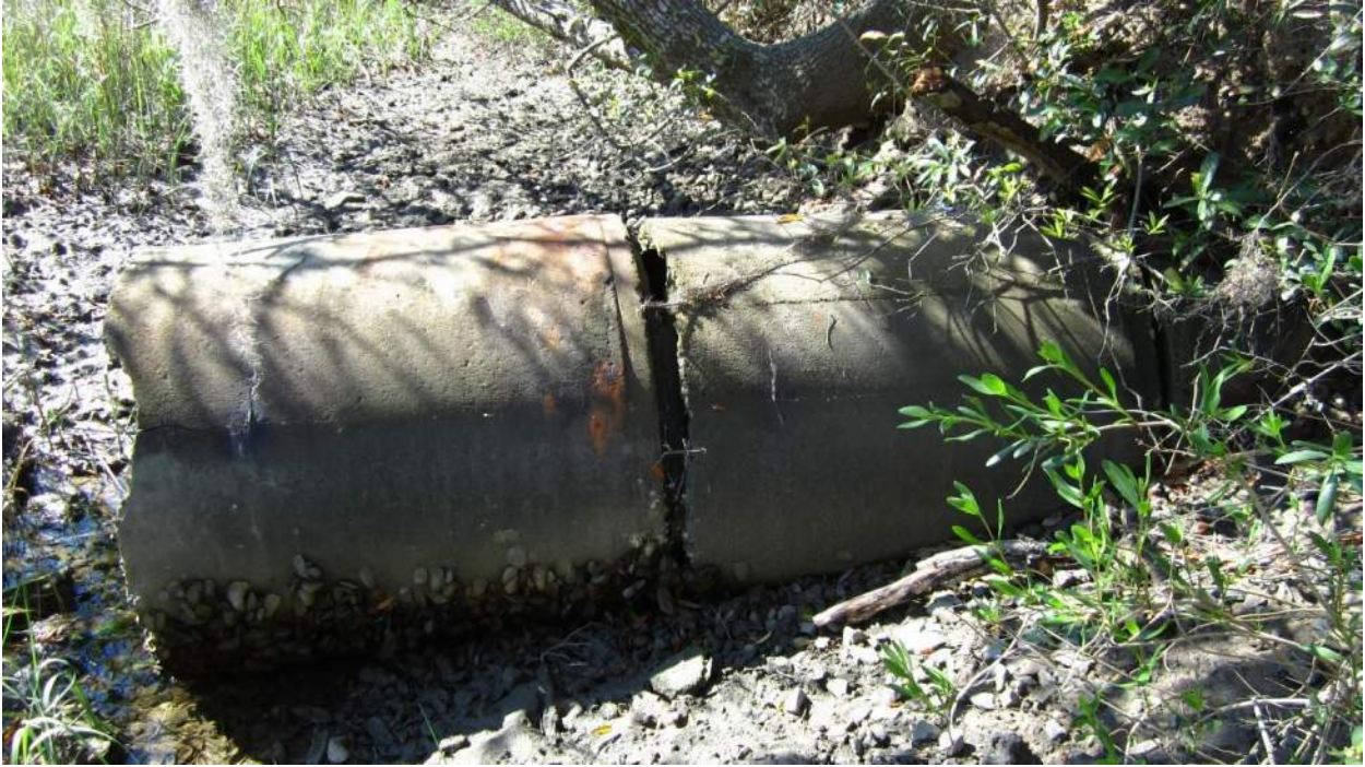
Inlet end of Spanish Moss Trail 36-in crossline pipe
