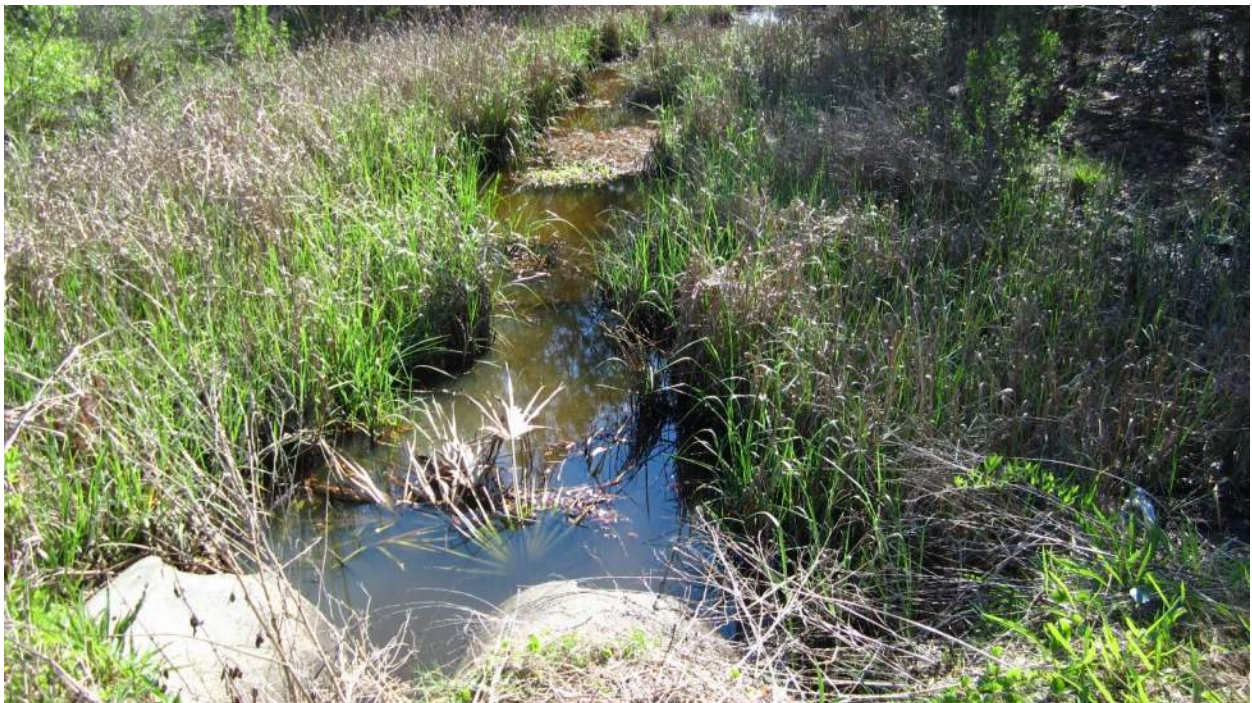
Main ditch upstream of Battery Creek Road crossline pipes
