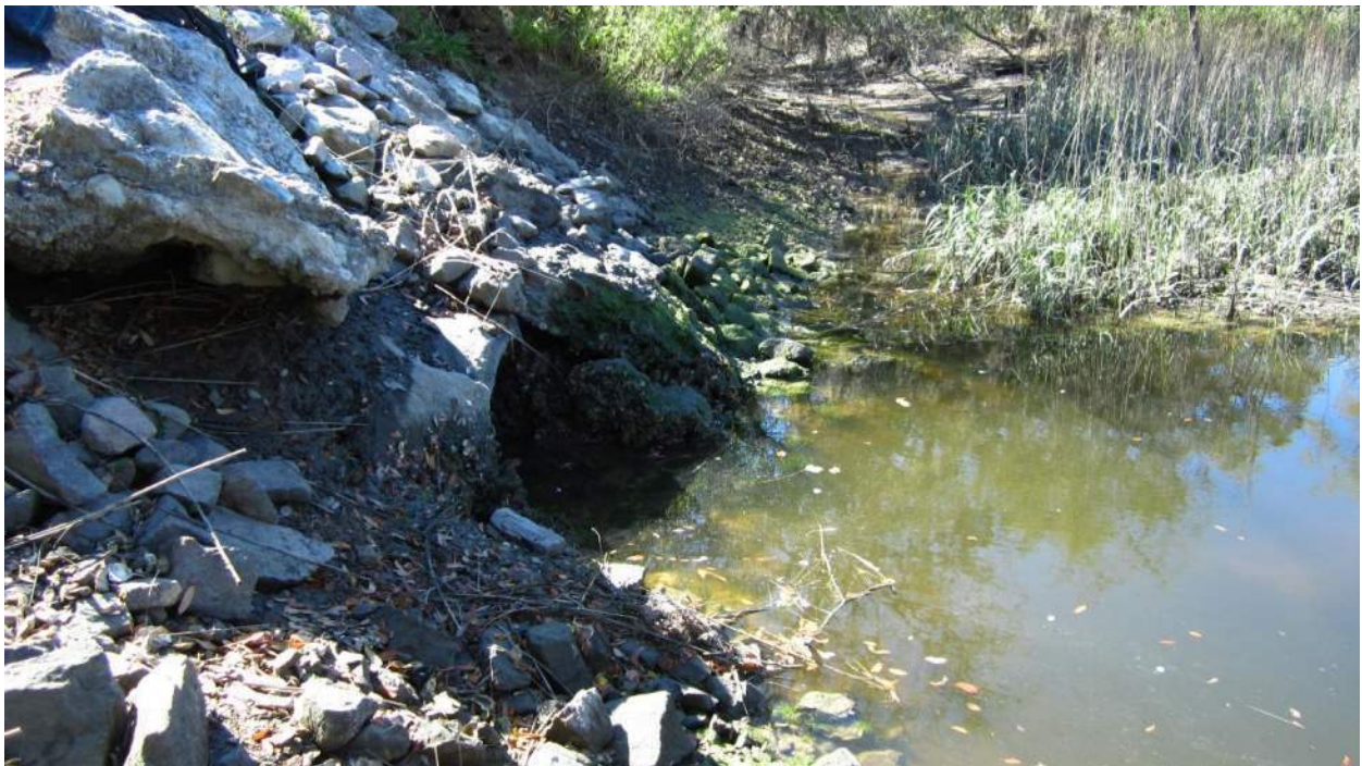
Downstream (Battery Creek) end of Spanish Moss Trail 36-in crossline pipe
