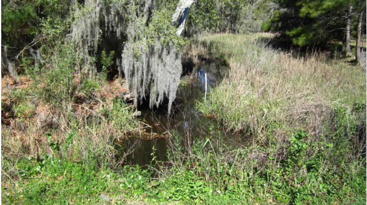
Main ditch downstream of Battery Creek Road crossline pipes
