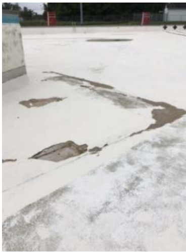
Expansion joint under gutter
