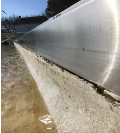
Expansion joint under gutter
