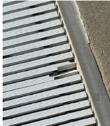
grating over gutter at zero depth
