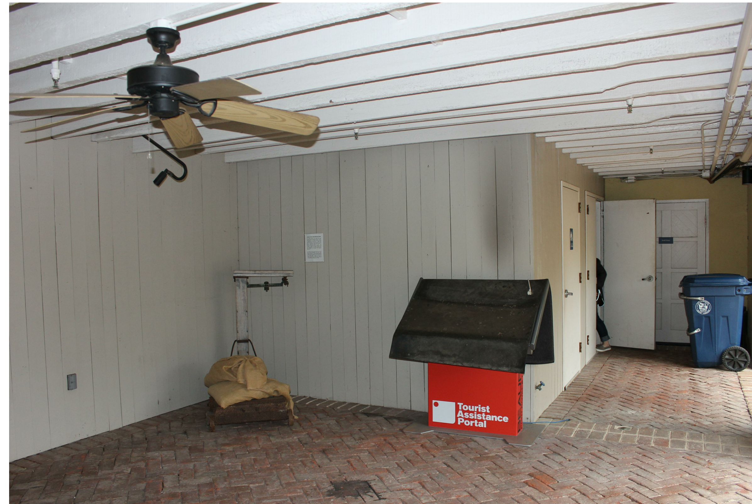
EXISTING CONDITIONS- EXTERIOR OF ADA RESTROOM NOT TO SCALE
