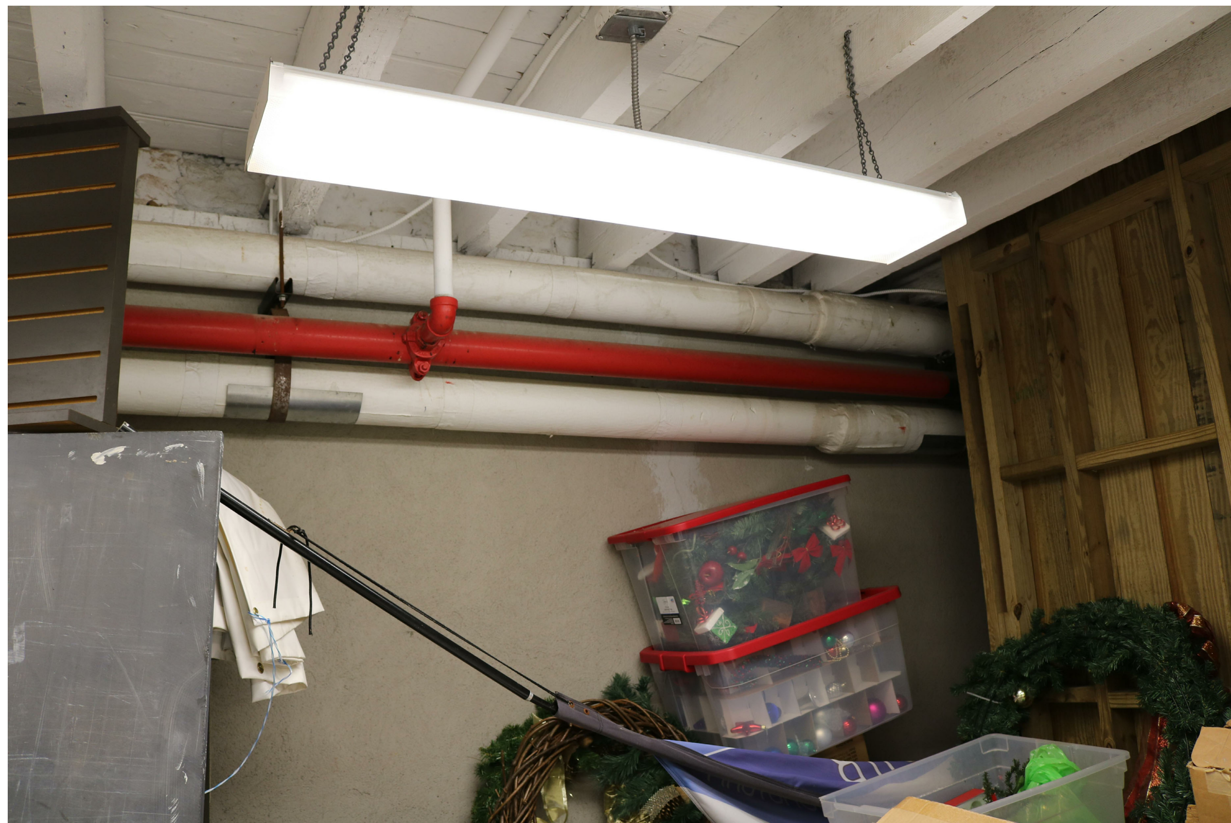
EXISTING CONDITIONS- INTERIOR OF STORAGE ROOM NOT TO SCALE
