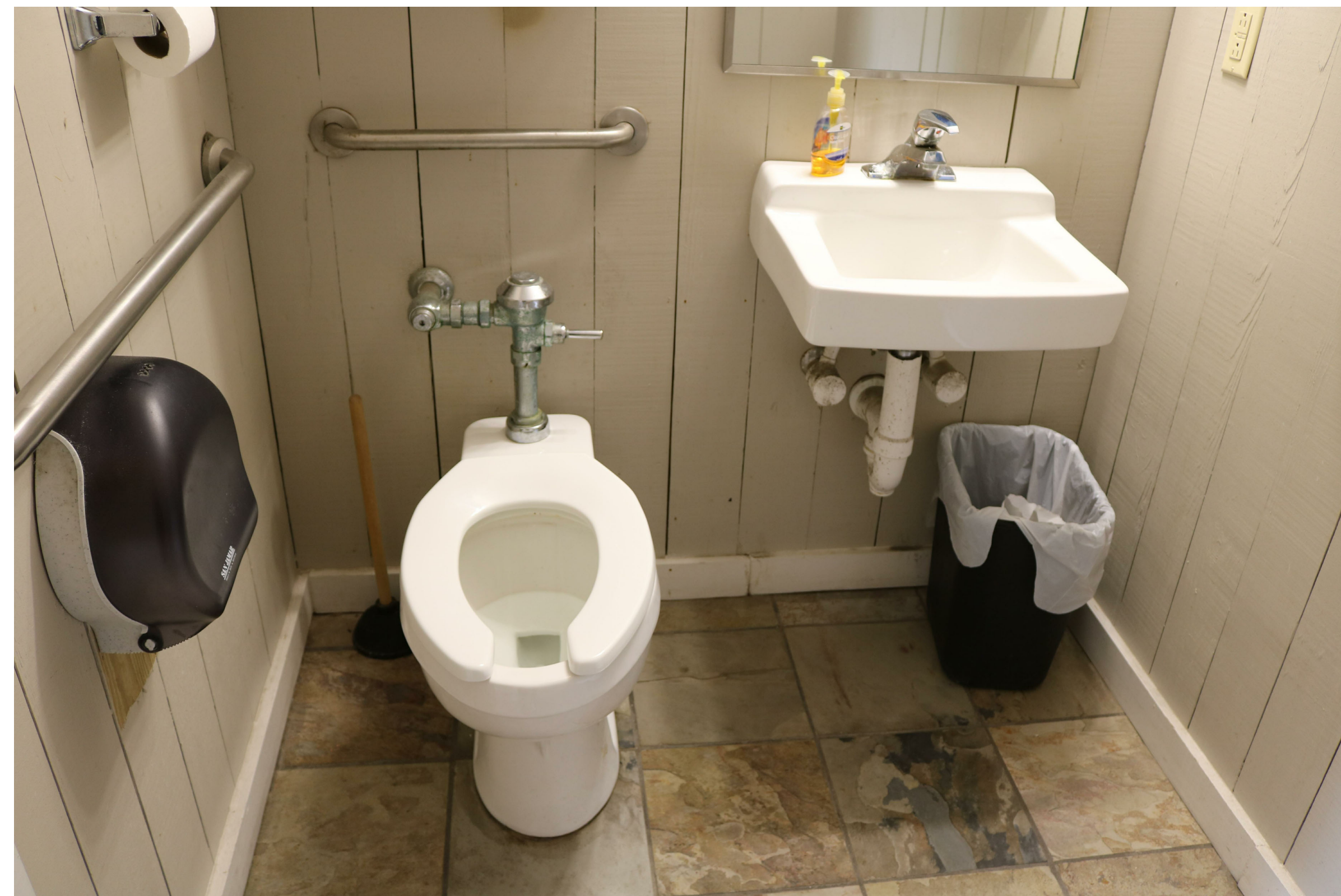
EXISTING CONDITIONS- INTERIOR OF ADA RESTROOM NOT TO SCALE
