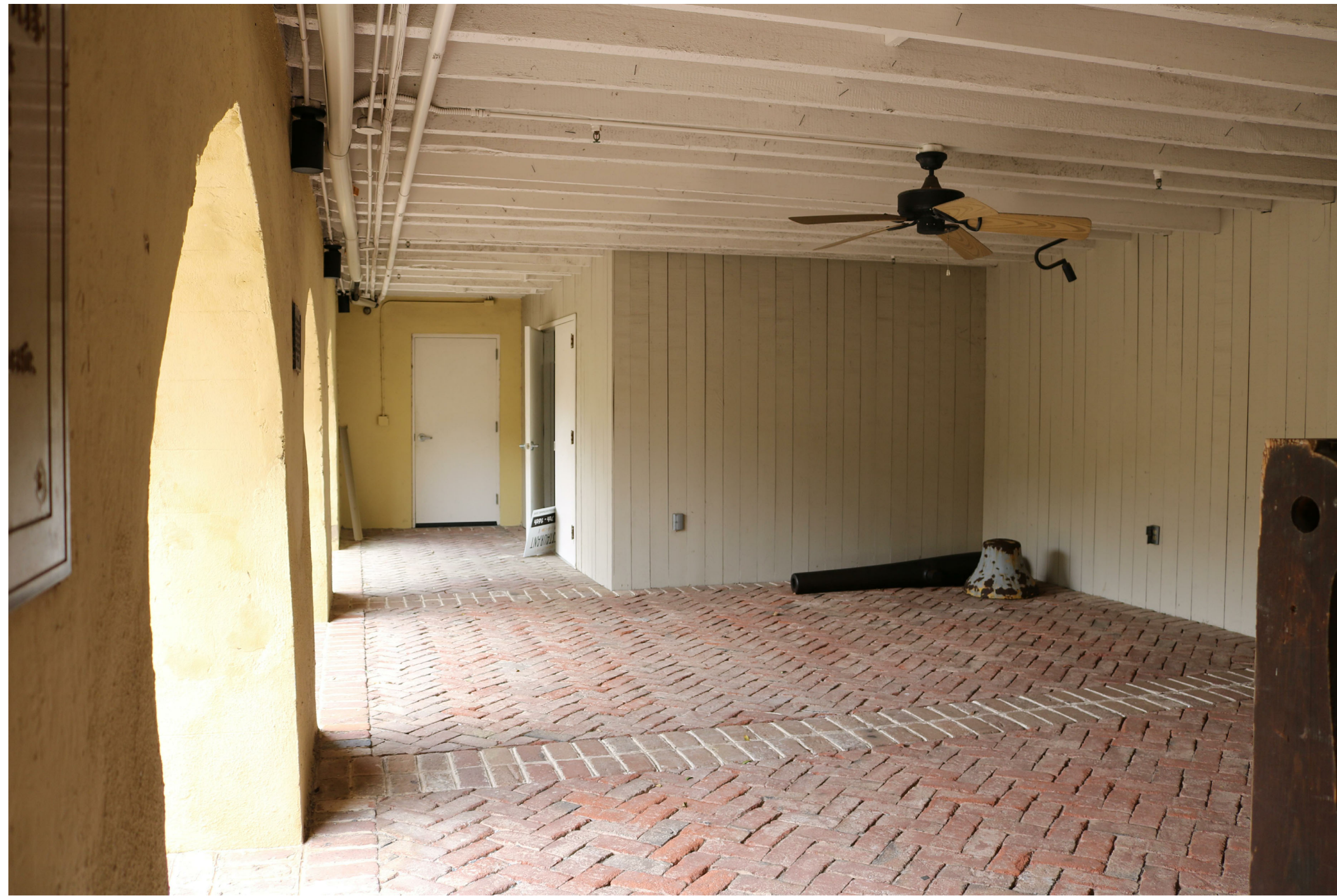
EXISTING CONDITIONS- EXTERIOR OF STORAGE ROOM NOT TO SCALE
