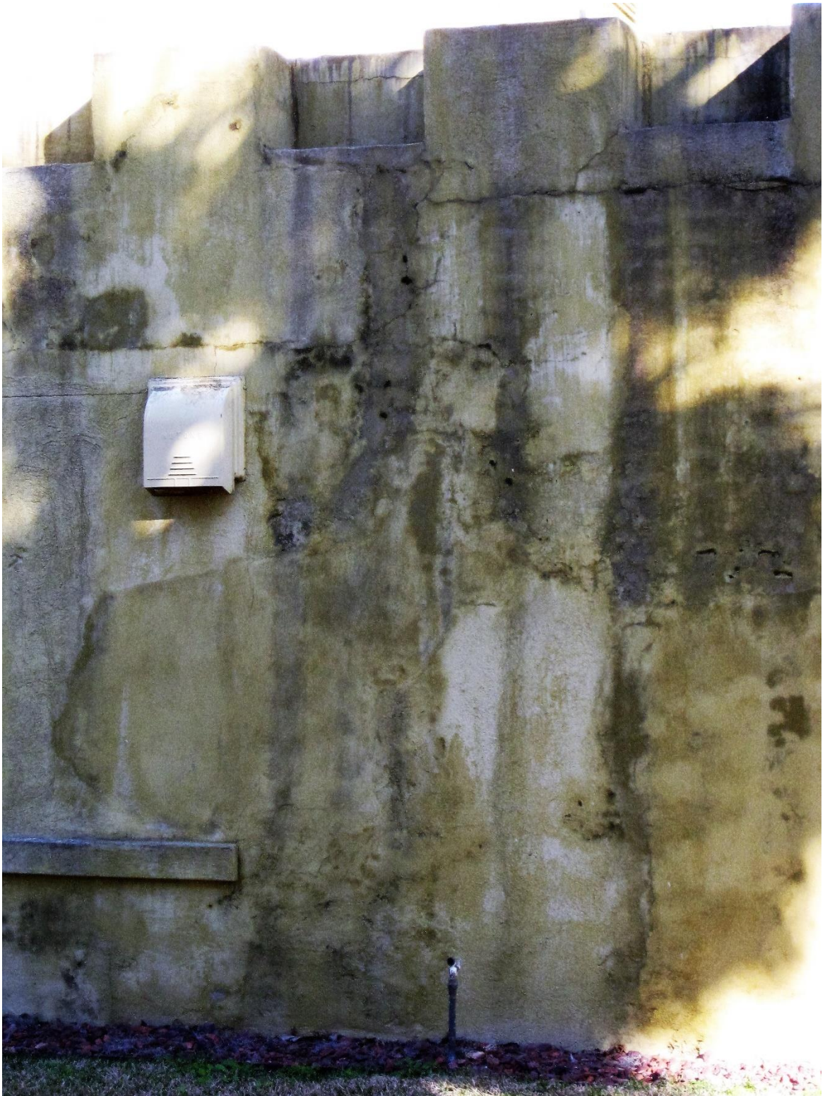
B1. West Outer Wall
