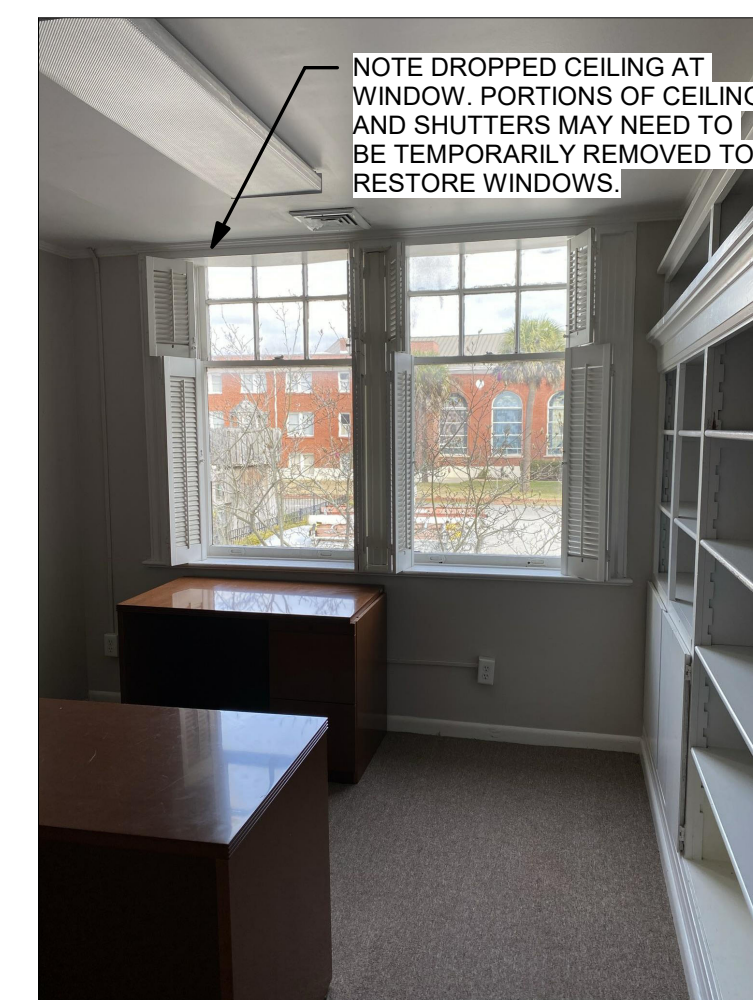
EXISTING CONDITIONS- OFFICE ROOM 104
