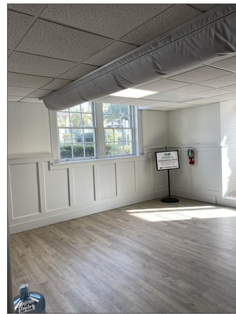
EXISTING CONDITIONS- WINDOWS #5 & 6
