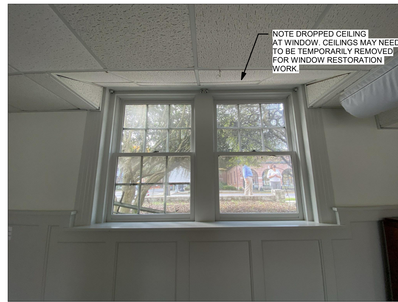
EXISTING CONDITIONS- WINDOWS #3 & 4
