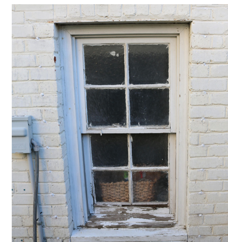
E BASEMENT SINGLE DOUBLE HUNG WINDOW (REPLACEMENT) REFERENCE PHOTOGRAPH WINDOW TYPE IS EXISTING. TYPE E IS FOUND ON WINDOWS 10.
