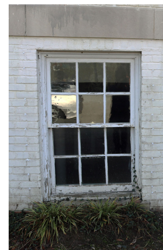
C BASEMENT SINGLE DOUBLE HUNG WINDOW (HISTORIC) REFERENCE PHOTOGRAPH WINDOW TYPE IS EXISTING. TYPE C IS FOUND ON WINDOWS 7.
