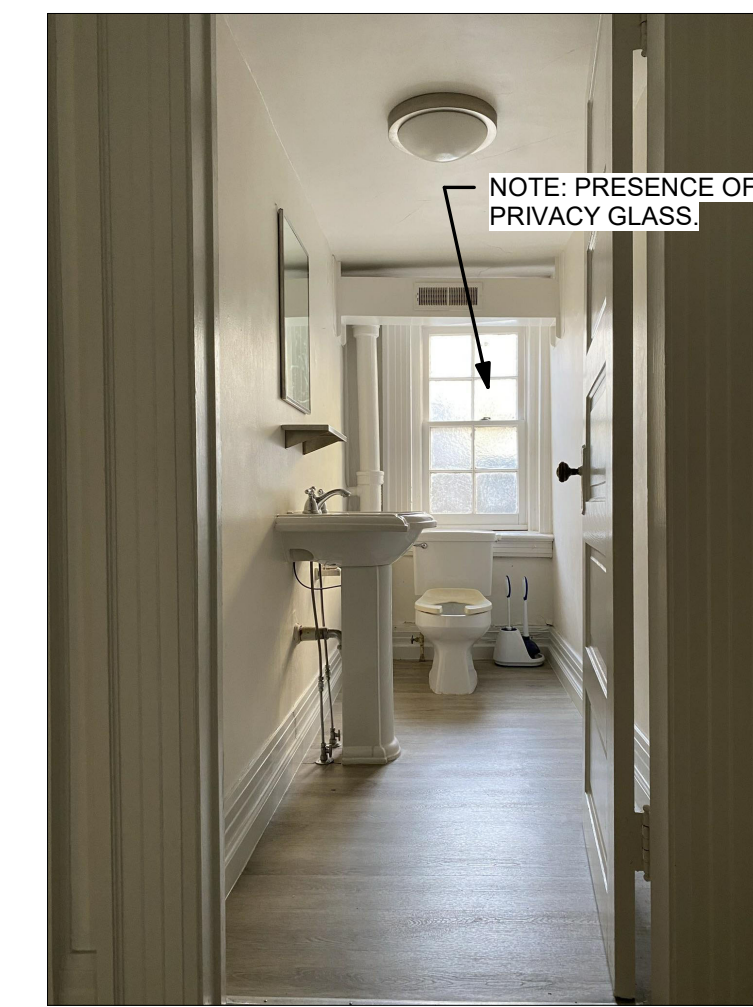
EXISTING CONDITIONS- RESTROOM ROOM 006
