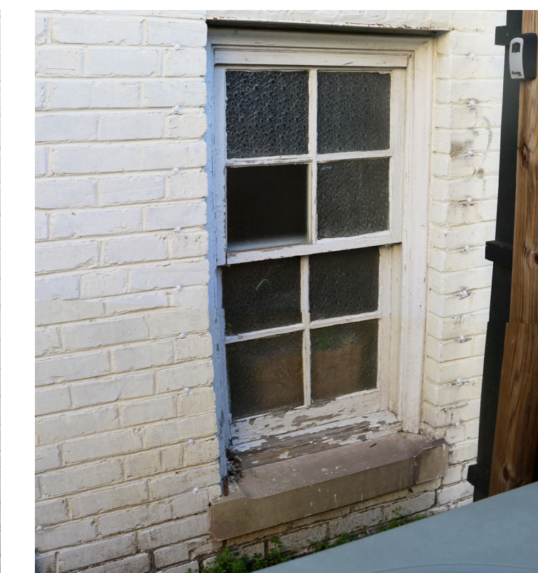
F BASEMENT SINGLE DOUBLE HUNG WINDOW (HISTORIC) REFERENCE PHOTOGRAPH WINDOW TYPE IS EXISTING. TYPE F IS FOUND ON WINDOWS 11.
