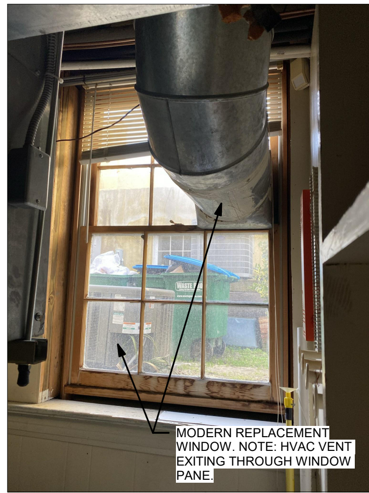
EXISTING CONDITIONS- WINDOW #9
