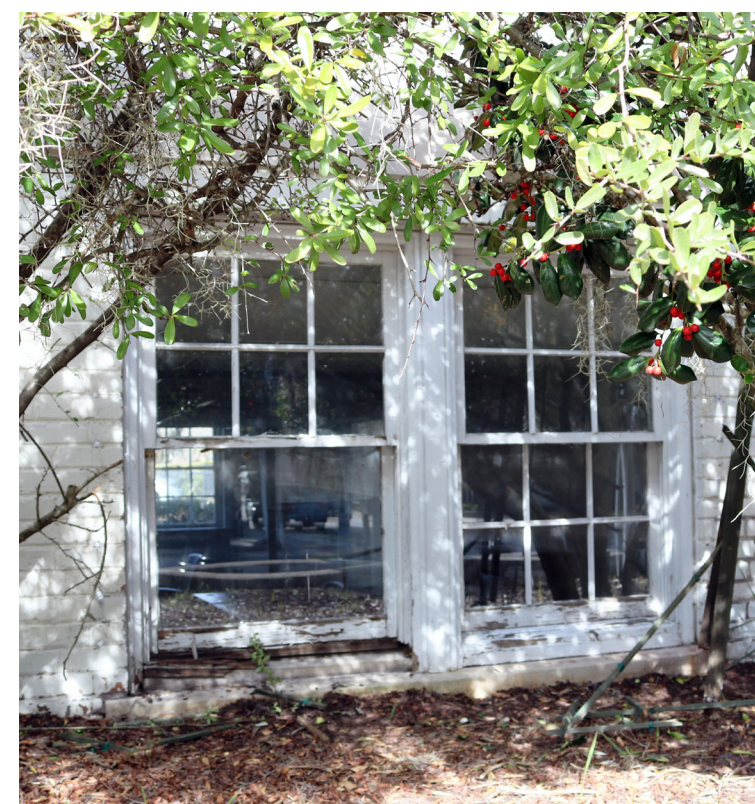
B BASEMENT PAIR OF DOUBLE HUNG WINDOWS (MODERN REPLACEMENT) REFERENCE PHOTOGRAPH WINDOW TYPE IS EXISTING. TYPE B IS FOUND ON WINDOWS 3 & 4.
