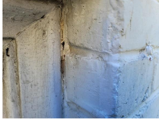
HOMOGENEOUS AREA 02 EXTERIOR WINDOW CAULK
