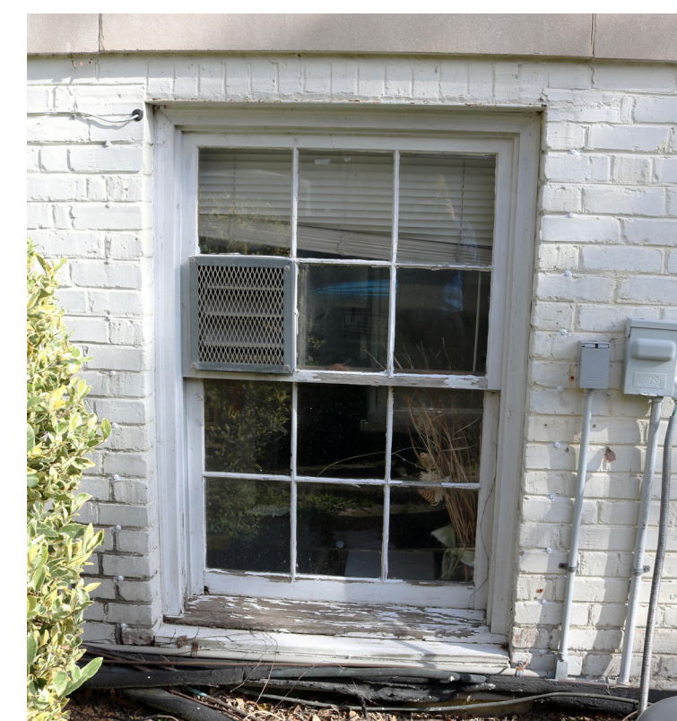
D BASEMENT SINGLE DOUBLE HUNG WINDOW (MODERN REPLACEMENT) REFERENCE PHOTOGRAPH WINDOW TYPE IS EXISTING. TYPE D IS FOUND ON WINDOWS 9.
