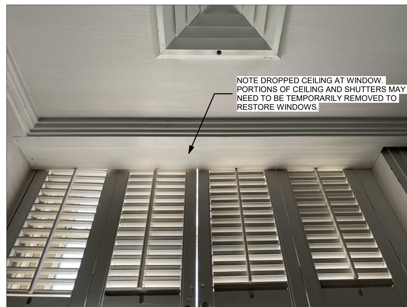
EXISTING CONDITIONS- OFFICE ROOM 106
