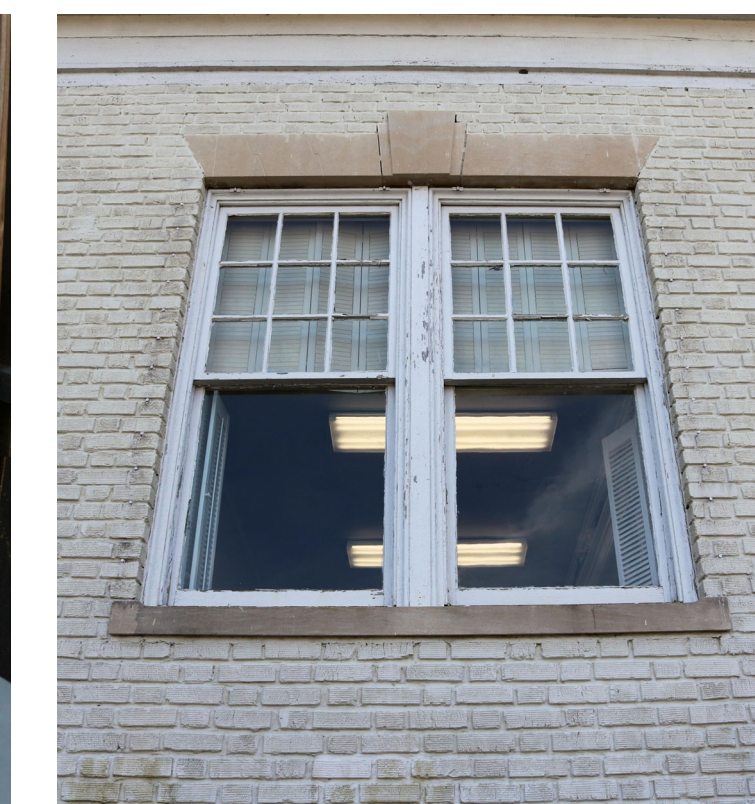
G 1ST FLOOR PAIR OF DOUBLE HUNG WINDOWS (HISTORIC) REFERENCE PHOTOGRAPH WINDOW TYPE IS EXISTING. TYPE G IS FOUND ON WINDOWS 12, 13, 14, 15, 16, 17, 18, 19, 20, 21, 22, 23, 24, & 25
