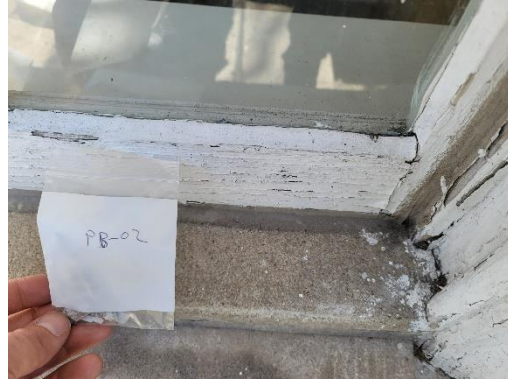
PB - 02 EXTERIOR WOOD WINDOW SILL & FRAME (WHITE)
