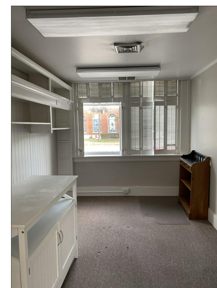
EXISTING CONDITIONS- OFFICE ROOM 103
