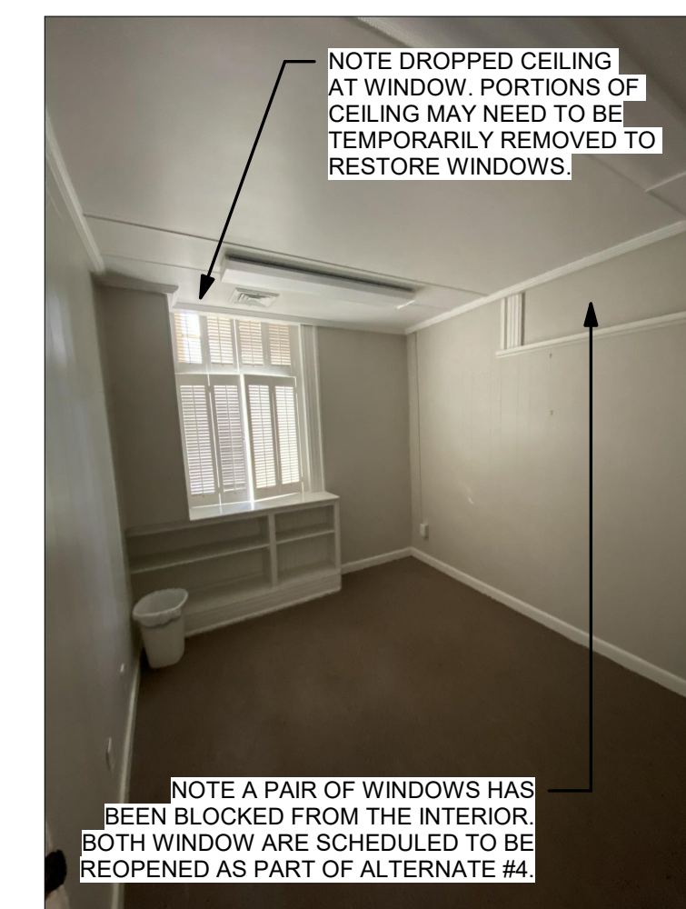
EXISTING CONDITIONS- OFFICE ROOM 106
