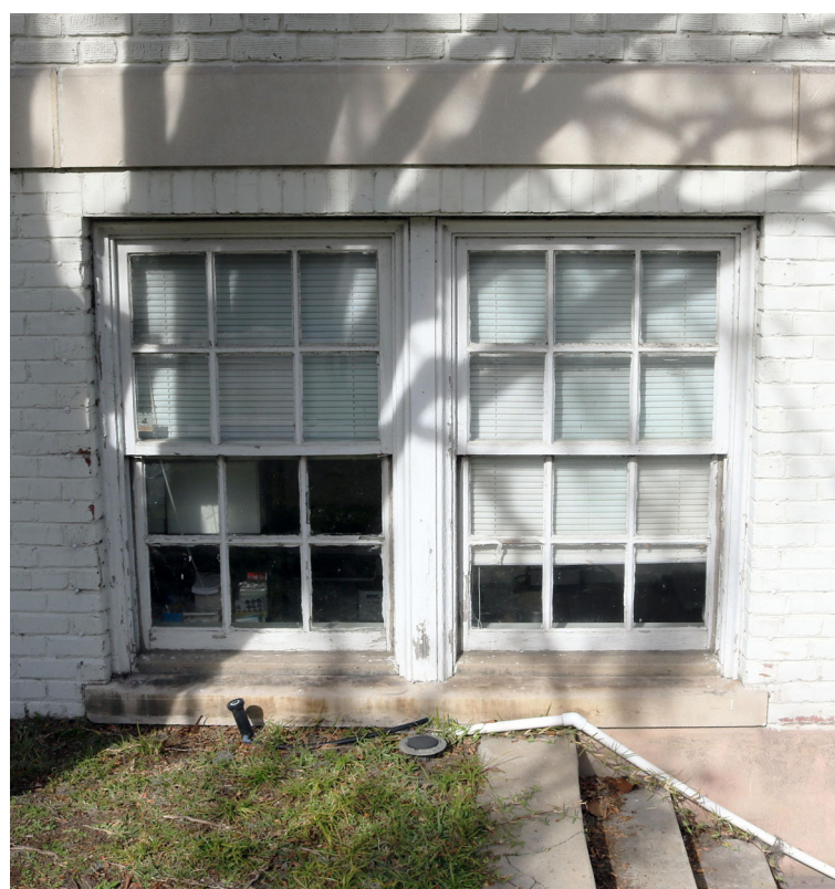
A BASEMENT PAIR OF DOUBLE HUNG WINDOWS (HISTORIC) REFERENCE PHOTOGRAPH WINDOW TYPE IS EXISTING. TYPE A IS FOUND ON WINDOWS 1, 2, 5, & 6.
