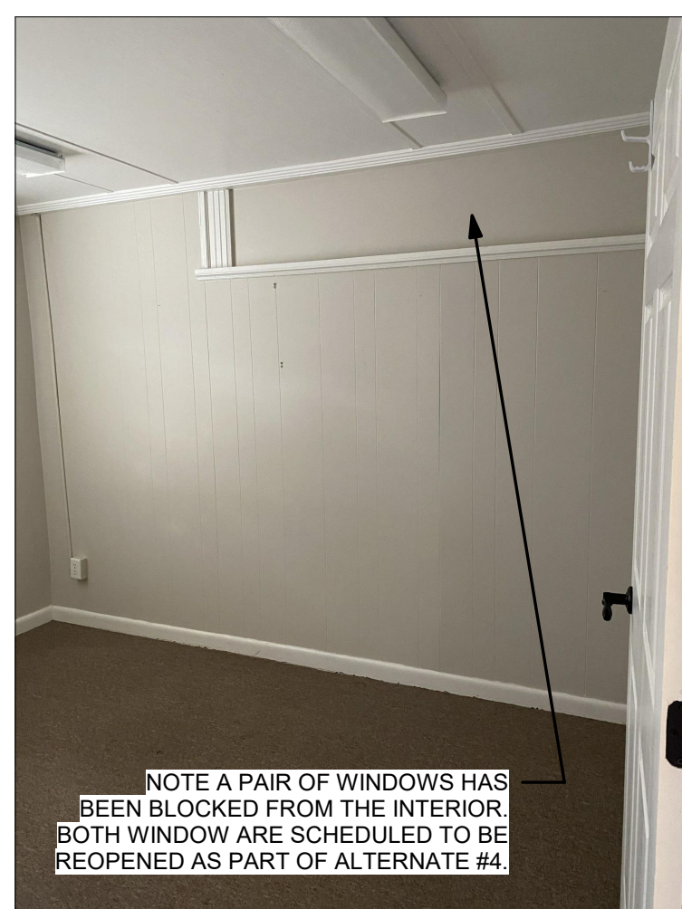
EXISTING CONDITIONS- OFFICE ROOM 106
