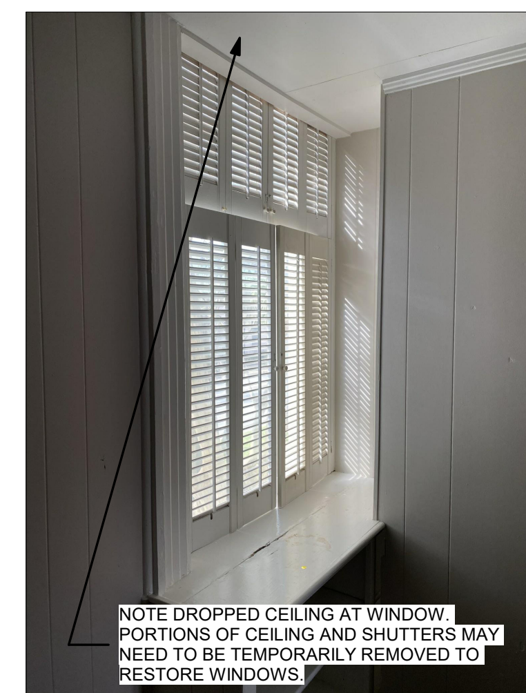
EXISTING CONDITIONS- OFFICE ROOM 107
