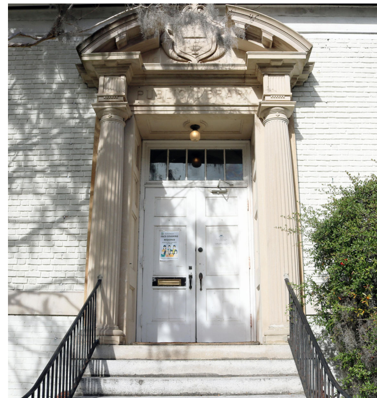
AA ENTRY DOUBLE DOOR 001 REFERENCE PHOTOGRAPH DOOR TYPE IS EXISTING.
