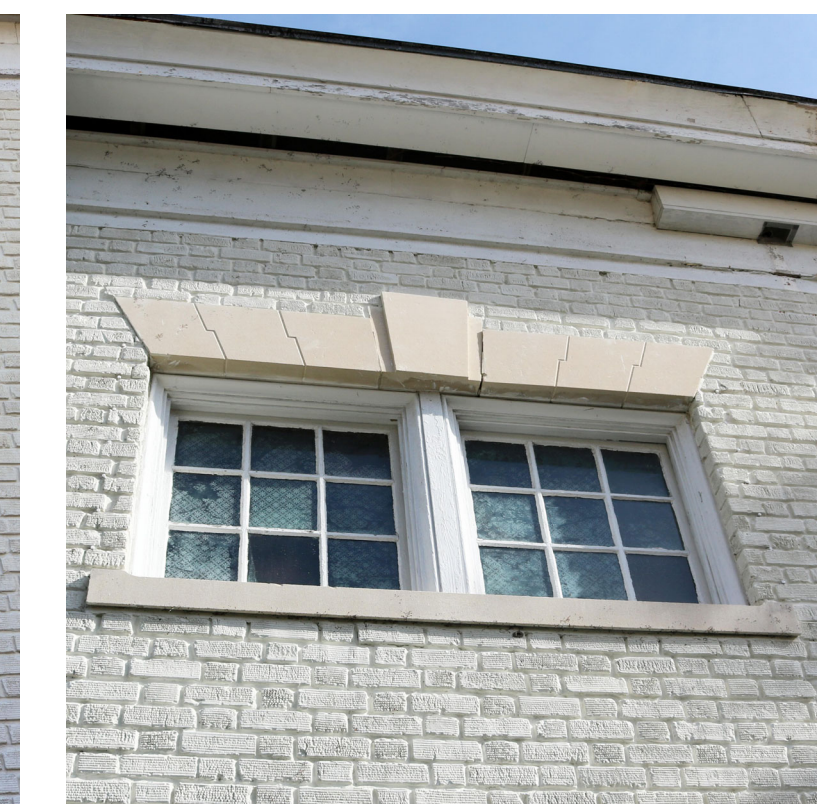
H 1ST FLOOR PAIR OF DOUBLE HUNG WINDOWS (HISTORIC) REFERENCE PHOTOGRAPH WINDOW TYPE IS EXISTING. TYPE H IS FOUND ON WINDOWS 26, 27, 28, & 29
