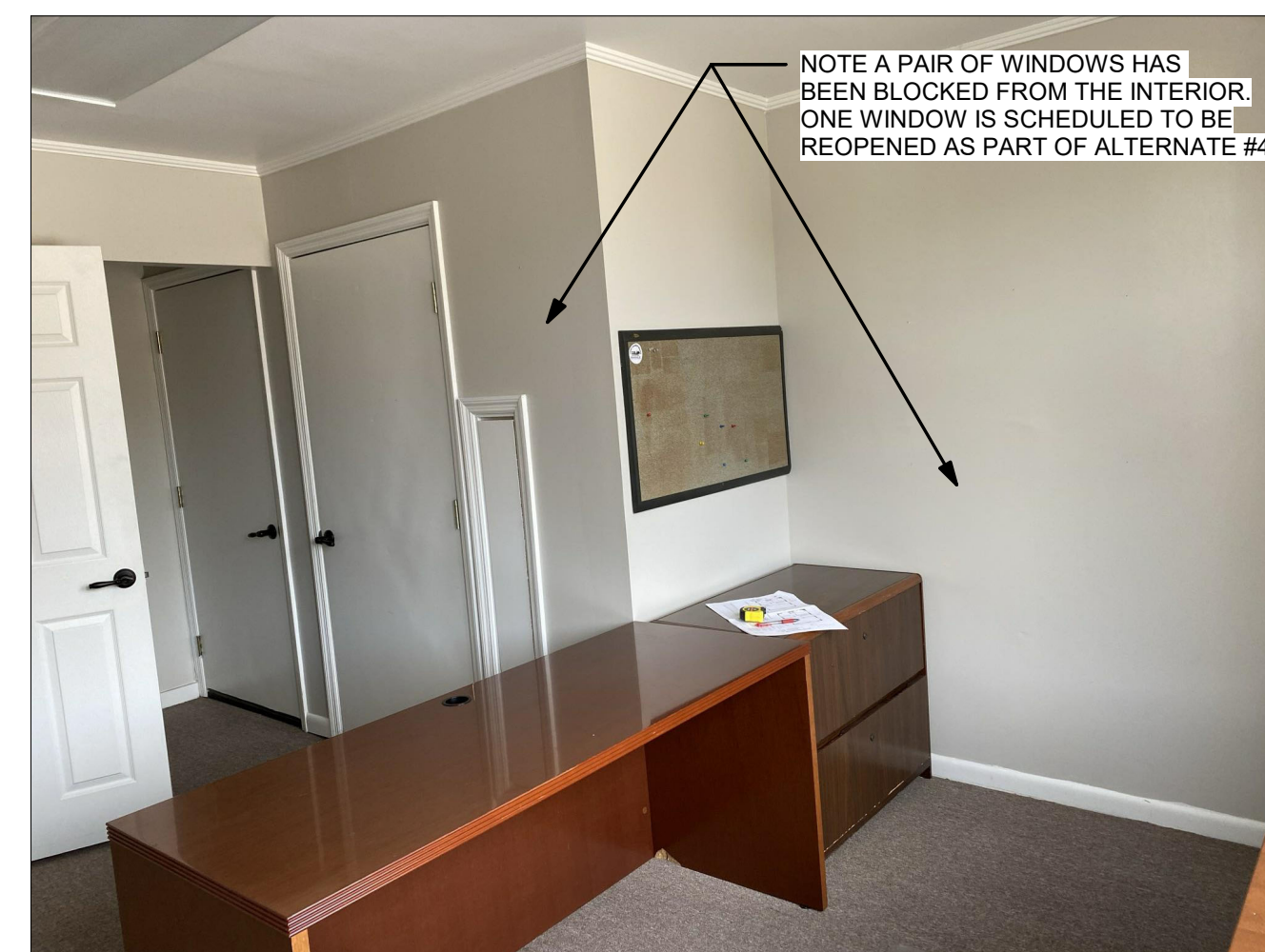
EXISTING CONDITIONS- OFFICE ROOM 104
