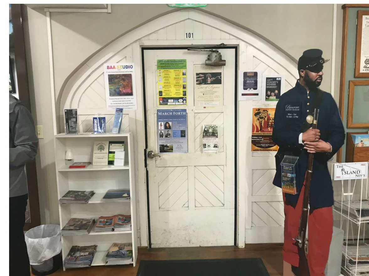
EXISTING CONDITIONS- ACCESS DOOR 2 INTERIOR NOT TO SCALE
