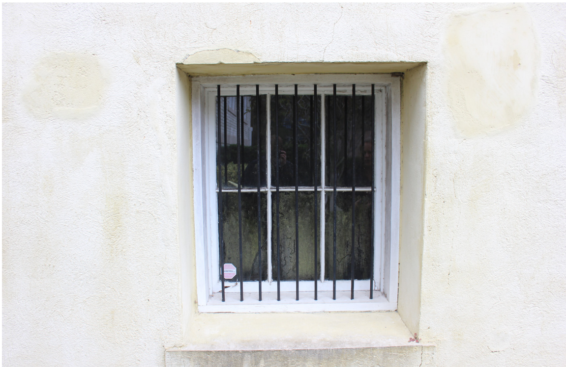
Figure 82: Overview of window #W-19. This is an historic casement window.
