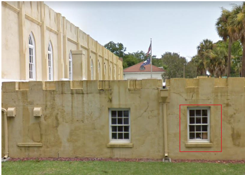
Figure 161: Overview of window #W-36. This is an historic double-hung sash window.
