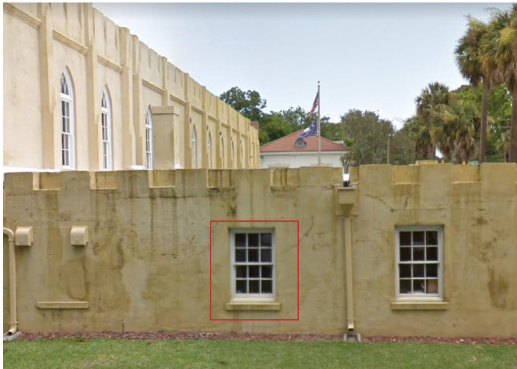
Figure 157: Overview of window #W-36. This is an historic double-hung sash window.
