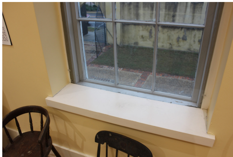
Figure 25: Detail of interior conditions.
