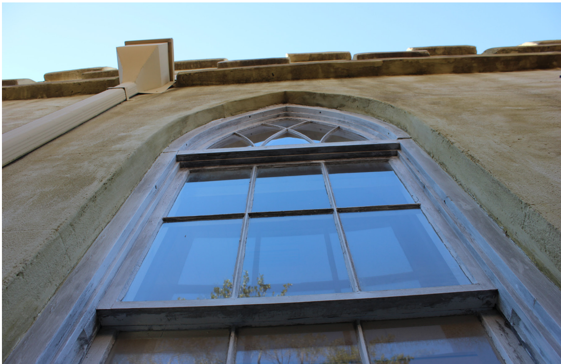
Figure 110: Overview of window #W-26. This is an historic double-hung sash window.
