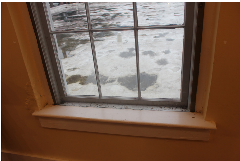
Figure 49: Detail of interior conditions.
