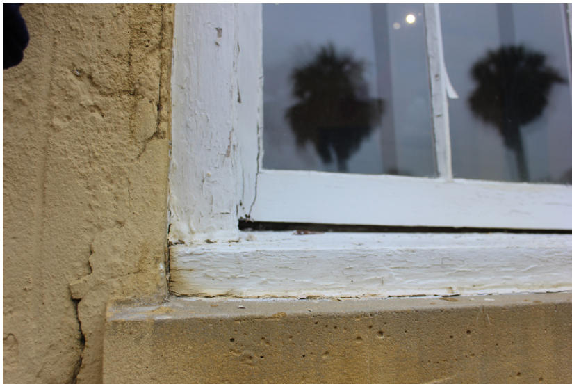
Figure 20: The left side of the window has been repaired with a composite material. The casing may be damaged beneath this repair.
