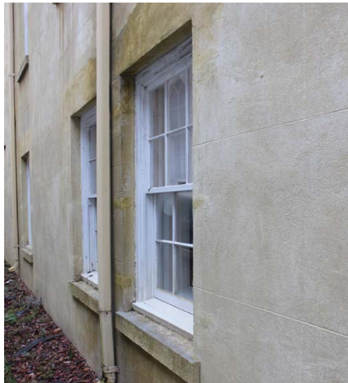
Figure 137: Overview of window #W-33. This is an historic double-hung sash window.
