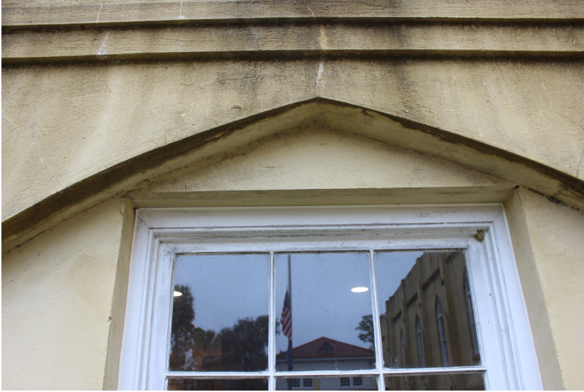
Figure 59: The window is in fair condition.
