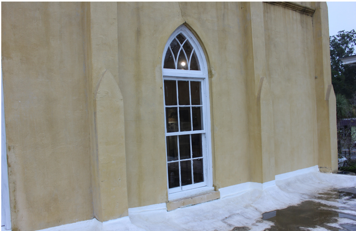
Figure 50: Overview of window #W-11. This is an historic double-hung sash window.
