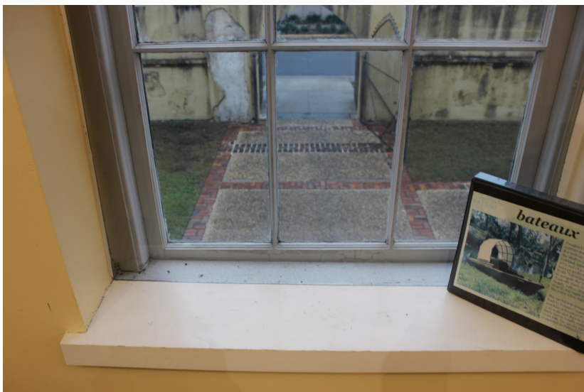
Figure 33: Detail of interior conditions.
