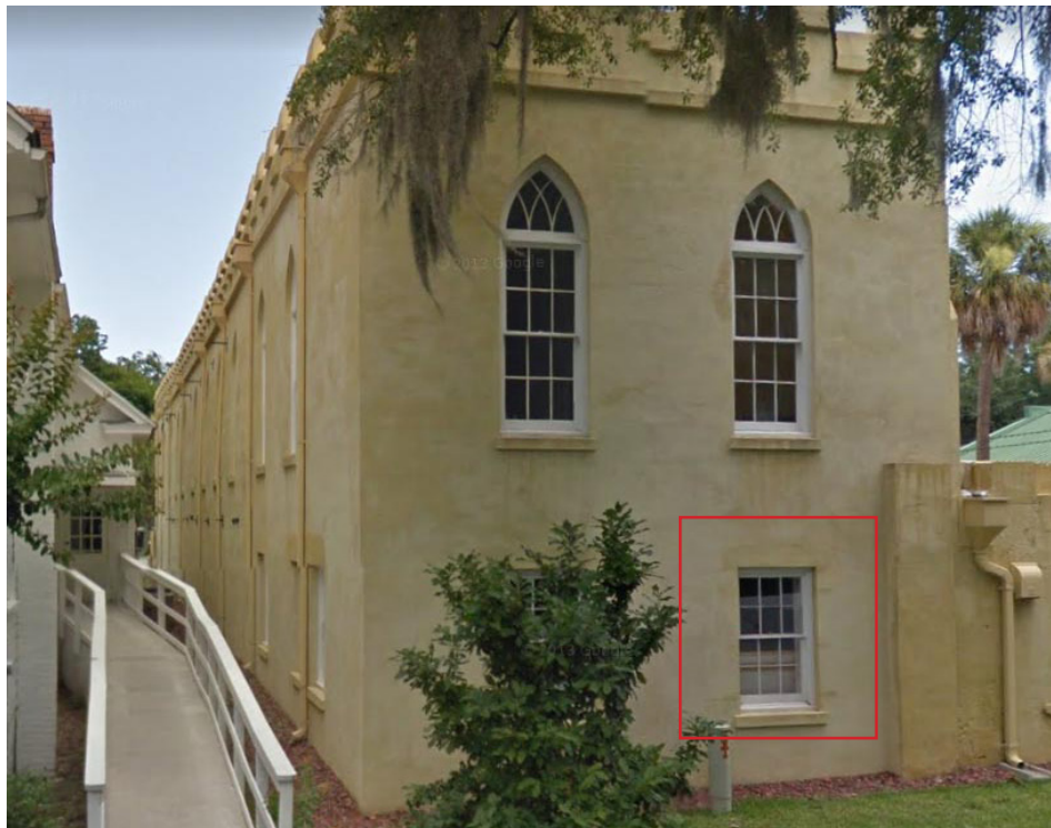
Figure 153: Overview of window #W-36. This is an historic double-hung sash window.
