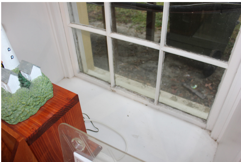
Figure 81: Detail of interior conditions.
