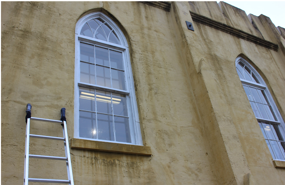
Figure 22: Overview of window #W-04. This is an historic double-hung sash window.
