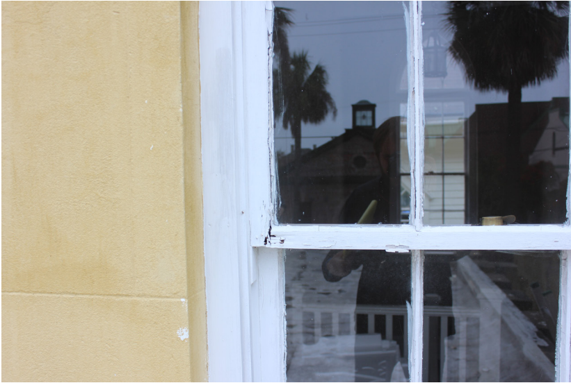
Figure 16: The upper sash is deteriorated at intersection of the left stile and bottom rail.
