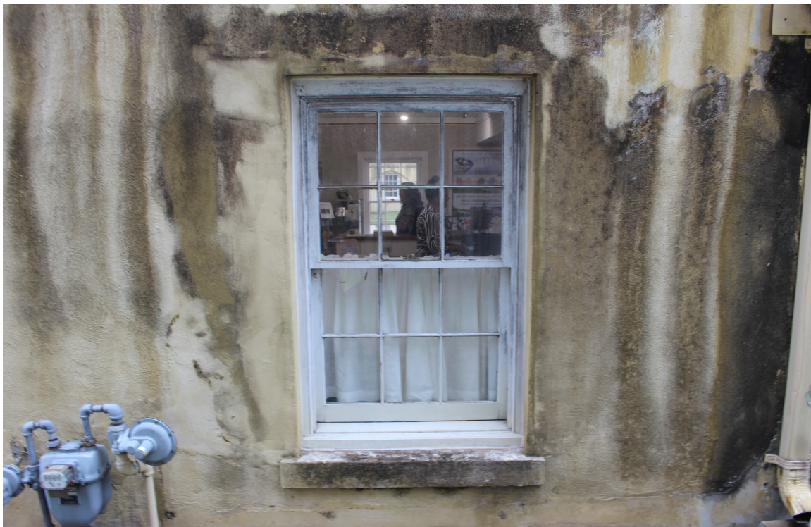
Figure 70: Overview of window #W-16. This is an historic double-hung sash window.
