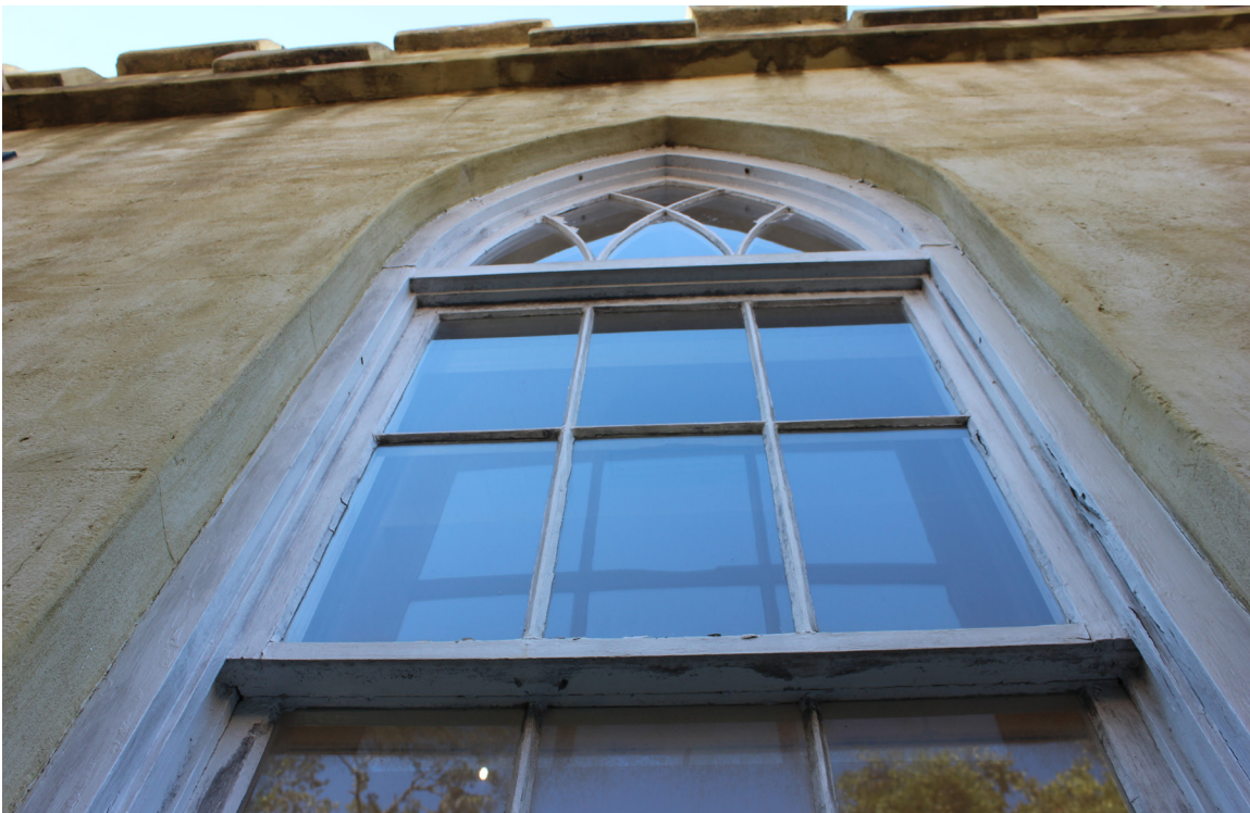
Figure 118: Overview of window #W-28. This is an historic double-hung sash window.
