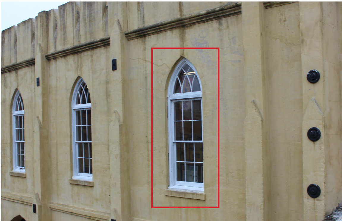
Figure 38: Overview of window #W-08. This is an historic double-hung sash window.
