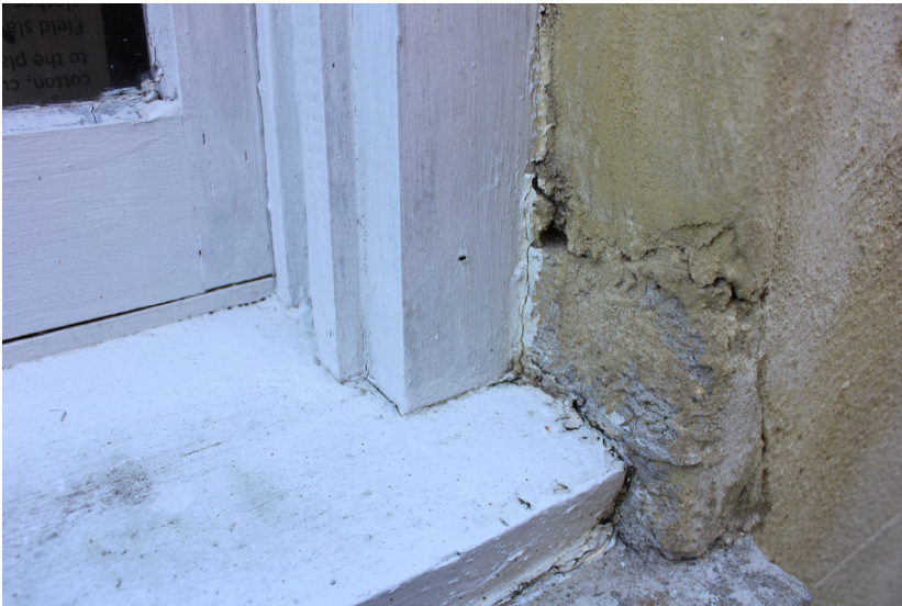
Figure 116: Detail of stucco repair.
