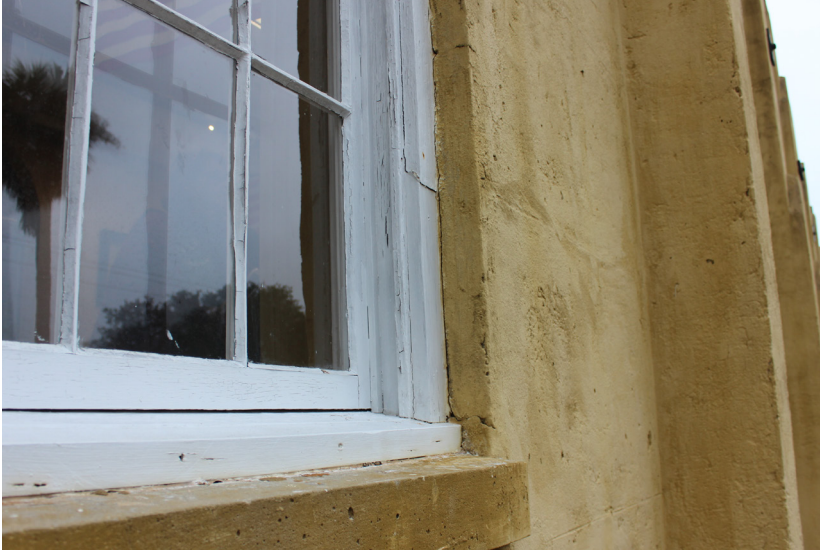
Figure 23: The casing on the lower right hand side has been repaired with a dutchman. The dutchman is now releasing from the casing.
