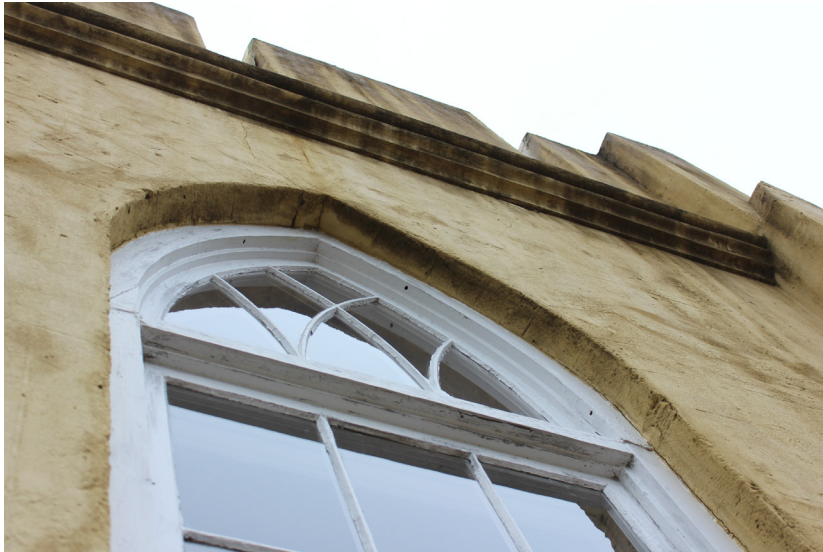
Figure 19: The transom appears to be historic and is in fair condition.
