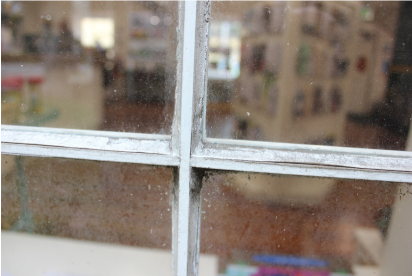
Figure 76: The woodwork is in fair condition.
