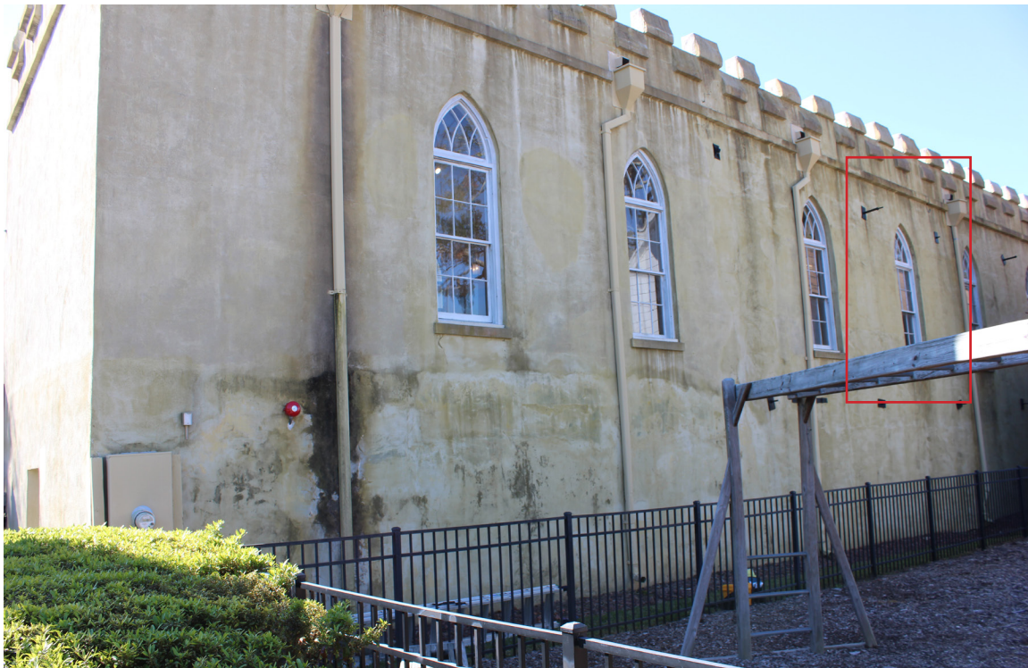
Figure 98: Overview of window #W-23. This is an historic double-hung sash window.
