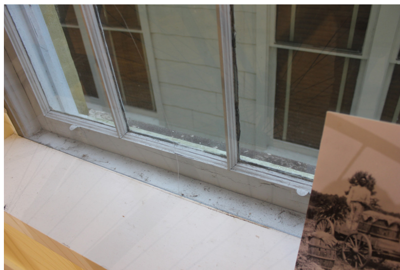
Figure 109: Detail of interior conditions.
