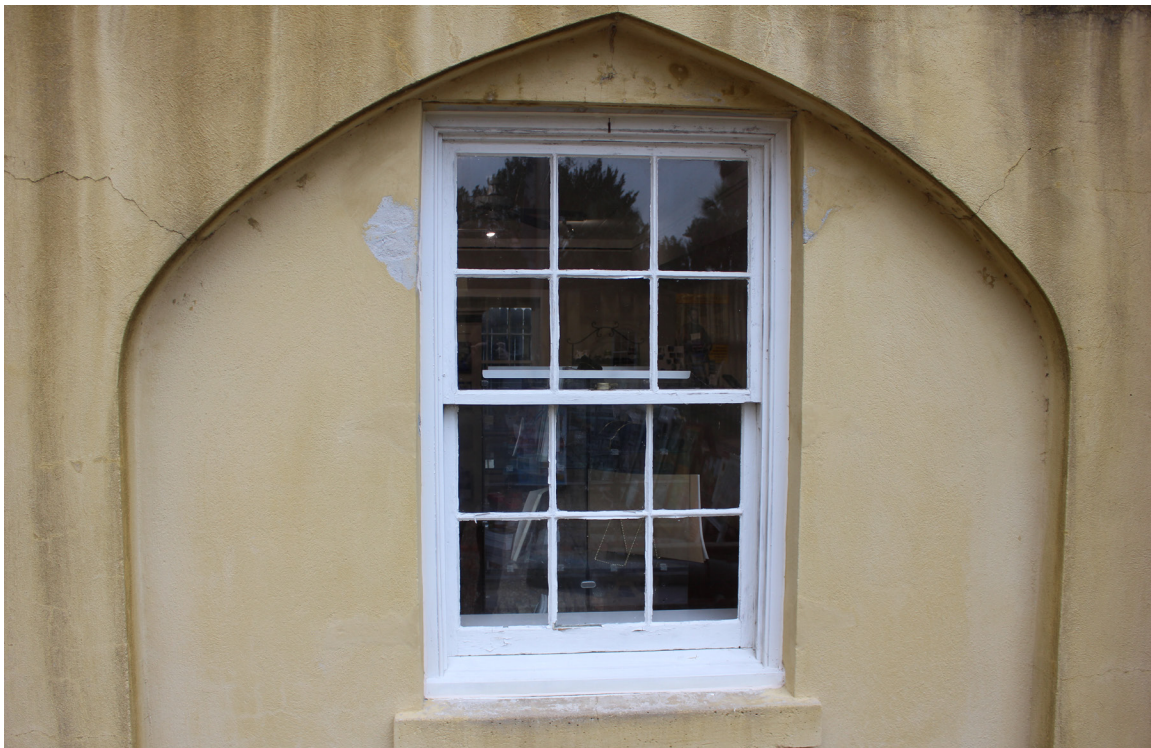
Figure 66: Overview of window #W-15. This is an historic double-hung sash window.
