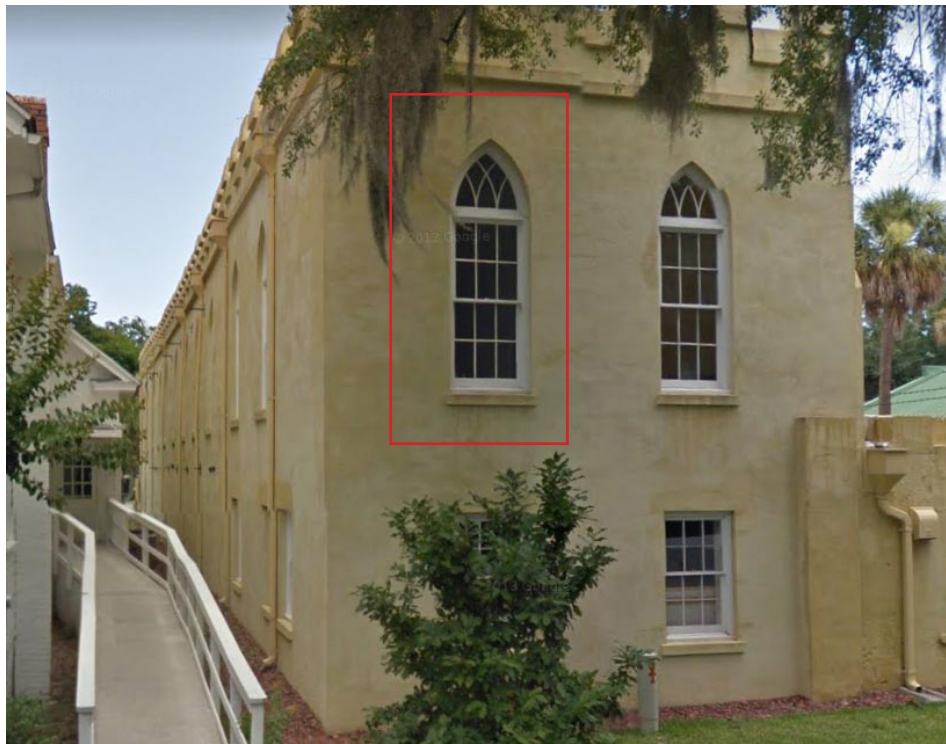
Figure 141: Overview of window #W-34. This is an historic double-hung sash window.
