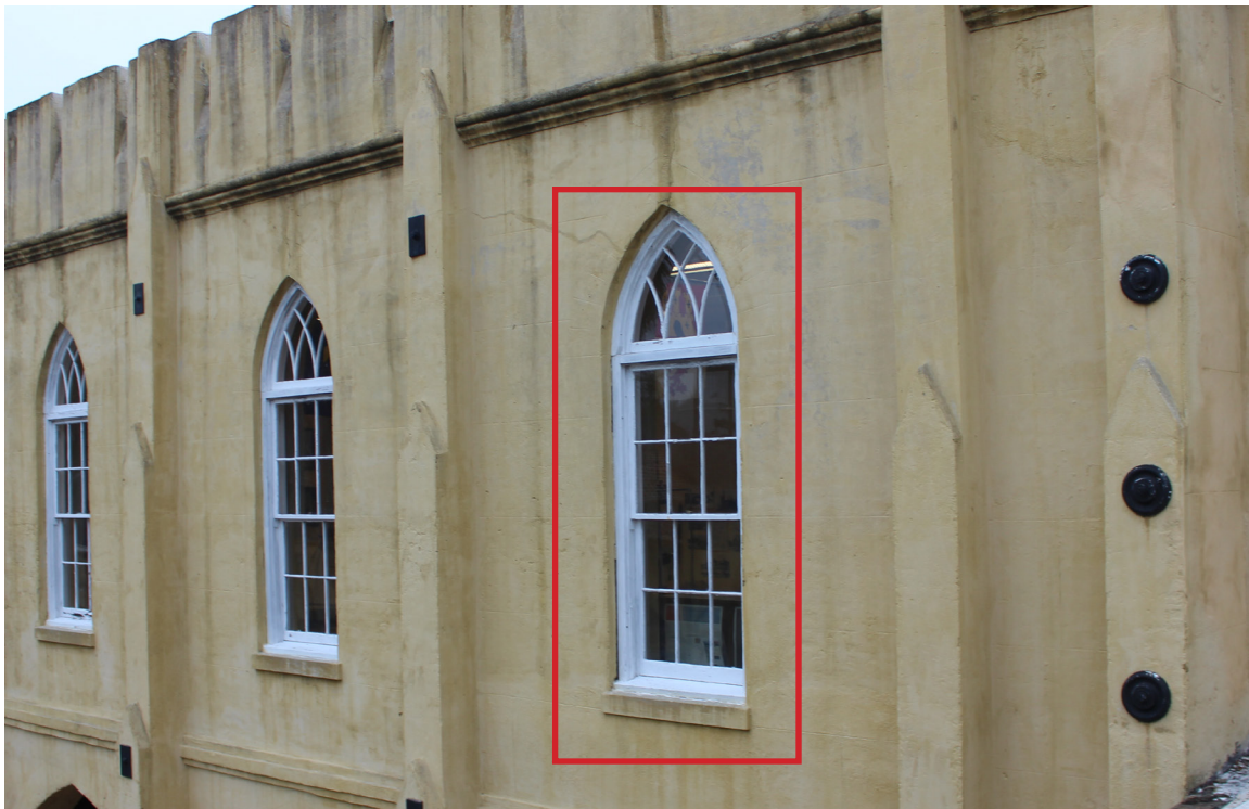
Figure 42: Overview of window #W-09. This is an historic double-hung sash window.
