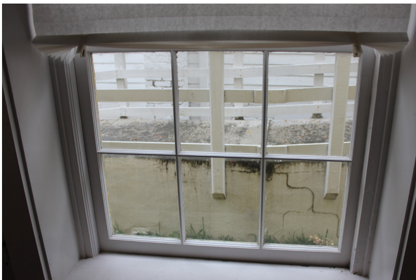
Figure 136: Detail of interior conditions.
