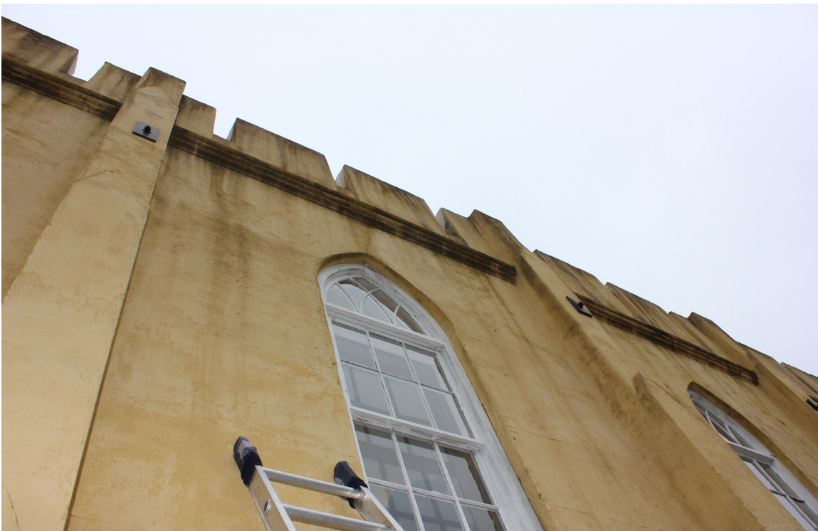
Figure 30: Overview of window #W-06. This is an historic double-hung sash window.
