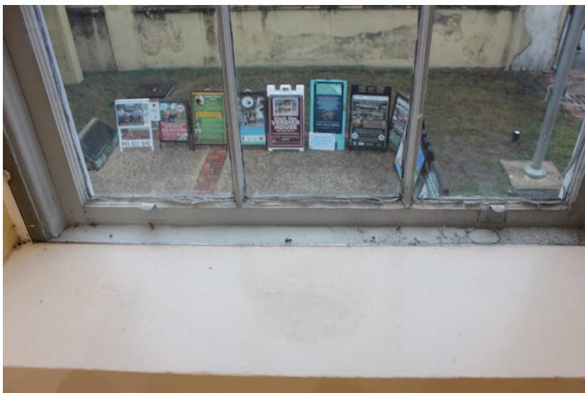
Figure 41: Detail of interior conditions.
