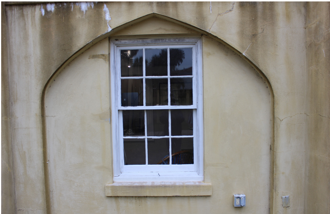
Figure 54: Overview of window #W-12. This is an historic double-hung sash window.
