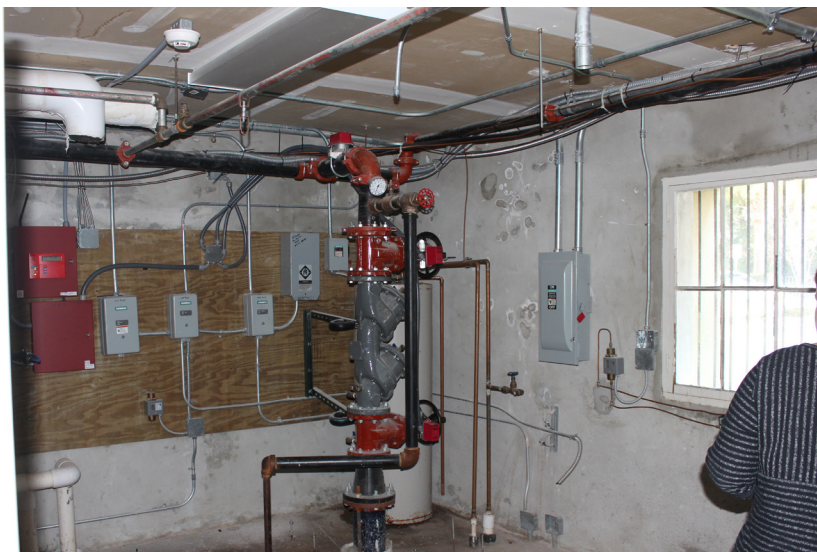
Figure 85: Detail of interior conditions.
