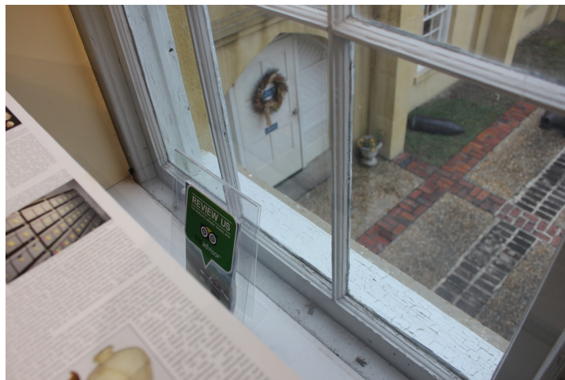
Figure 45: Detail of interior conditions.
