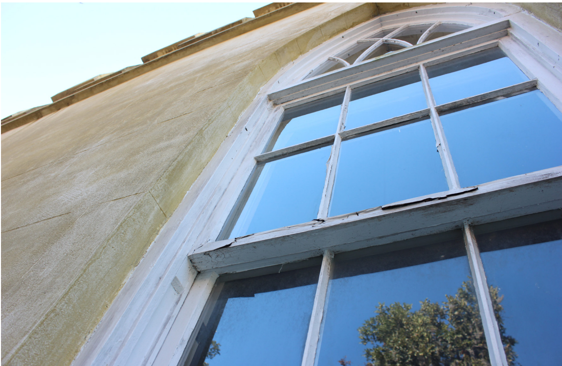
Figure 126: Overview of window #W-30. This is an historic double-hung sash window.
