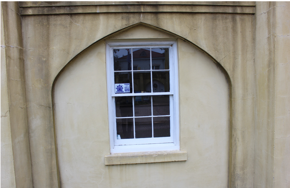
Figure 58: Overview of window #W-13. This is an historic double-hung sash window.
