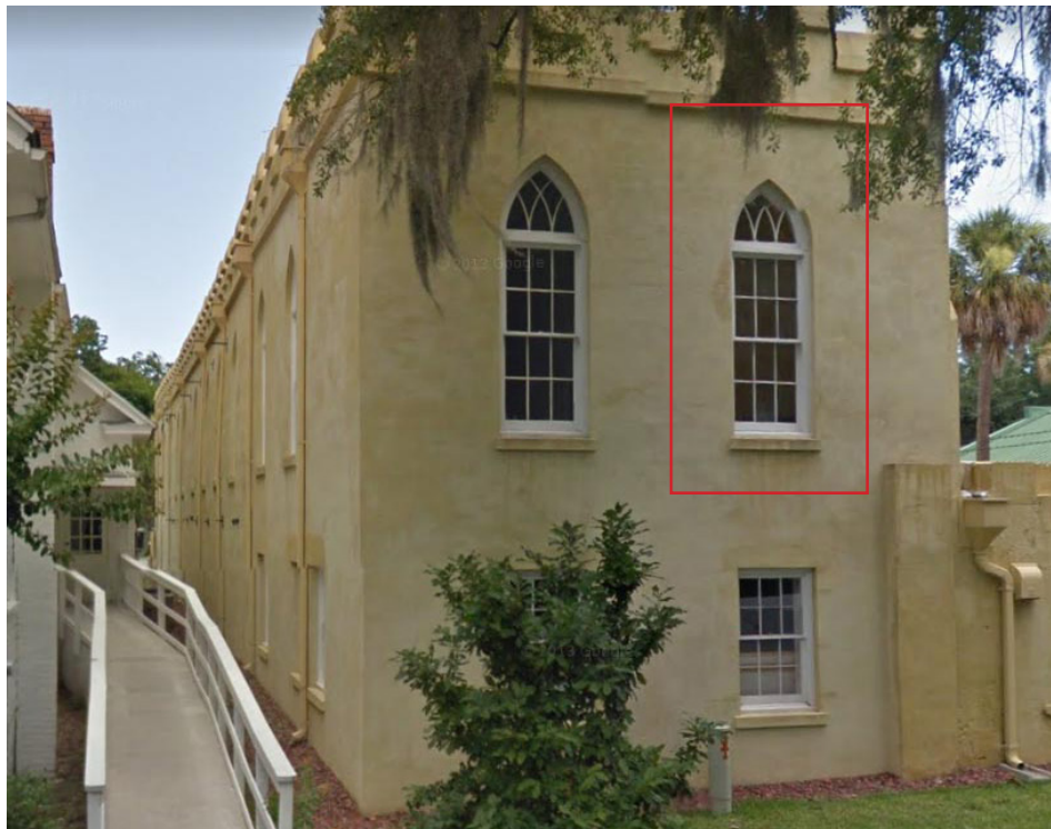
Figure 145: Overview of window #W-35. This is an historic double-hung sash window.
