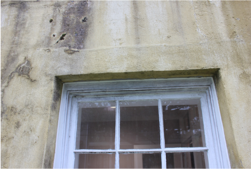
Figure 159: The wooden elements are in good condition.
