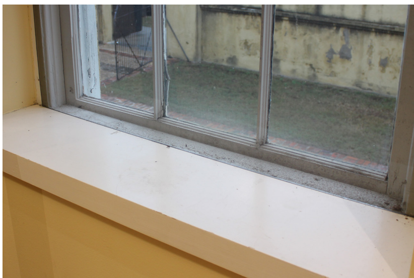
Figure 21: Detail of interior conditions.
