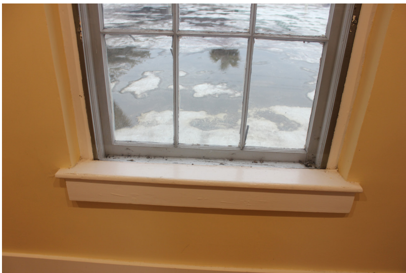
Figure 53: Detail of interior conditions.
