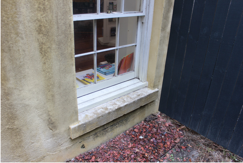
Figure 75: The woodwork is in fair condition.
