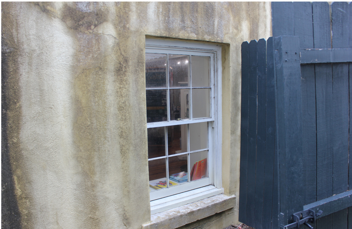
Figure 74: Overview of window #W-17. This is an historic double-hung sash window.
