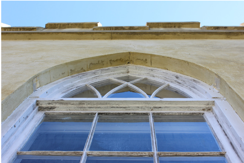
Figure 146: Biogrowth is present on all wooden elements.
