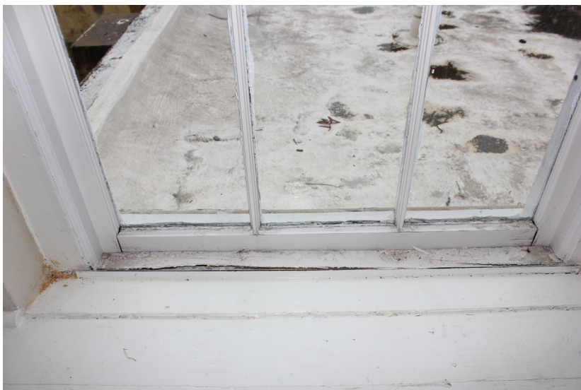
Figure 17: Detail of interior conditions.
