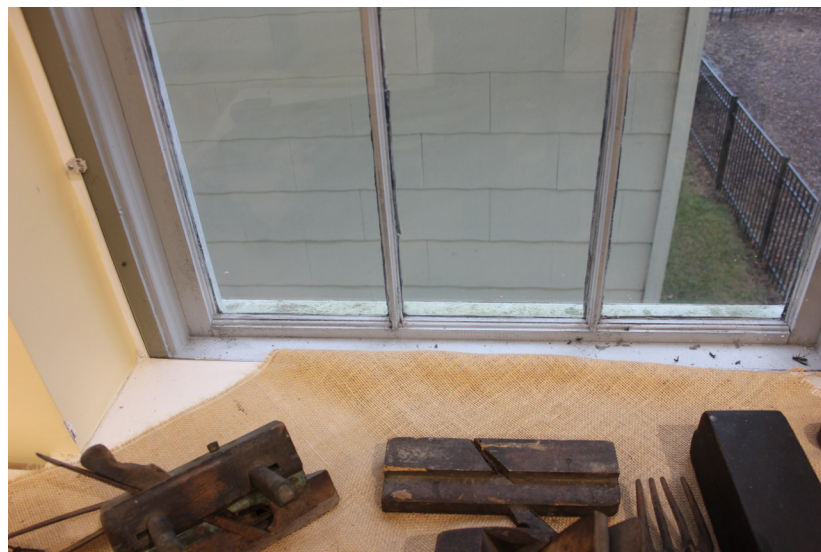
Figure 105: Detail of interior conditions.
