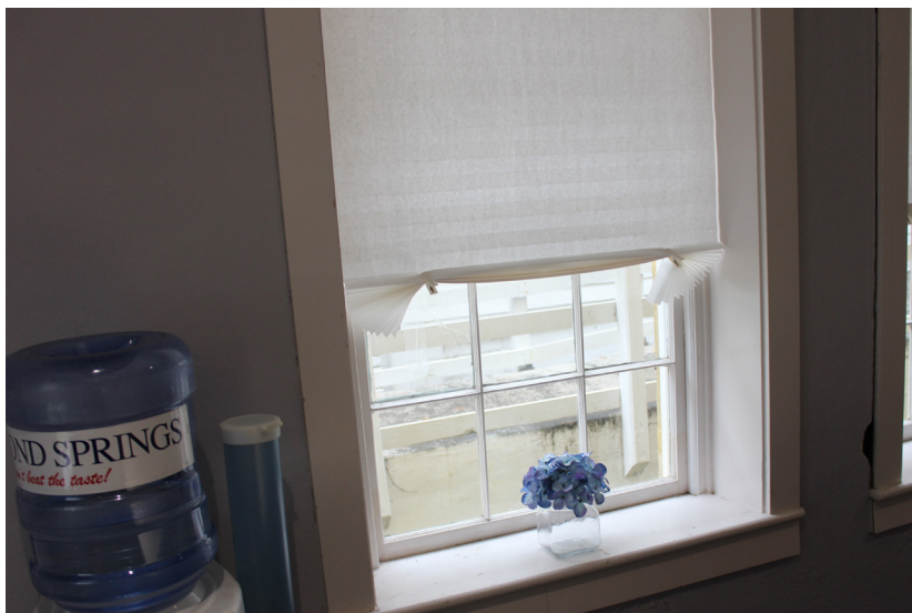
Figure 140: Detail of interior conditions.
