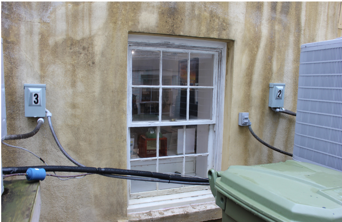
Figure 78: Overview of window #W-18. This is an historic double-hung sash window.
