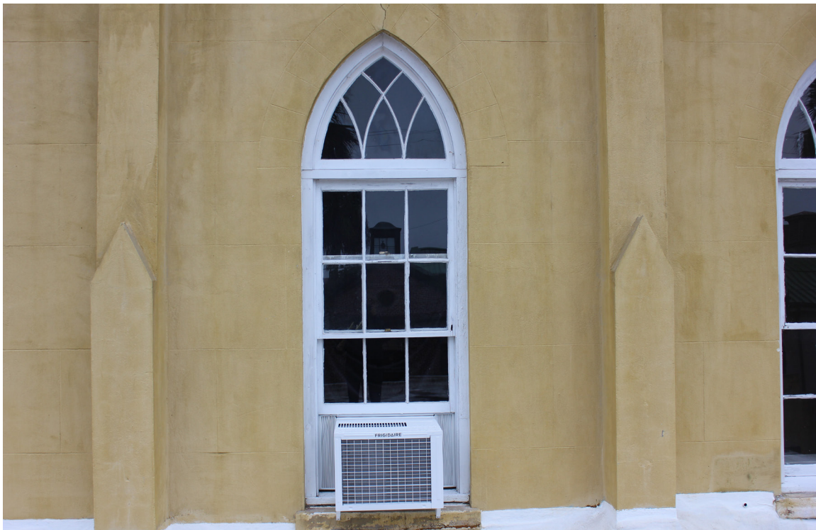
Figure 10: Overview of window #W-01. This is an historic double-hung sash window.
