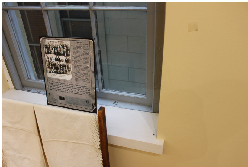
Figure 113: Detail of interior conditions.
