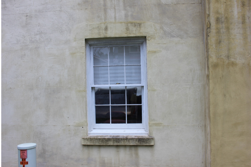
Figure 154: Detail of broken glass.
