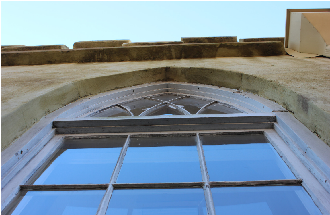
Figure 114: Overview of window #W-27. This is an historic double-hung sash window.
