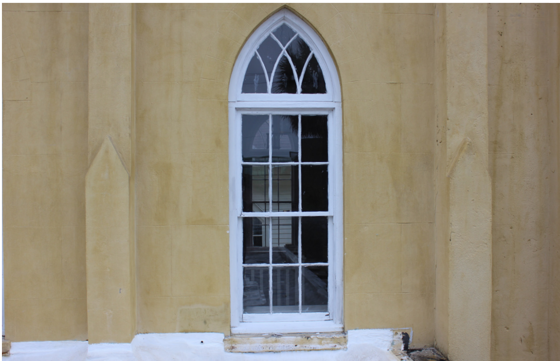
Figure 14: Overview of window #W-02. This is an historic double-hung sash window.
