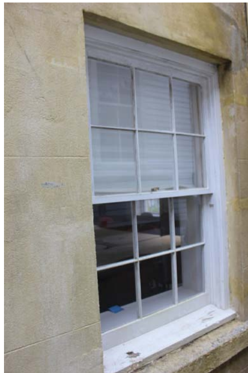
Figure 133: Overview of window #W-32. This is an historic double-hung sash window.
