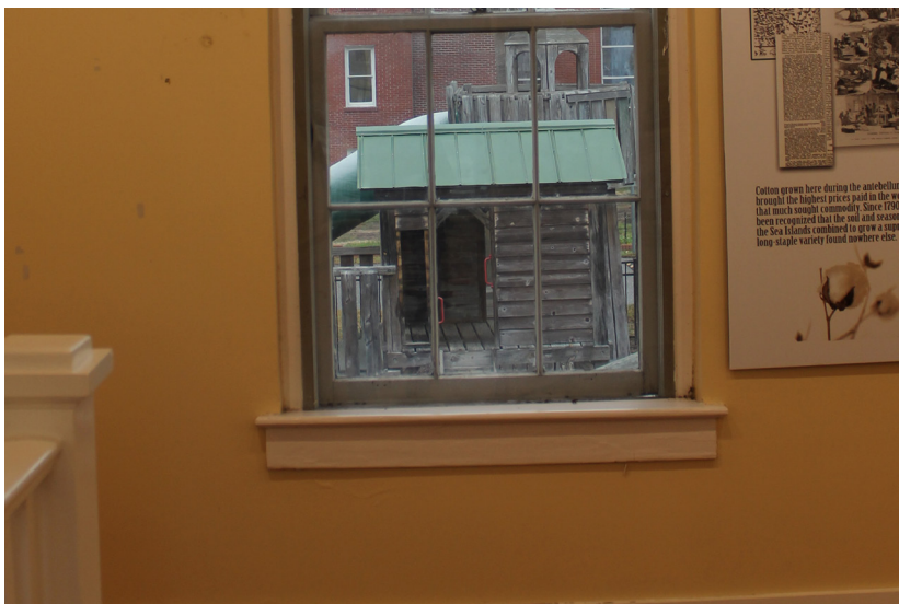
Figure 89: Detail of interior conditions.
