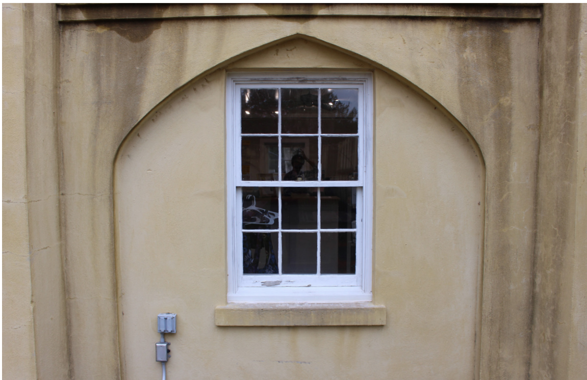
Figure 62: Overview of window #W-14. This is an historic double-hung sash window.
