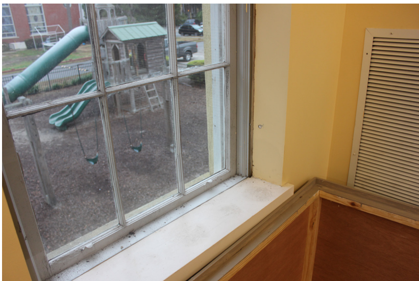
Figure 97: Detail of interior conditions.
