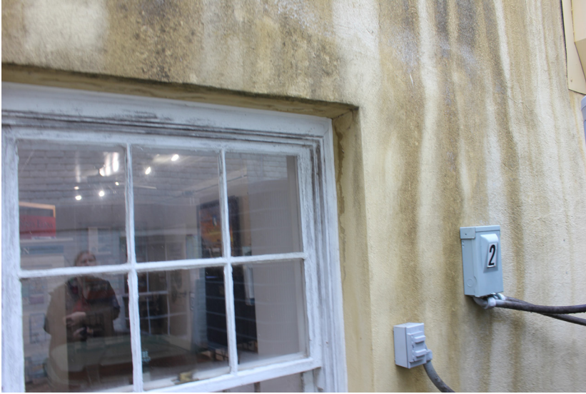
Figure 79: The woodwork is weathered but appears to be sound.
