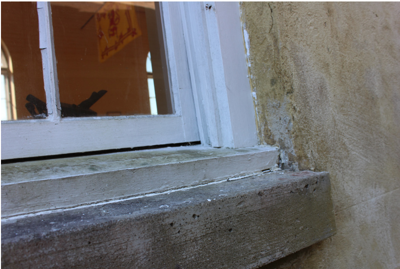
Figure 104: A gap is present between the lower sash and the sill. Biogrowth is present on the sill.
