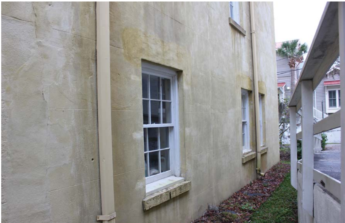
Figure 130: Overview of window #W-31. This is an historic double-hung sash window.
