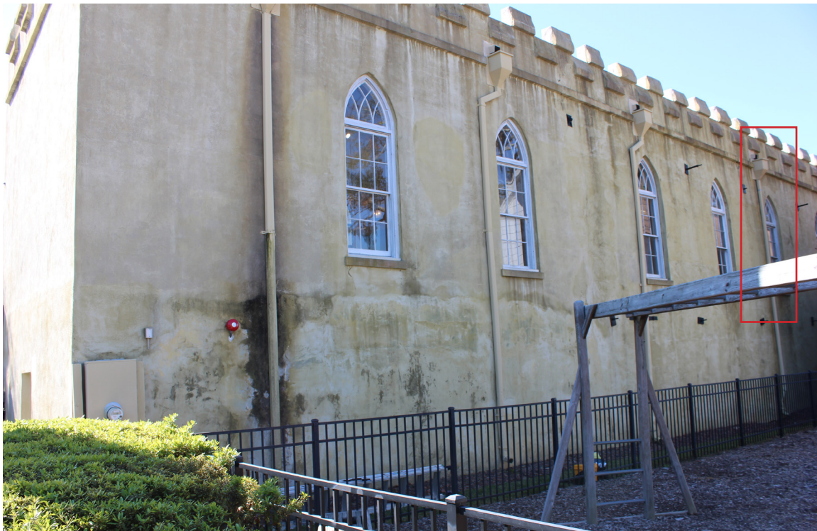
Figure 102: Overview of window #W-24. This is an historic double-hung sash window.
