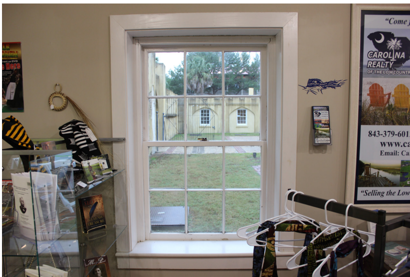
Figure 69: Detail of interior conditions.
