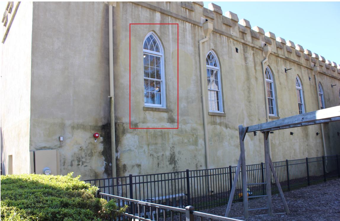
Figure 86: Overview of window #W-20. This is an historic double-hung sash window.
