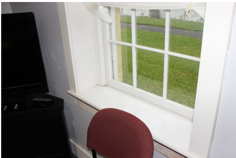
Figure 156: Detail of interior conditions.
