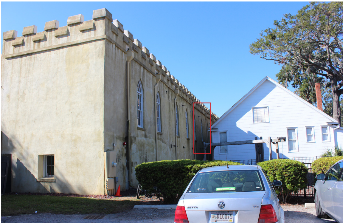
Figure 106: Overview of window #W-25. This is an historic double-hung sash window.
