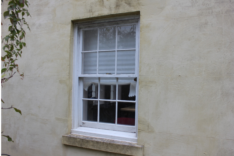
Figure 150: The window is in good condition.
