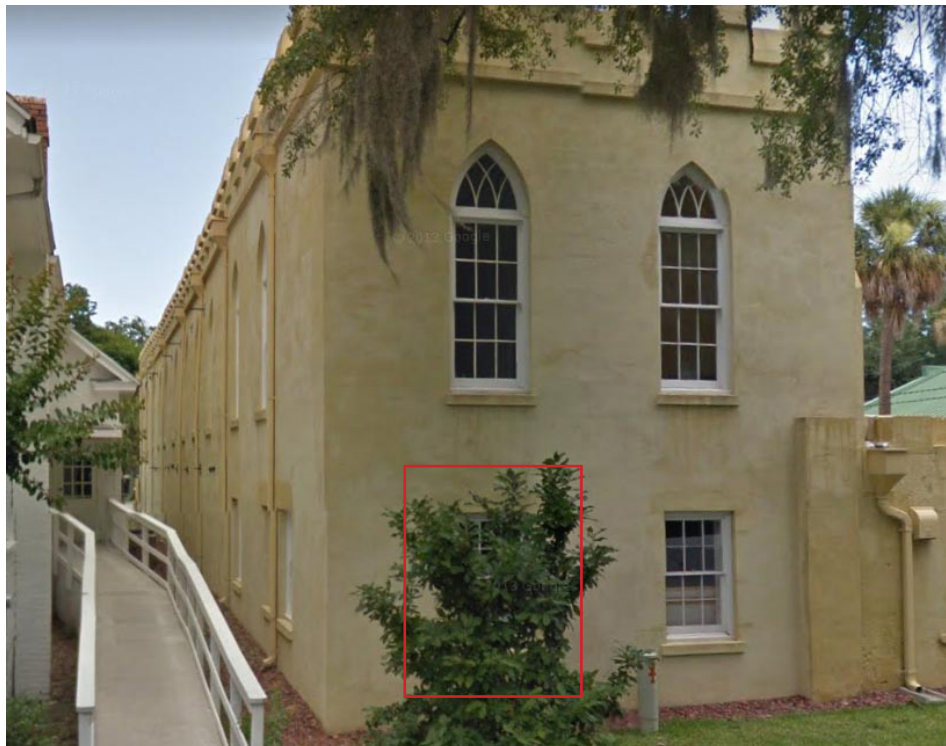
Figure 149: Overview of window #W-36. This is an historic double-hung sash window.
