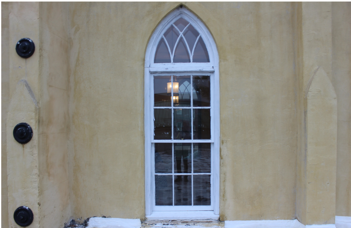
Figure 46: Overview of window #W-10. This is an historic double-hung sash window.
