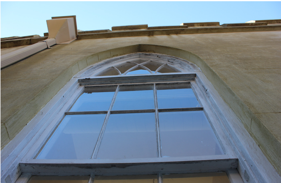
Figure 122: Overview of window #W-29. This is an historic double-hung sash window.
