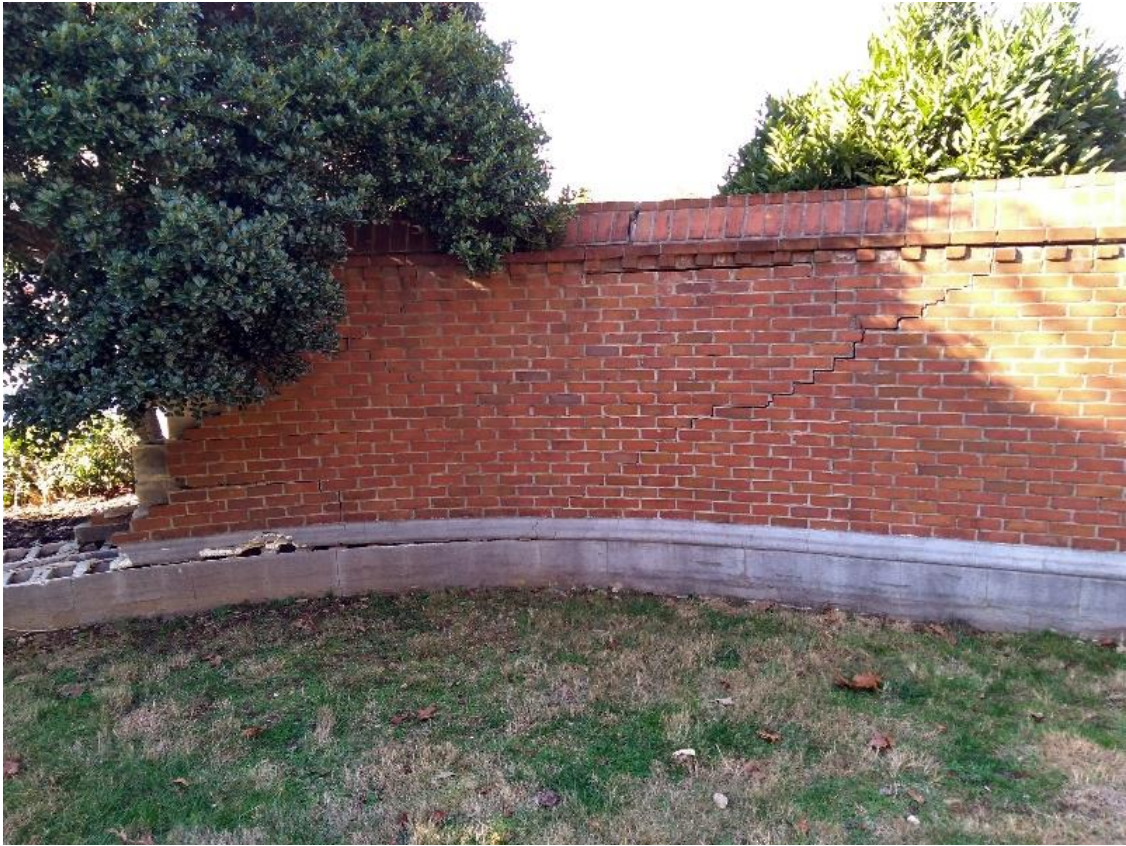
Melton Lake Drive Back Side of Wall
