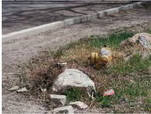
Photograph 1: Example Fire Hydrant Condition
