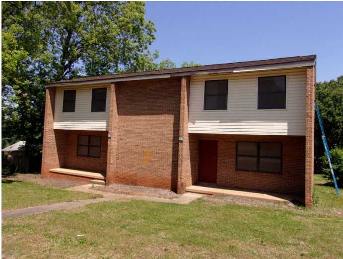
Photo 1 – Typical view of a 2-story duplex.
