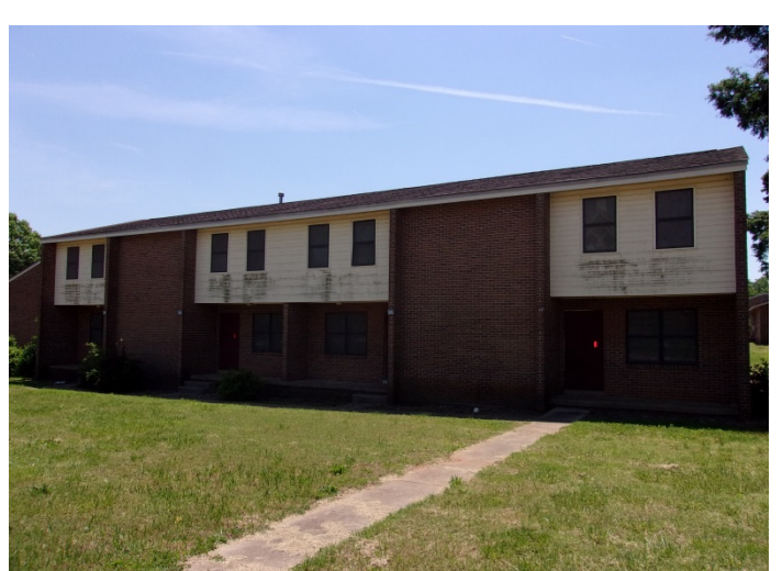
Photo 24 – Typical view of a 2-story, 4-unit building.
