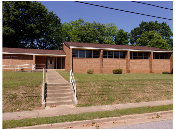
Photo 42 – Administration building No. 30.
