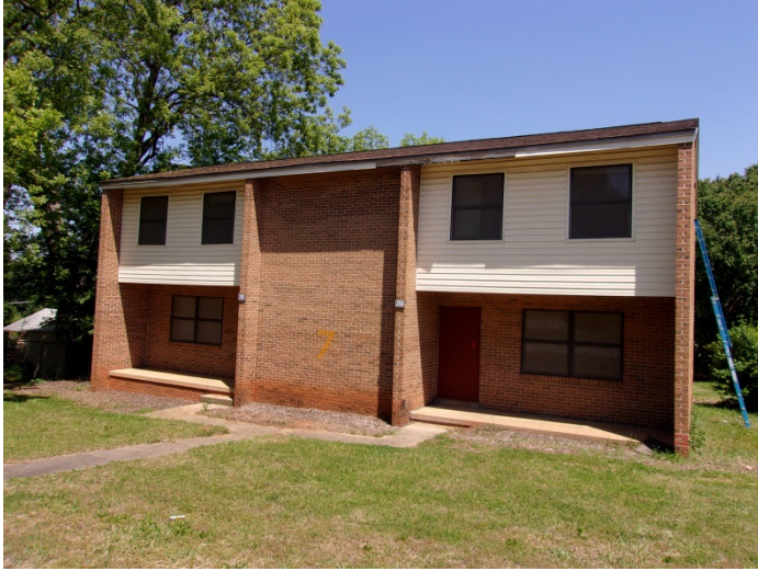
Photo 1 – Typical view of a 2-story duplex.
