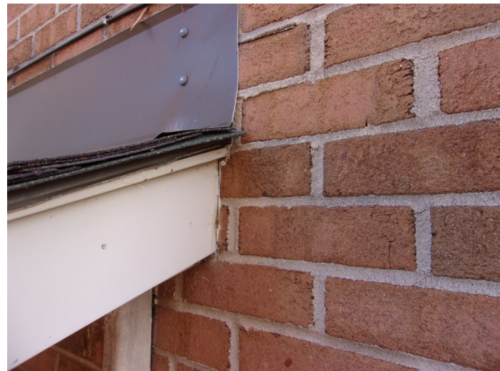
Photo 15 – Typical view of the caulk on the awning & flashing on buildings 1-6 & 36-38.
