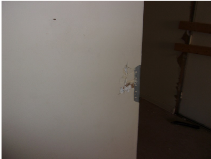
Photo 1 – Typical view of drywall with joint compound and tape throughout buildings 1-6 & 36-38.
