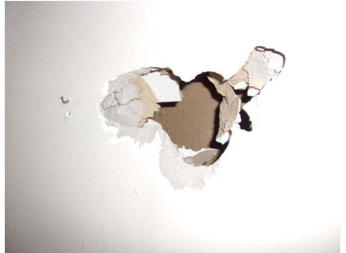
Photo 2 – Typical view of drywall with joint compound and tape throughout buildings 1-6 & 36-38.
