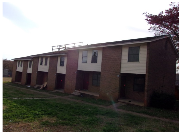
Photo 24 – Typical view of a 2-story; 2 & 3 bedrooms; 1 bathroom; 6-plex apartment building.
