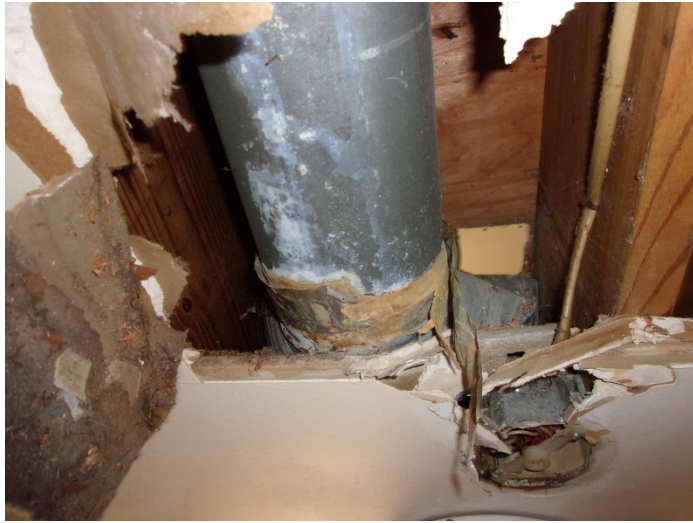
Photo 19 – Typical view of HVAC tape & mastic above the ceilings throughout buildings 1-6 & 36 & 38.
