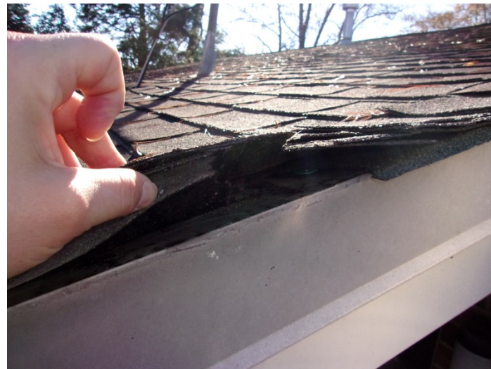
Photo 9 – Typical view of the roof shingles & felt on the main roof and awning roofs on buildings 1-6 & 36-38.
