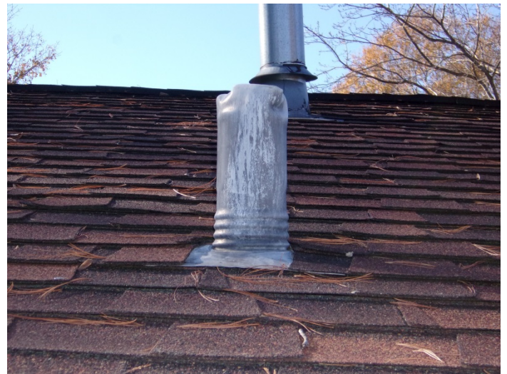
Photo 10 – Typical view of the paint coated roof vents on buildings 1-6 & 36-38.
