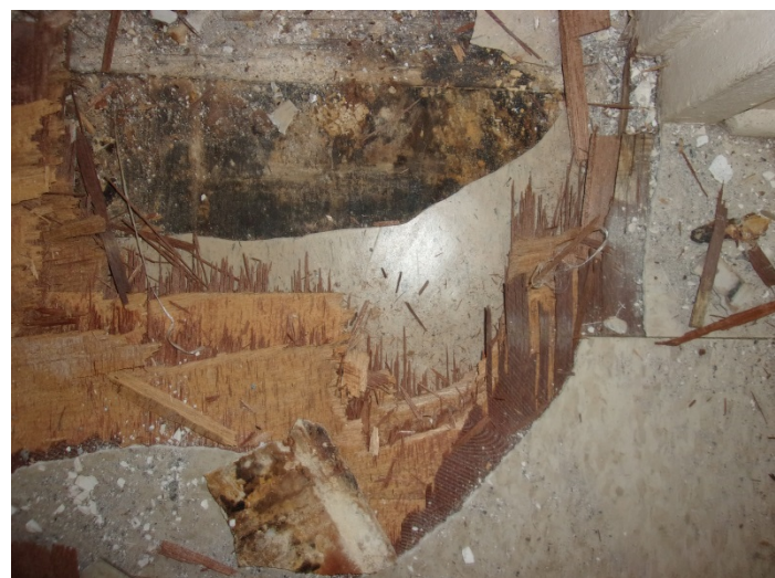
Photo 17 – Typical view of 12" x 12" tan speckled floor tile & mastic over 2 nd layer of floor tile & mastic under wood throughout buildings 1-6 & 36-38.
