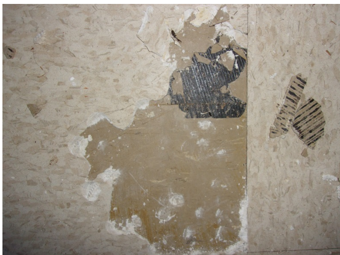
Photo 23 – Typical view of 12"x12" brown streaked floor tile and mastic (bottom layer) assumed positive in Buildings 7 to 35.
