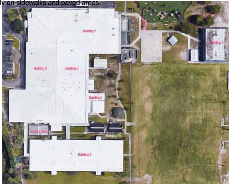
Aerial of JBES Roofs
