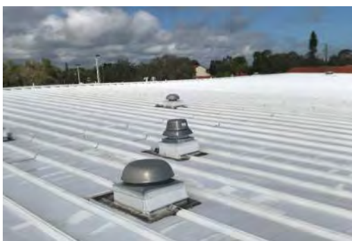
Buildings 2, 3 & 5 Looking Northwest
