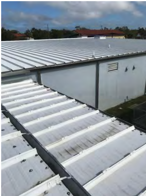
Buildings 2, 3 & 5 Looking Northeast
