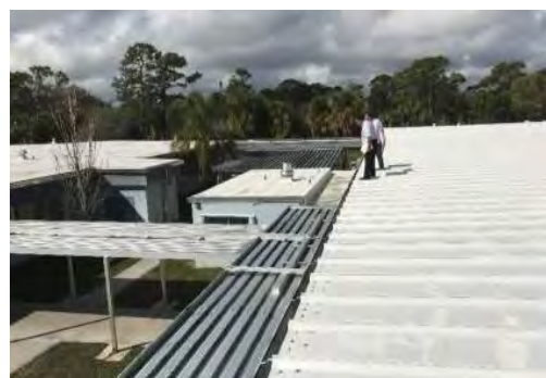
Buildings 2, 3 & 5 Looking West
