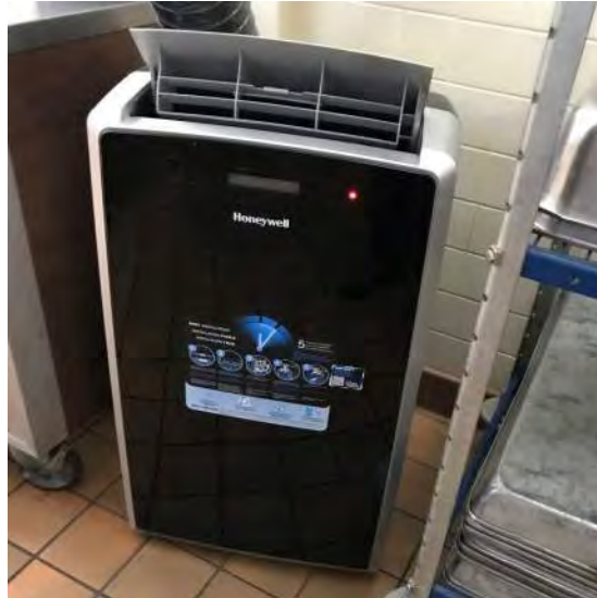
Spot Cooler used in Kitchen
