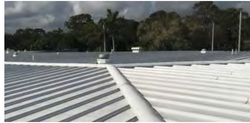
Buildings 2, 3 & 5 Looking West
