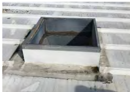
Weather Cover Removed by Irma
