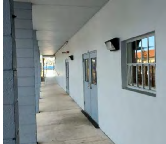
Exterior Lighting Accessible to Vandals
