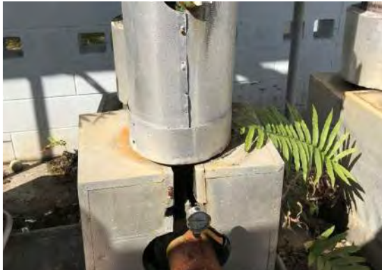
Degraded Insulation
