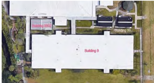
Aerial of JBES Roofs
