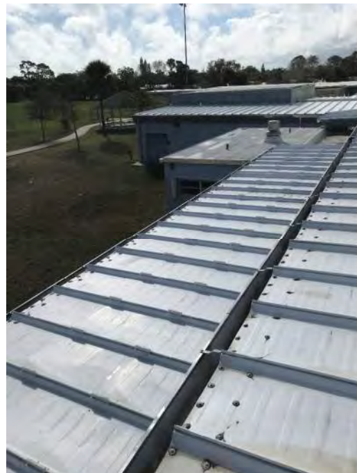
Buildings 2, 3 & 5 Looking Southeast
