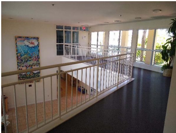
Atrium over Lobby
