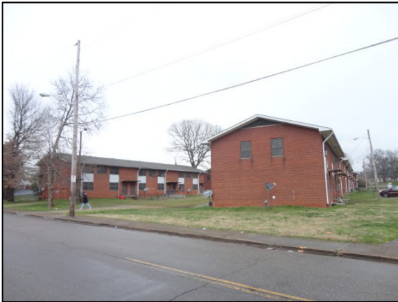
Site facing east from S Bell Street.
