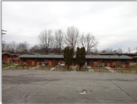
Subject site facing north from Kenner Avenue.
