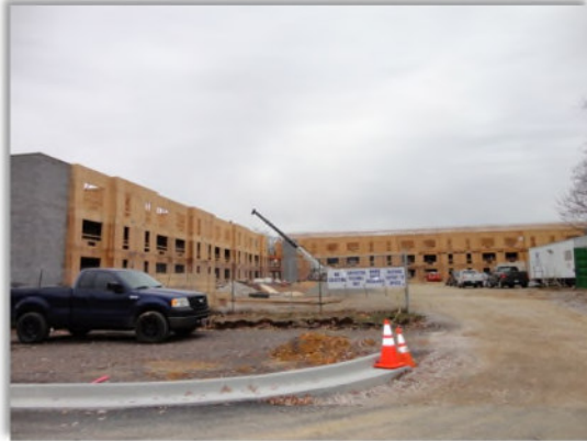
Five Points Phase I under construction to the south.
