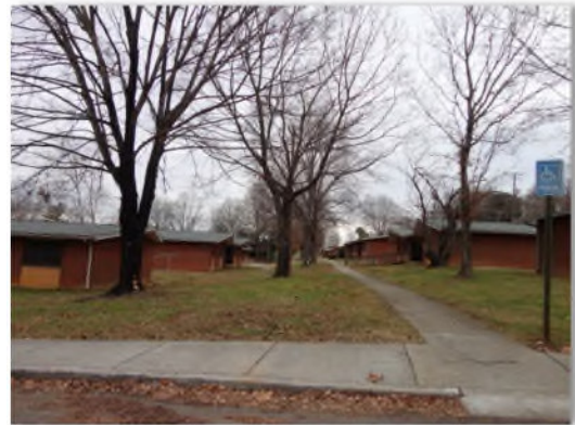
Site facing east from S Kyle Street.
