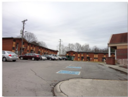
Existing buildings and parking lot.
