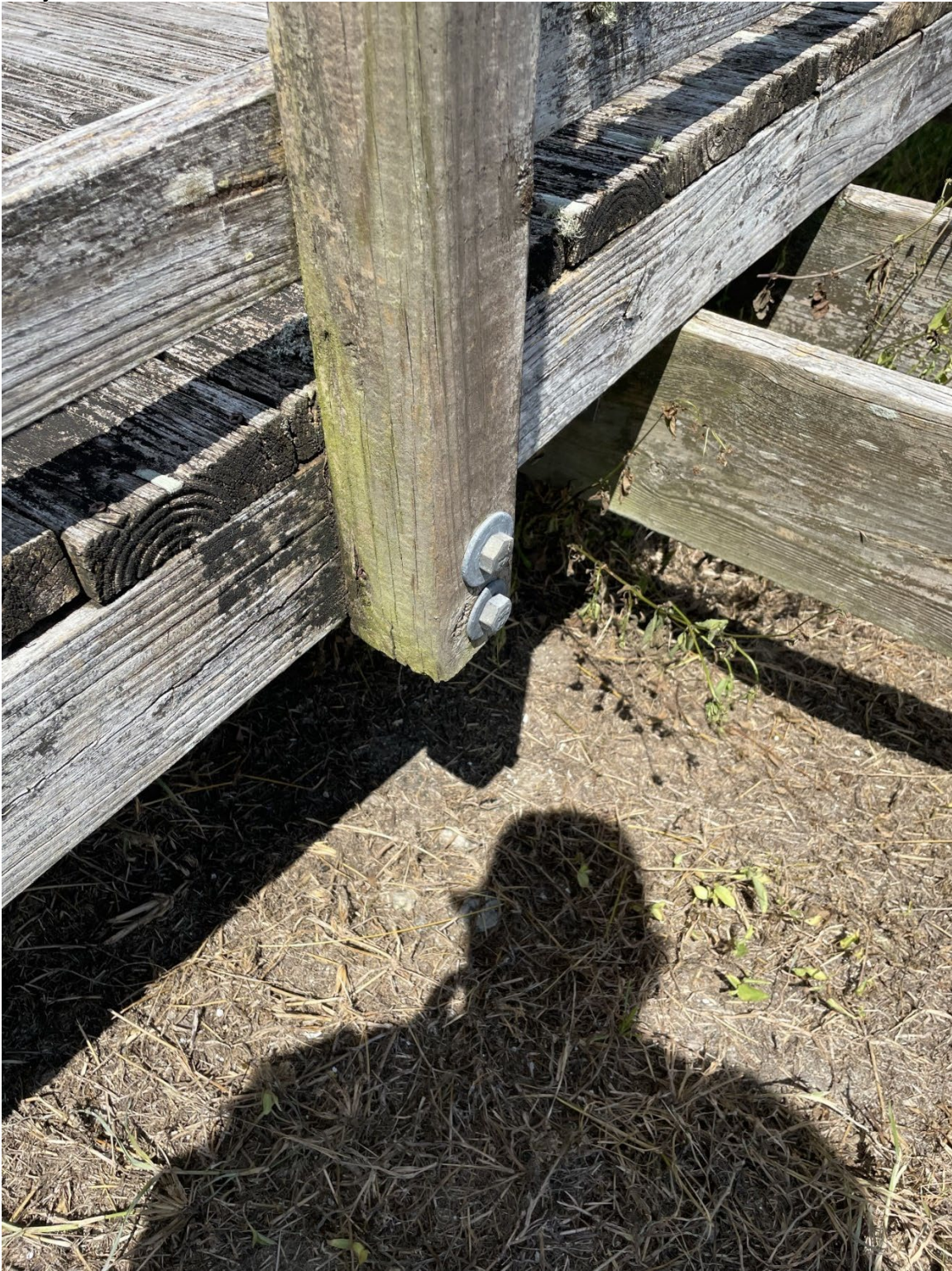
Figure 6: SLWMA – S-262 WALKWAY 4" by 4" Installation
