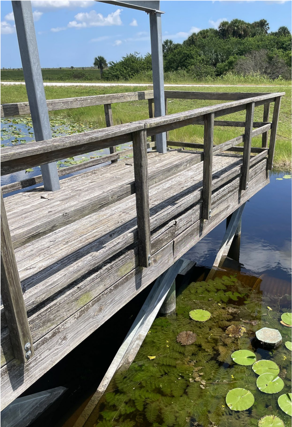
Figure 5: SLWMA – S-262 WALKWAY Platform at end of Walkway (east side)
