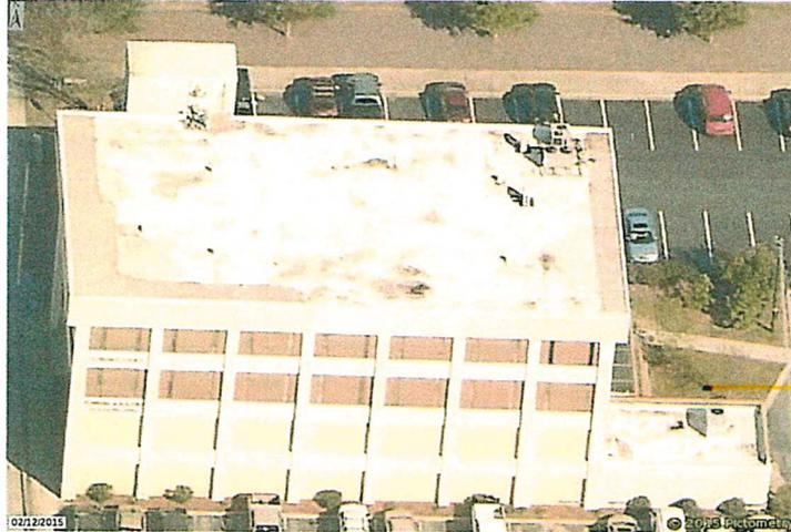
The roof system has 2 roofs. The original roof is a structural concrete deck with a multi ply asphalt roof system. The second roof is a ballasted TPO single ply membrane over a recover board.
