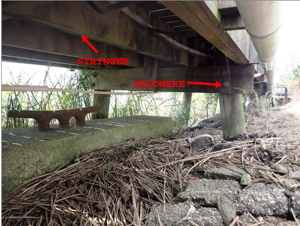
Figure 1.2-2: Typical Bent – Northwestern section, 8 foot wide (Sta. 13+50)
