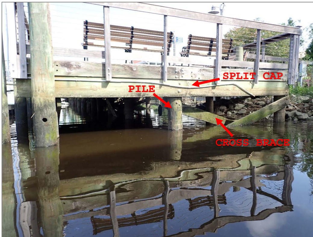
Figure 1.2-1: Typical Bent – Southeastern section, 12 foot wide (Sta. 0+00)
