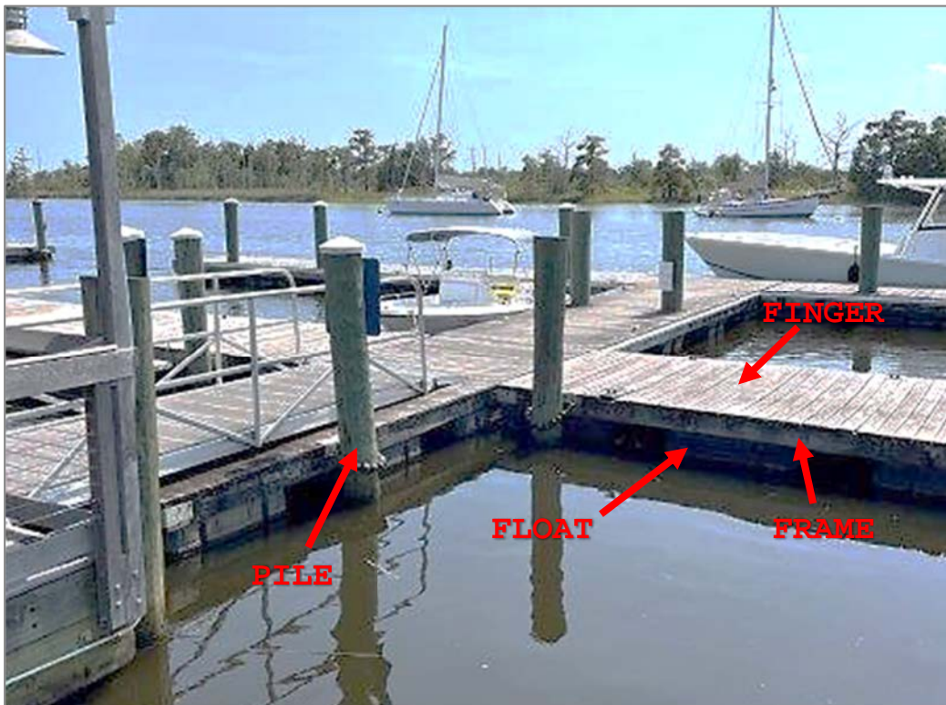
Figure 1.2-3: Typical Floating Dock – East Floating Dock (Sta. 0+00)
