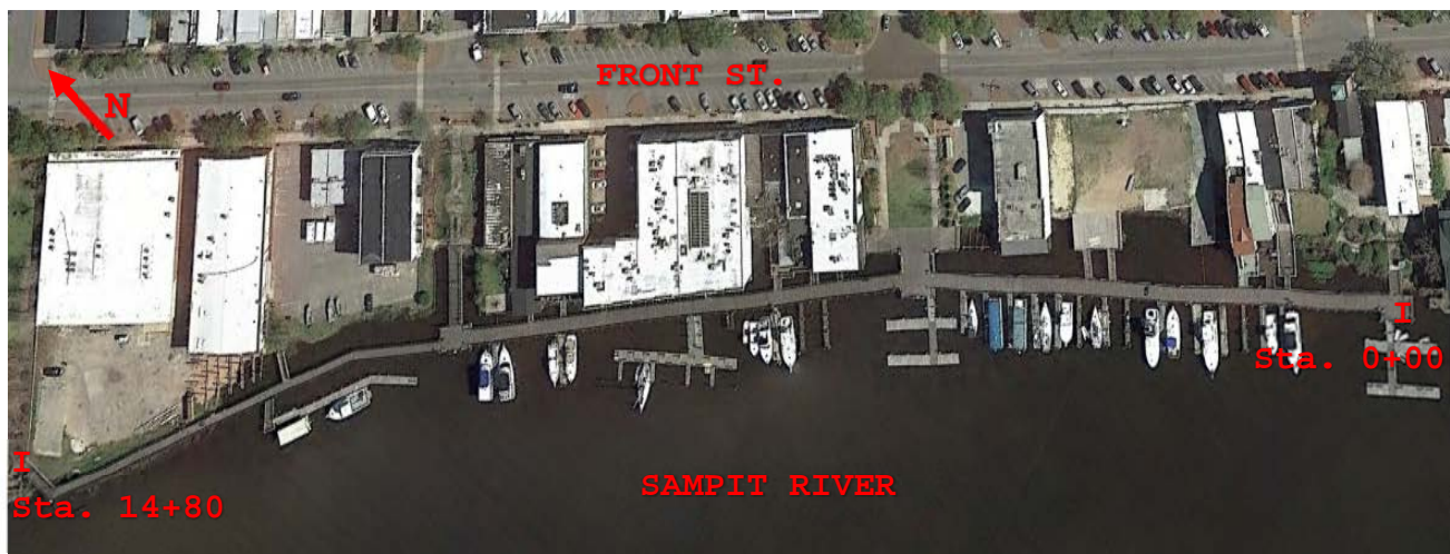
Figure 1.1-1. Aerial View of the Harborwalk from Google Earth 2023 with Annotation from Collins
