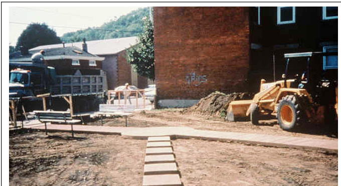
FIGURE 12.22 Replacing resident pathway after soil removal.
