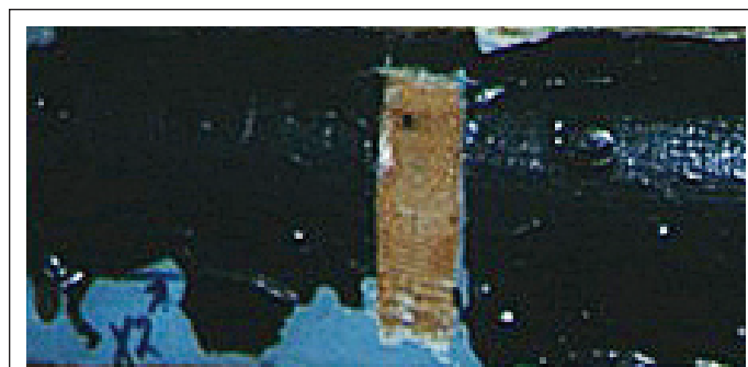
FIGURE 5.17 Damage to painted surface caused by paint chip sampling.
