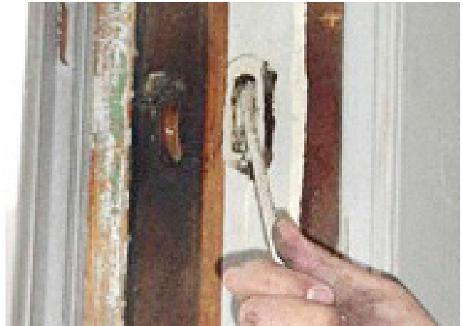
FIGURE 11.8 Remove sash controls/weights.
