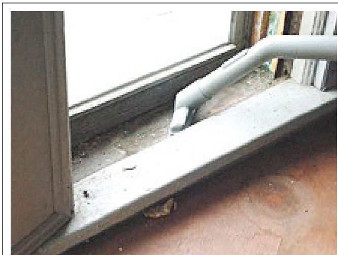
FIGURE 11.5 Prepare the worksite and pre-clean the window.
