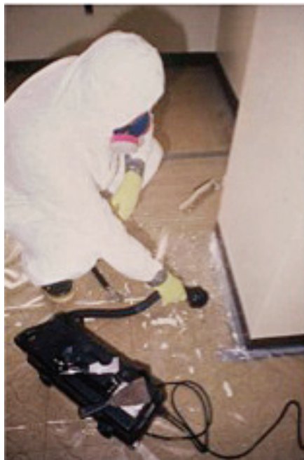
FIGURE 14.8 Vacuuming the floor containment.
