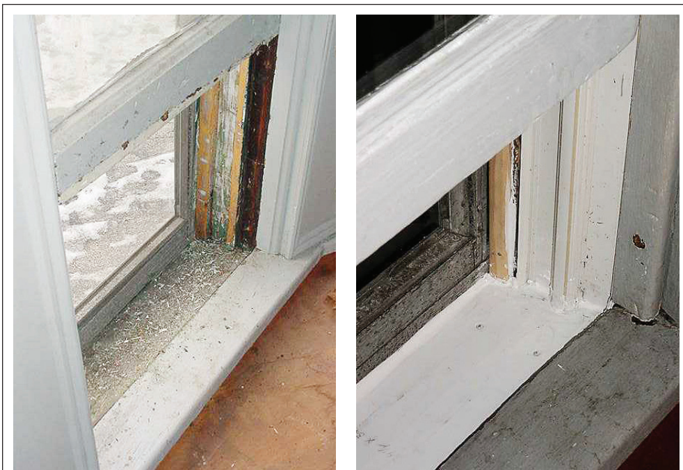
FIGURE 11.3 Window before and after friction treatment.
