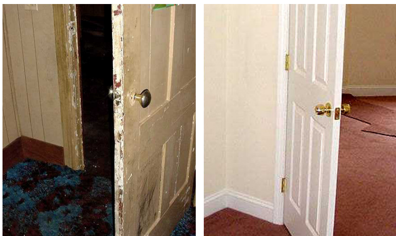
FIGURE 12.4 Pre-and post-abatement interior doors.
