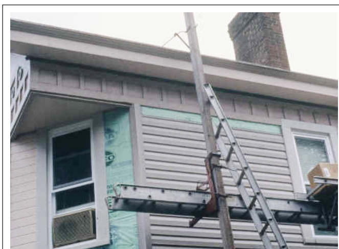
FIGURE 12.6 Installation of replacement siding.
