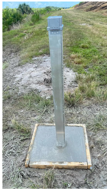
Typical Well Cover
