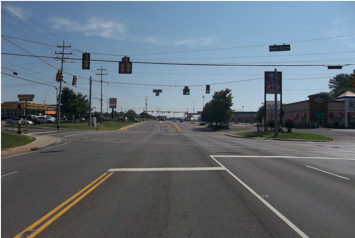
STATE ROUTE 76 AT HESTER DRIVE/CHARLES DRIVE – EASTBOUND APPROACH (L.M. 16.18)
