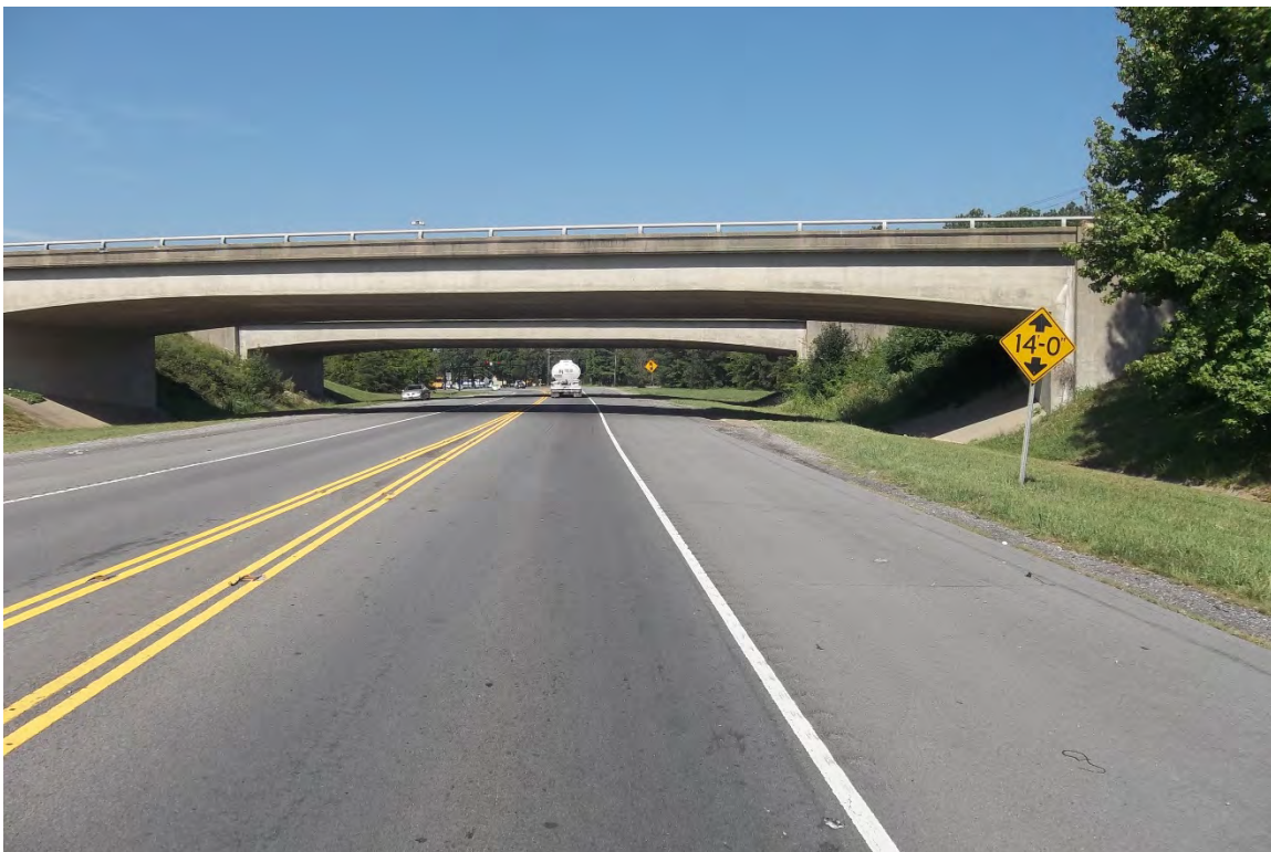
STATE ROUTE 76 LOOKING WEST NEAR THE INTERSTATE 65 UNDERPASS BRIDGES (L.M. 15.95)
