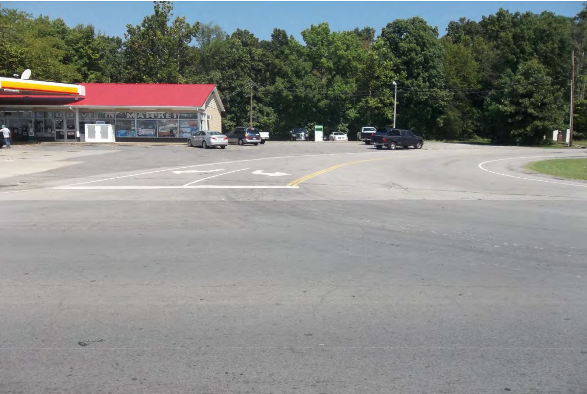
STATE ROUTE 76 AT INDUSTRIAL DRIVE – LOOKING NORTH ACROSS INTERSECTION (L.M. 15.66)
