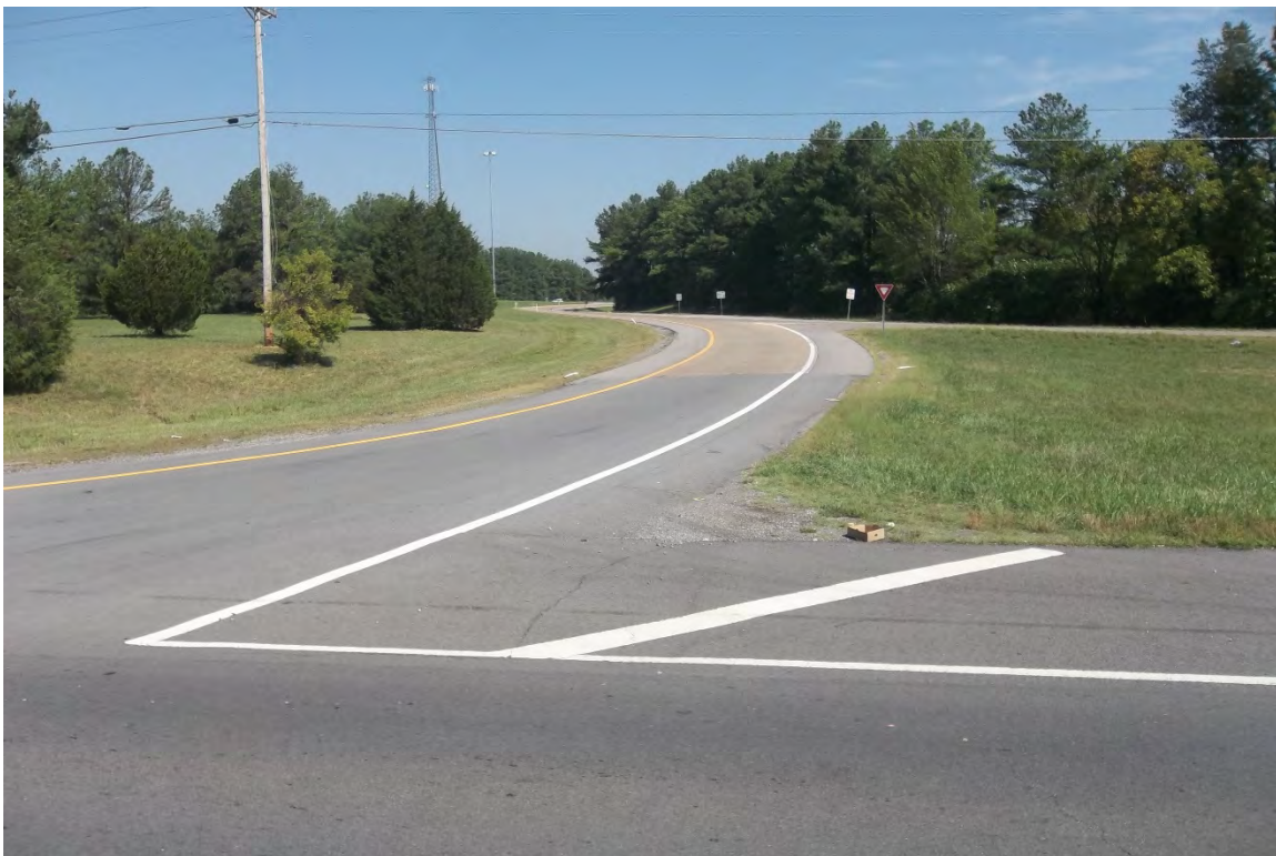
STATE ROUTE 76 LOOKING NORTH AT THE I-65 NORTHBOUND ON-RAMP (L.M. 16.03)
