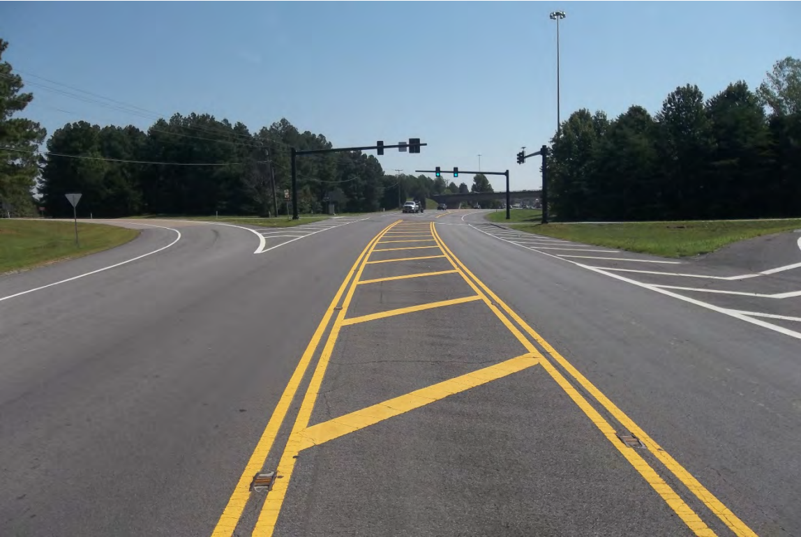
STATE ROUTE 76 AT THE I-65 SOUTHBOUND RAMPS – EASTBOUND APPROACH (L.M. 15.78)
