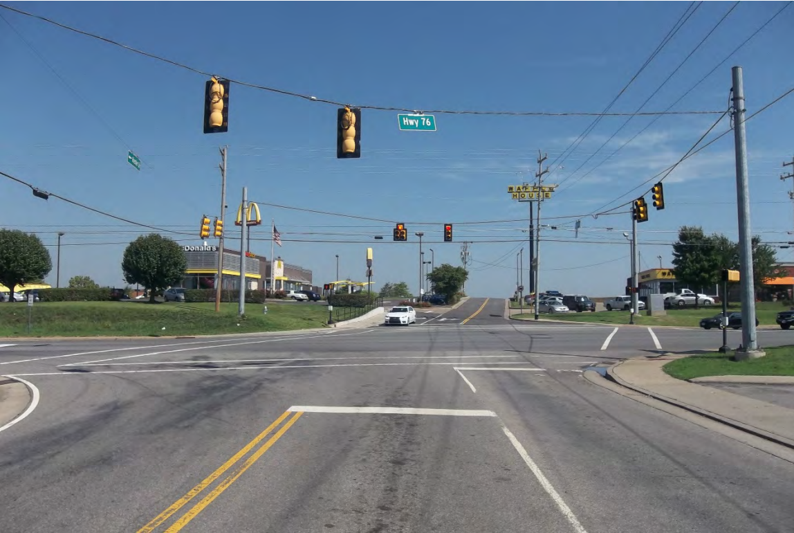
STATE ROUTE 76 AT HESTER DRIVE/CHARLES DRIVE – NORTHBOUND APPROACH (L.M. 16.18)
