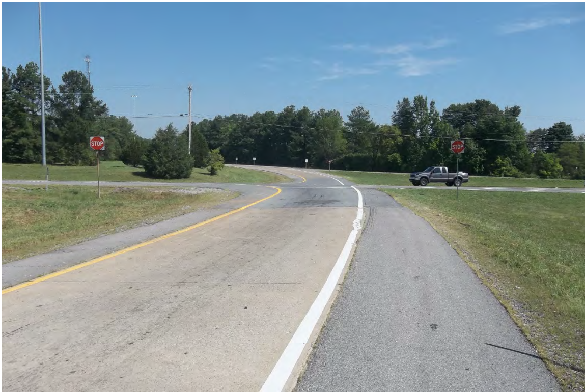
STATE ROUTE 76 AT THE I-65 NORTHBOUND RAMPS – NORTHBOUND APPROACH (L.M. 16.03)
