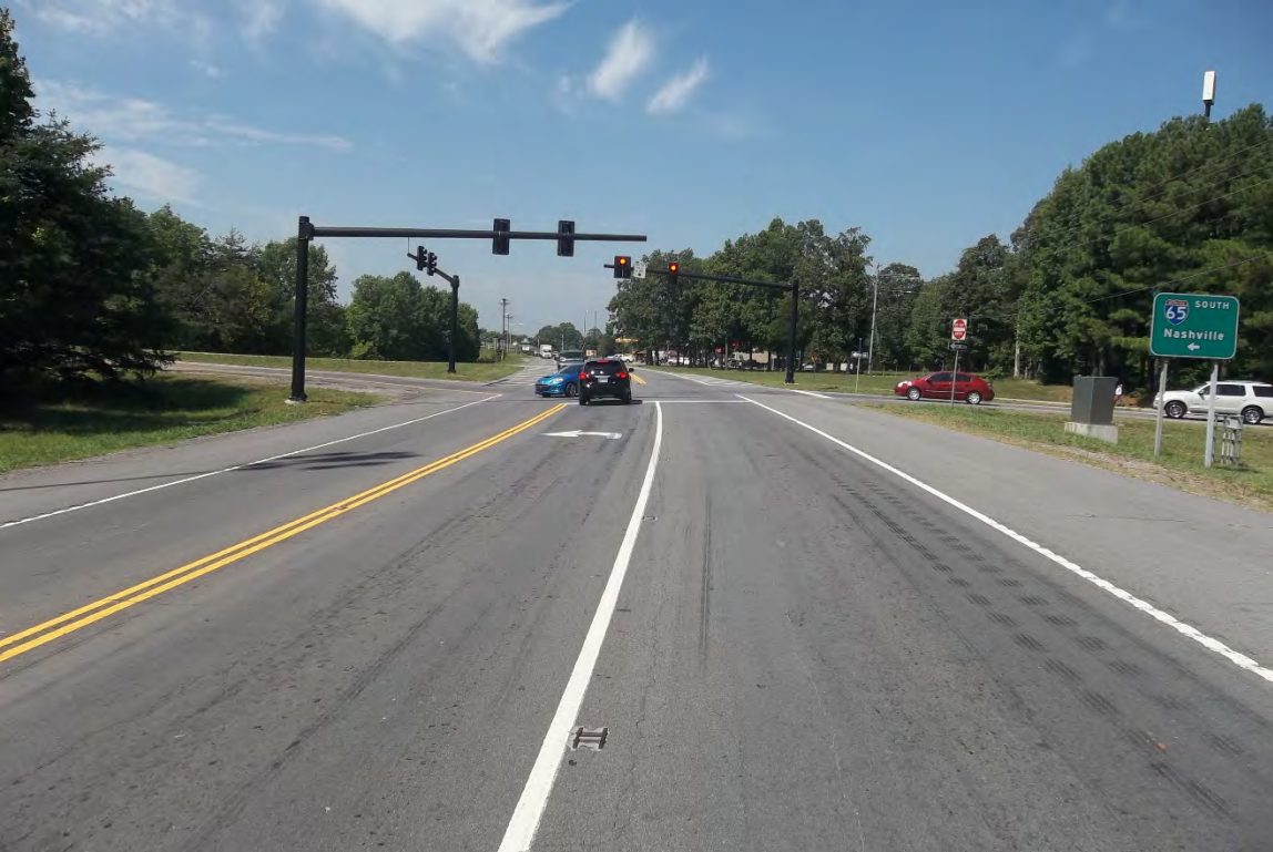
STATE ROUTE 76 AT THE I-65 SOUTHBOUND RAMPS – WESTBOUND APPROACH (L.M. 15.78)
