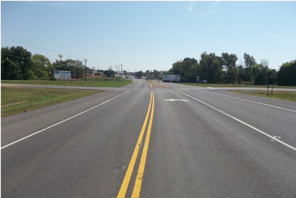
STATE ROUTE 76 AT THE I-65 NORTHBOUND RAMPS – EASTBOUND APPROACH (L.M. 16.03)
