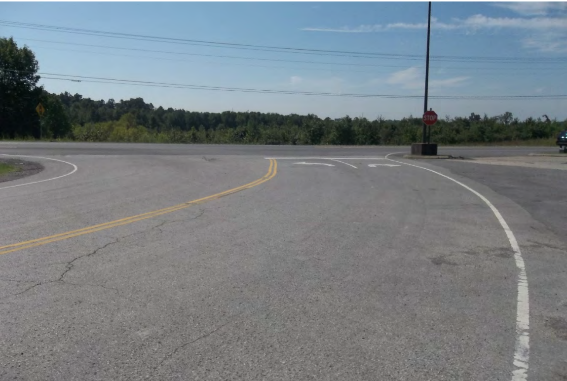
STATE ROUTE 76 AT INDUSTRIAL DRIVE – SOUTHBOUND APPROACH (L.M. 15.66)
