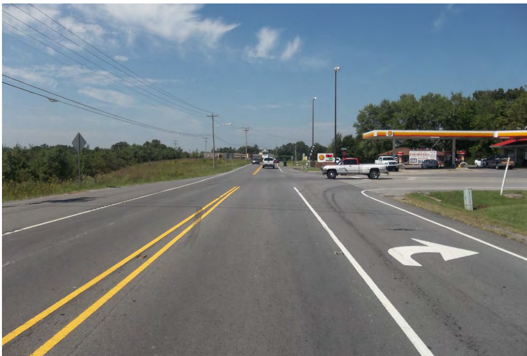
STATE ROUTE 76 AT INDUSTRIAL DRIVE – WESTBOUND APPROACH (L.M. 15.66)
