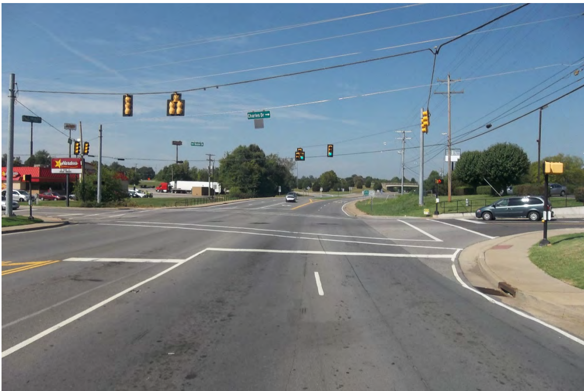
STATE ROUTE 76 AT HESTER DRIVE/CHARLES DRIVE – WESTBOUND APPROACH (L.M. 16.18)
