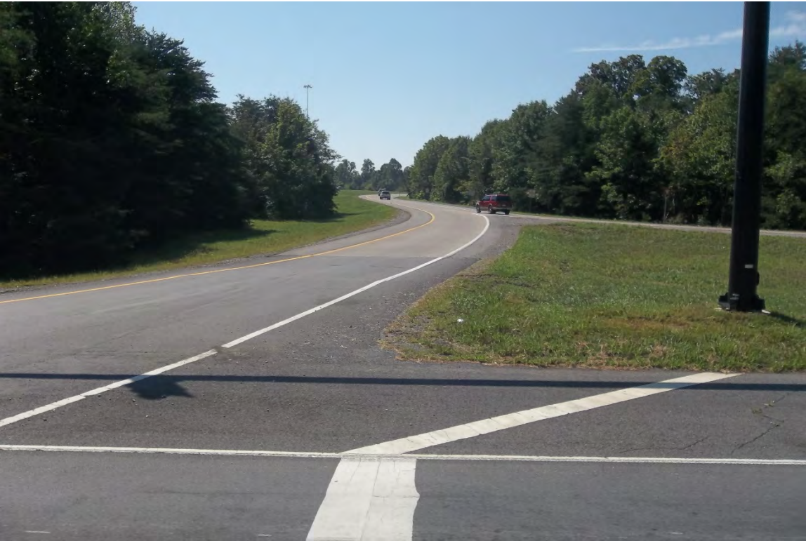
STATE ROUTE 76 LOOKING SOUTH AT THE INTERSTATE 65 SOUTHBOUND ON-RAMP (L.M. 15.78)
