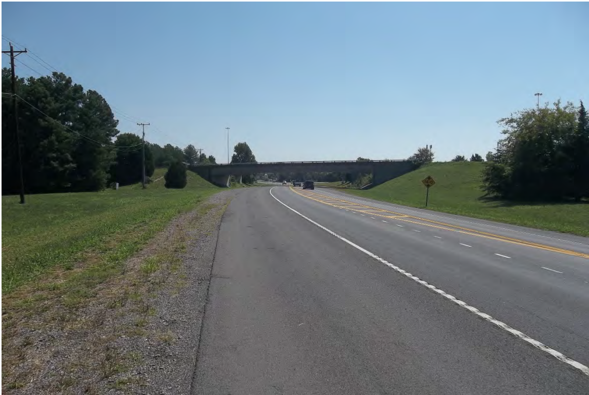
STATE ROUTE 76 LOOKING EAST NEAR THE INTERSTATE 65 UNDERPASS BRIDGES (L.M. 15.86)
