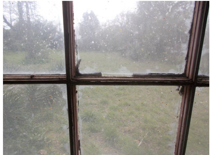
Photo 4 – Wooden window glazing.
