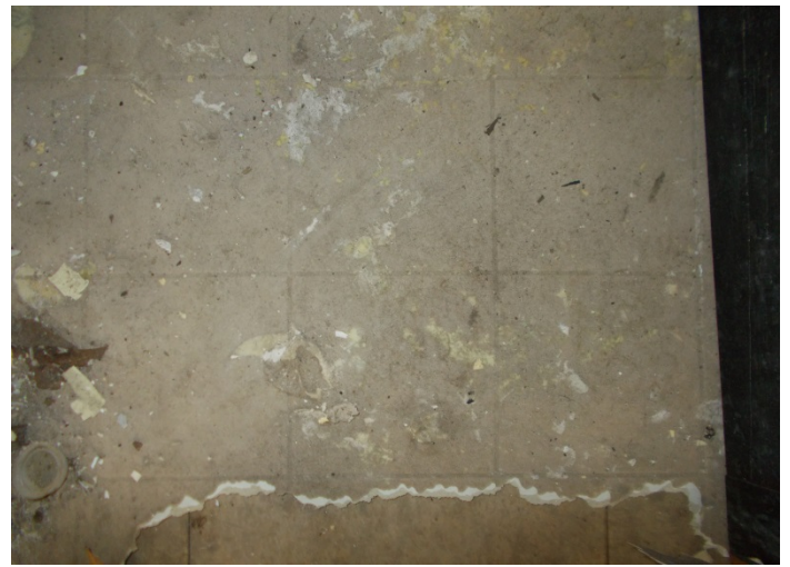
Photo 10 – Cream square pattern vinyl floor with no mastic.
