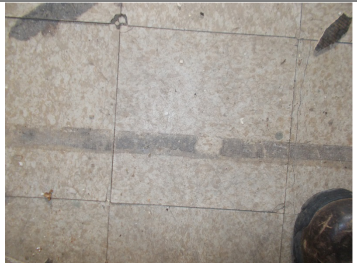
Photo 8 – 9"x9" beige speckled pattern vinyl floor tile with mastic.
