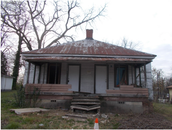
Photo 1 -- 369 Farley Street in Spartanburg, SC.
