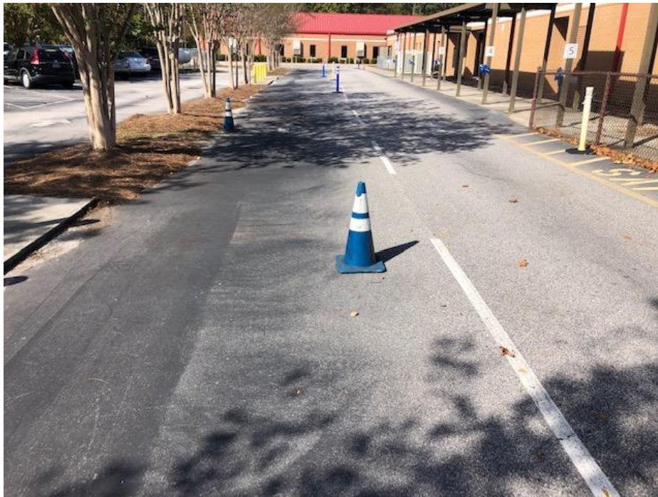
Figure 2: Good to fair pavement conditions
