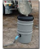
Figure 3. Concrete washout filter
