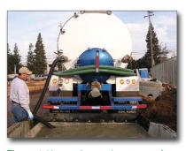
**Figure 4.** Vacuuming washwater out of a washout container for treatment and reuse
