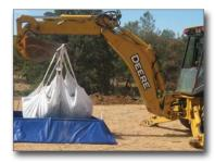
Figure 12. Extracting the concrete solids or gelled washwater
