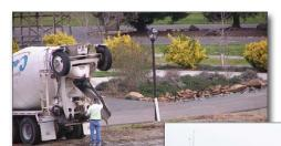
**Figure 1.** Chute washwater being dumped on the ground
