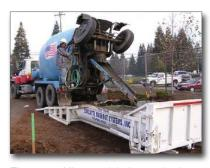
Figure 13. Mixer truck being washed out into a roll-off bin
