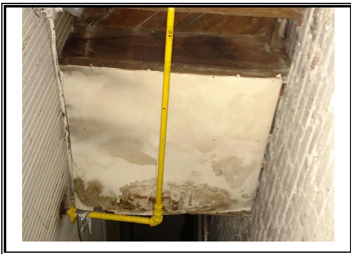
4. View of drywall in stairwell.
