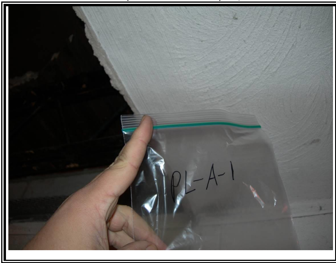
3. View of plaster ceiling.
