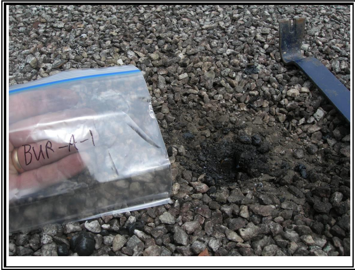
7. View of built up roofing on the main roof.
