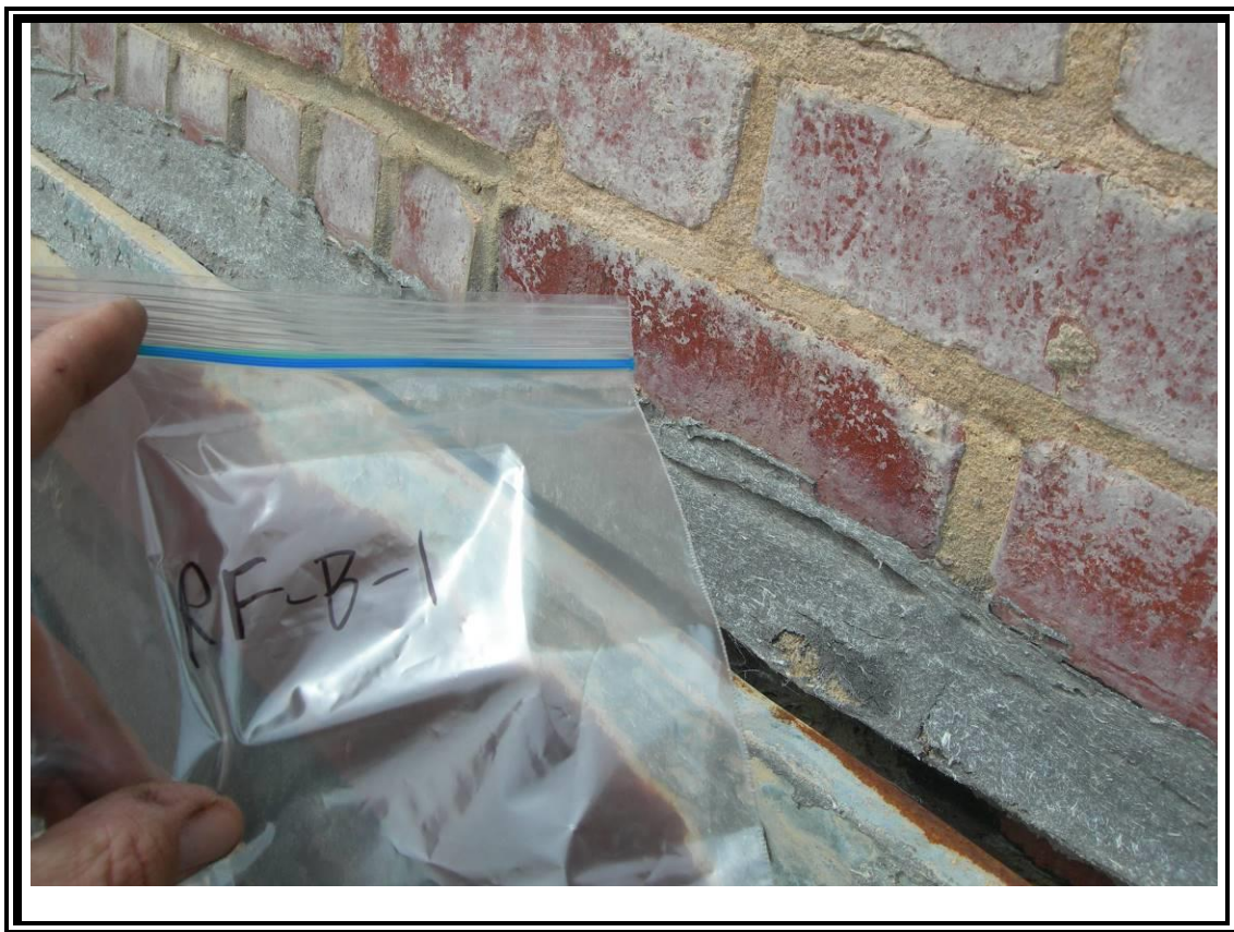
8. View of roof flashing on east side roof.
