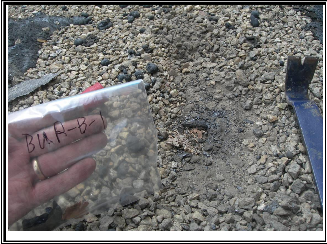
9. View of built up roofing on east side roof.
