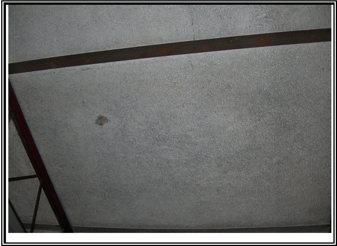
5. View of roof deck on east side of the building.
