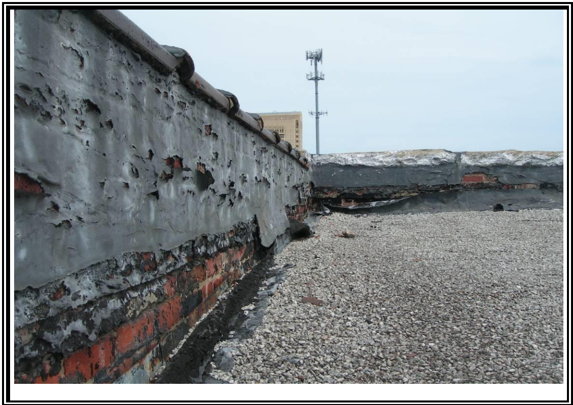
6. View of roof flashing on main roof.
