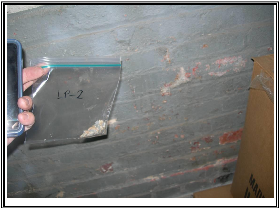
12. View of interior gray paint.
