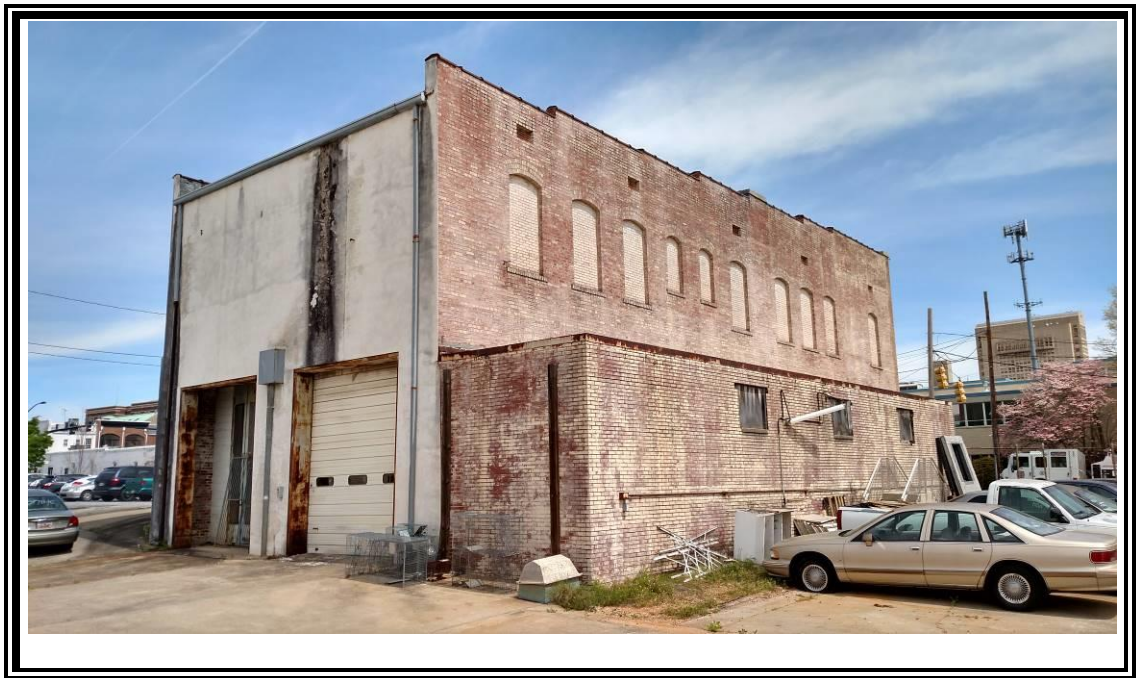
2. View of plaster exterior on rear.
