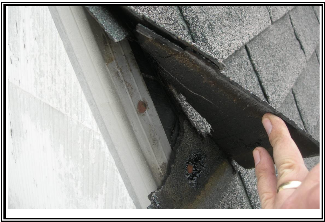
6. View of roofing shingles and felt paper on roof vent.
