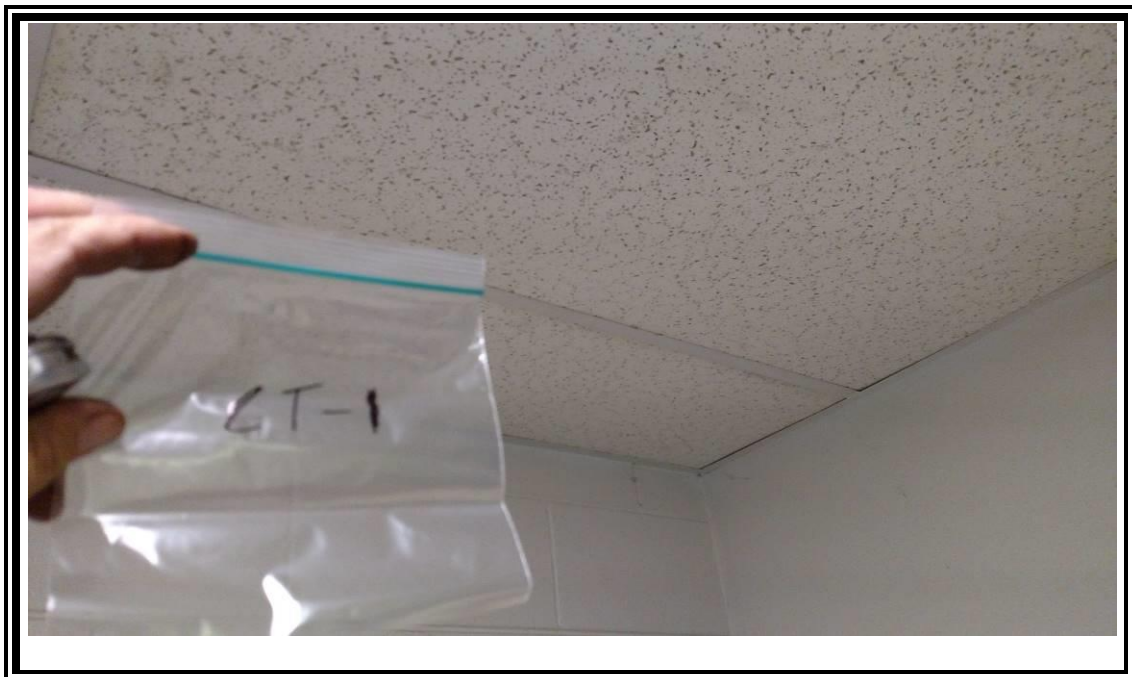
12. View of ceiling tile in the office area.
