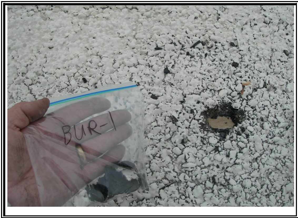
8. View of built up roofing.
