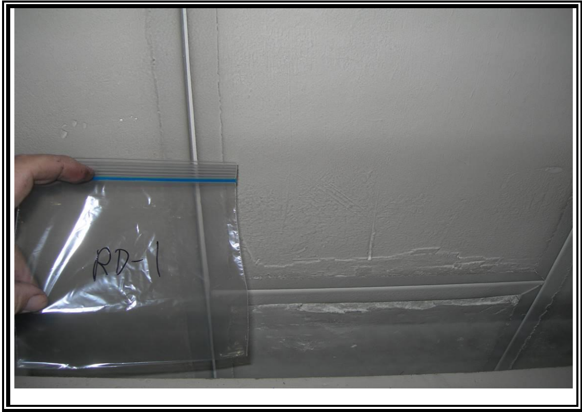
9. View of roof decking.
