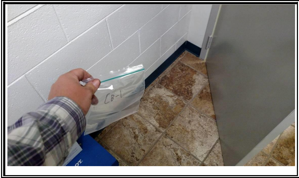
11. View of cove base in the office area.
