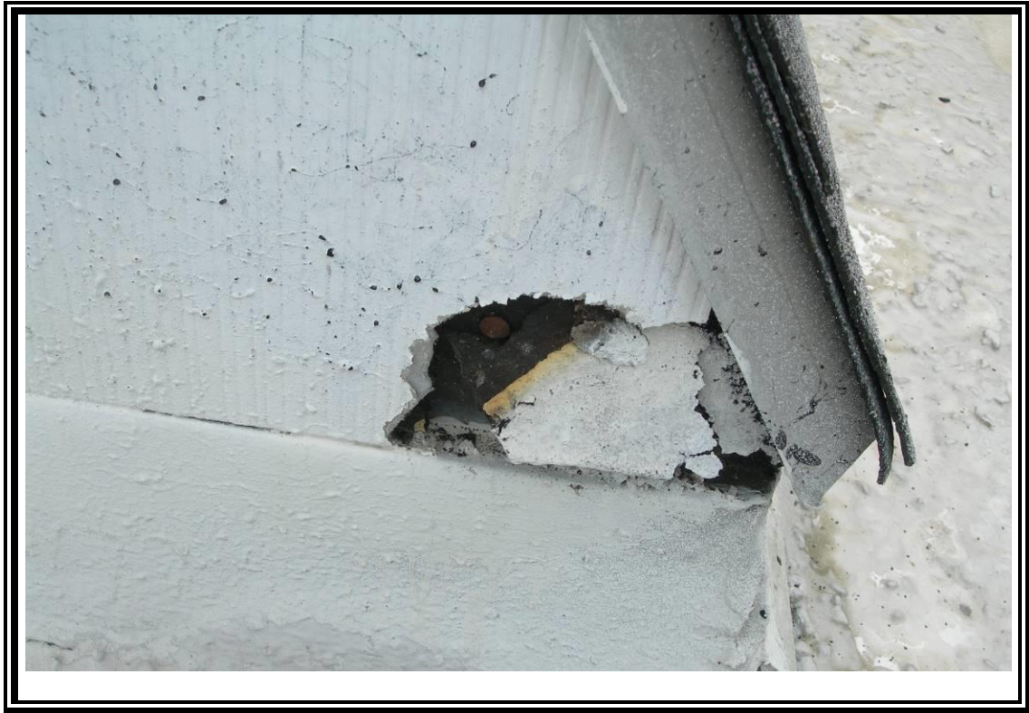
5. View of felt paper under cement tiles on roof vent.
