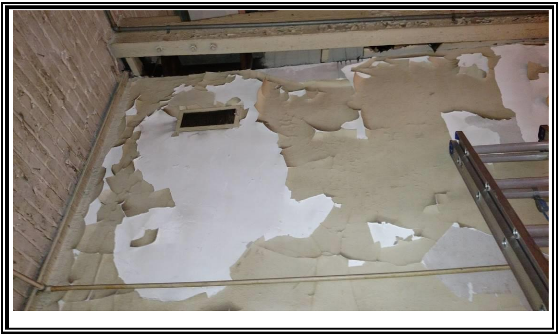
14. View of plaster wall and Interior tan paint.
