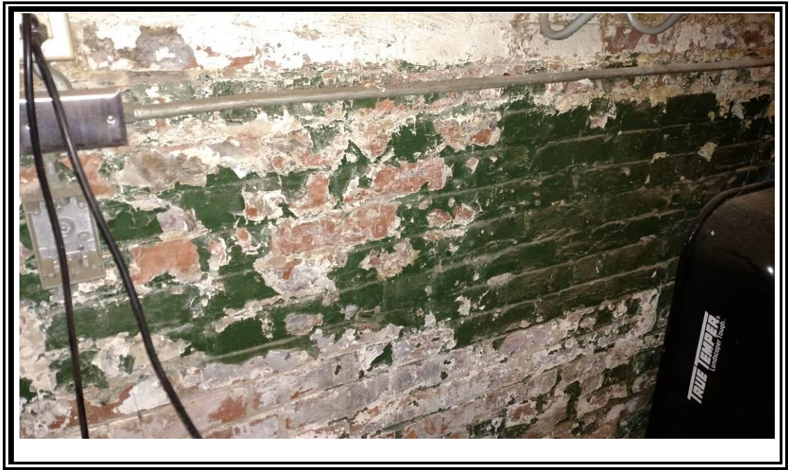
15. View of interior green paint.
