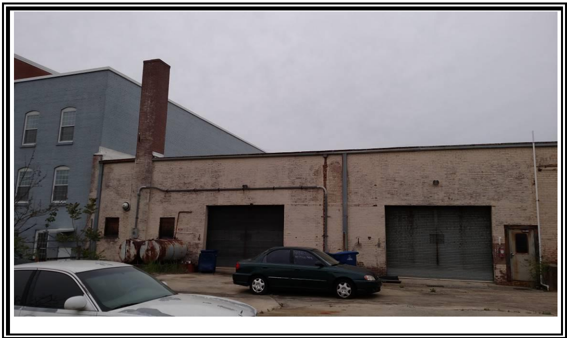
2. View of rear of building.
