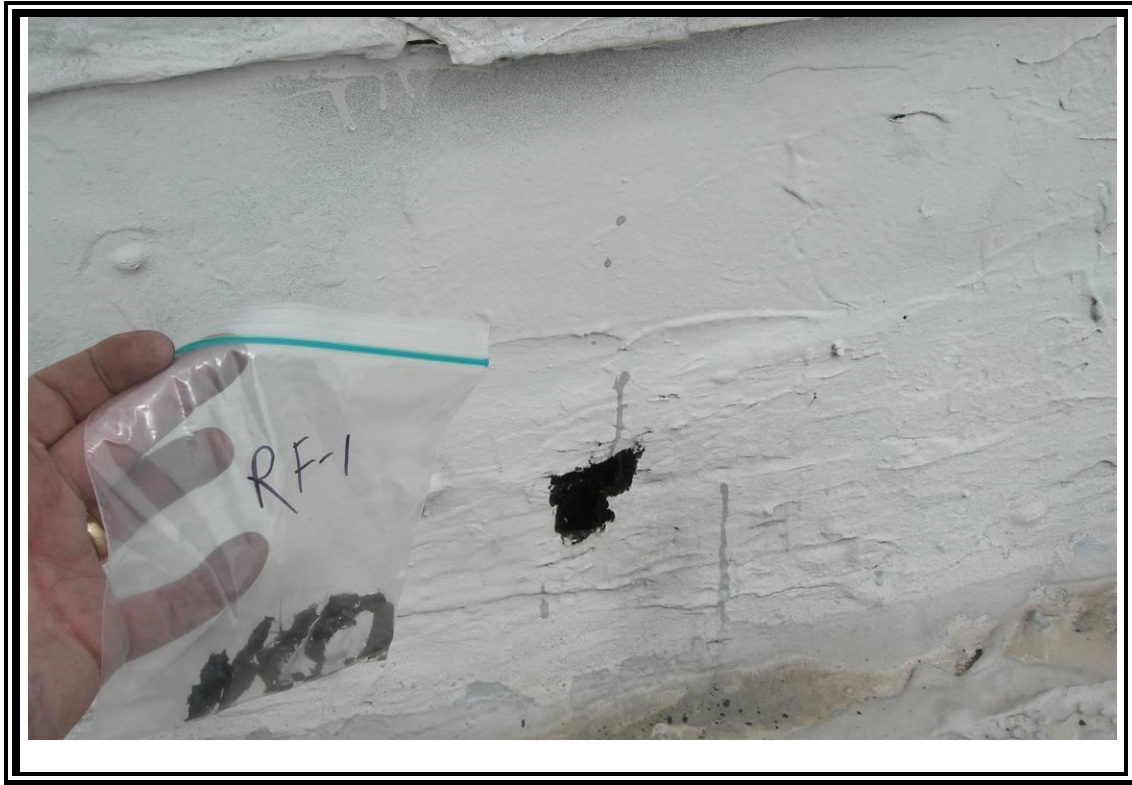
7. View of roof flashing.
