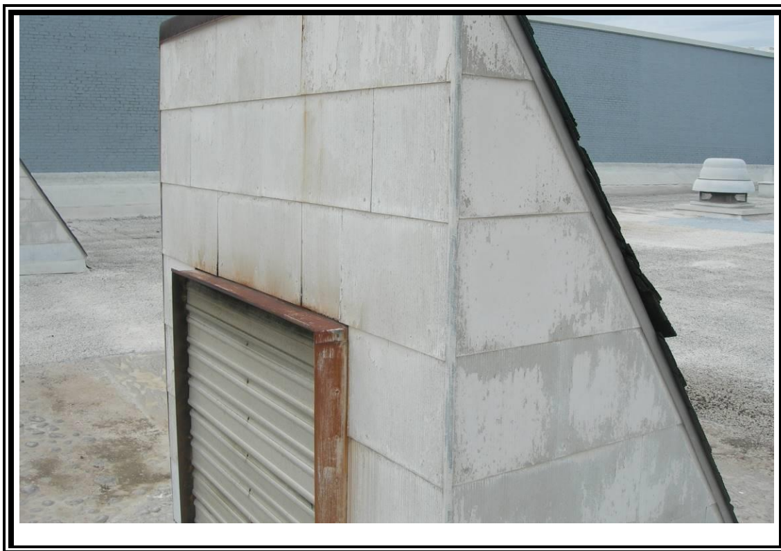
4. View of cement tiles on roof vent.
