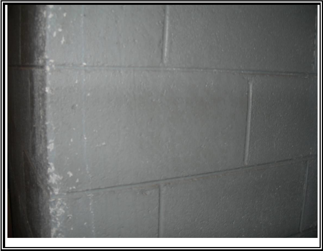
13. View of interior gray paint.
