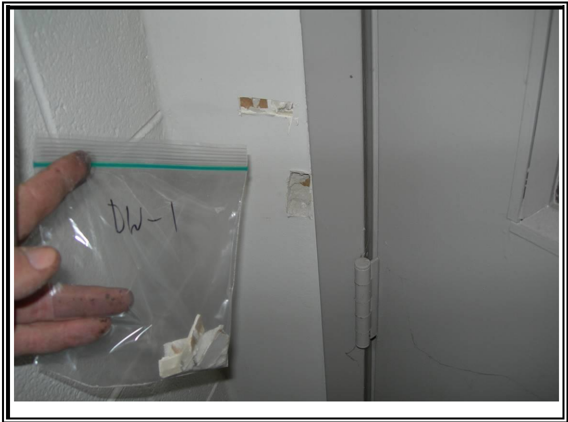
10. View of drywall and joint compound in the office area.
