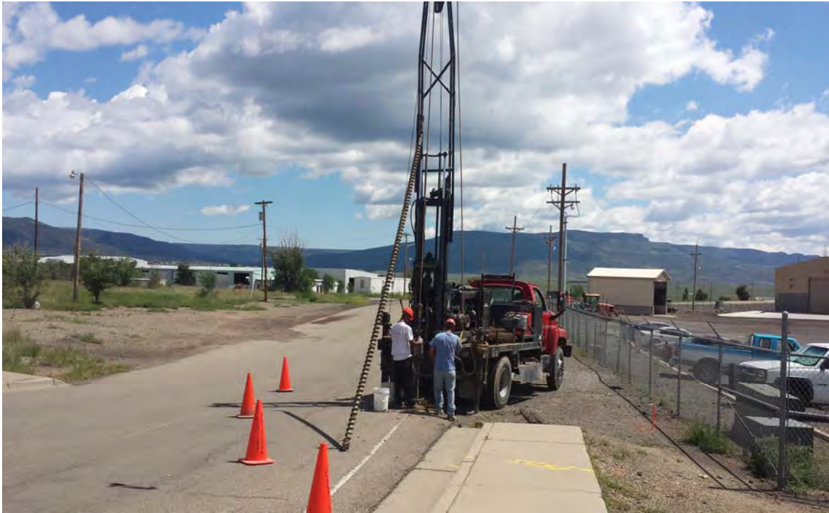
DRILLING BORING B-2 (MANHOLE STRUCTURE) - LOOKING SOUTHEAST
