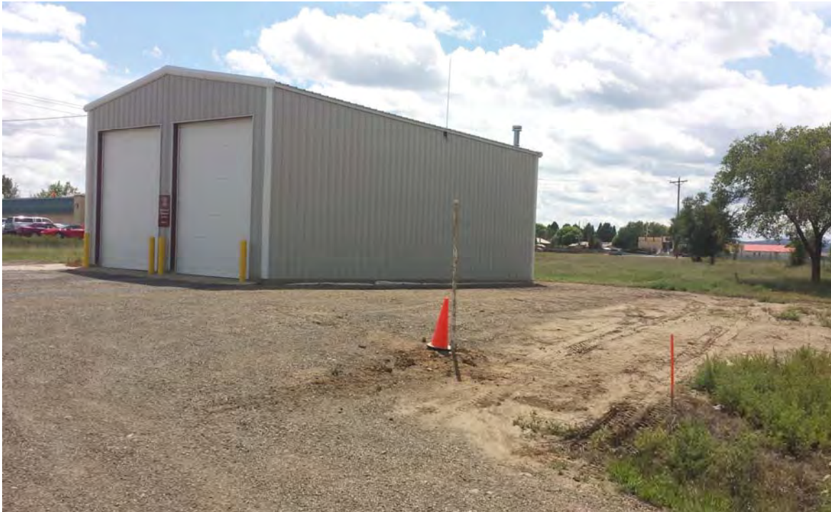
BORING B-1 (LIFT STATION SITE) - LOOKING SOUTHWEST
