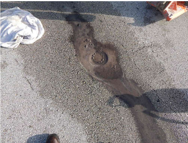
Photo 9: Weak asphalt matrix washing out of core hole C-4
