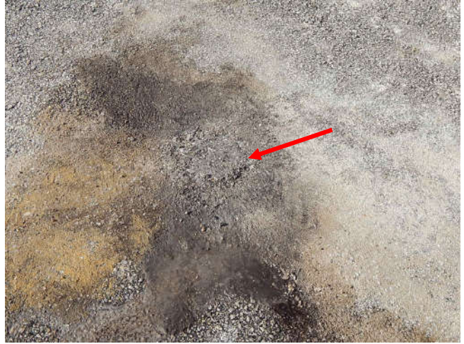
Photo 8: Patched asphalt
