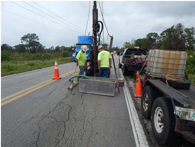
Photo 1: Installation of boring
