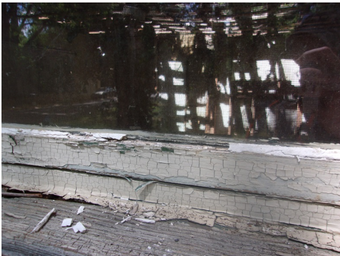
Photo 5 – Wooden window glazing
