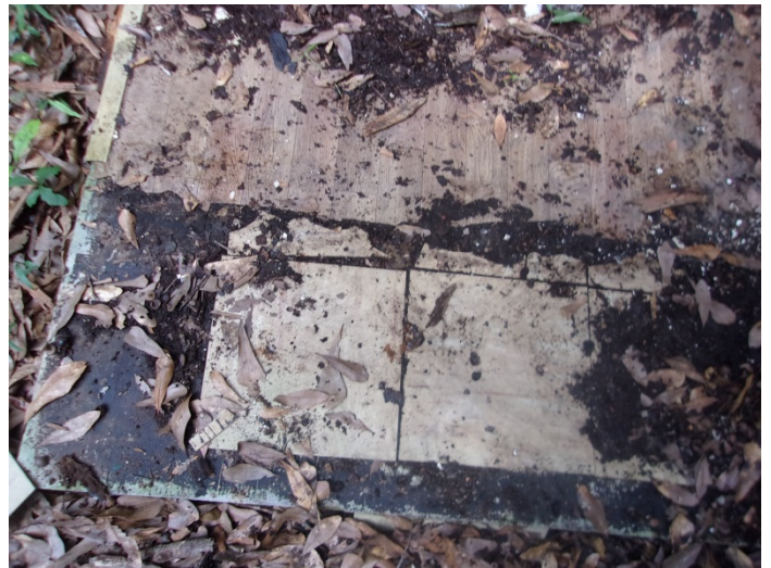
Photo 10 – 9" x 9" tan floor tile & black mastic in the kitchen landing
