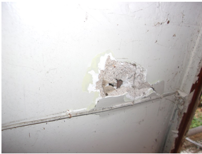
Photo 7 – Plaster & finish throughout on the walls
