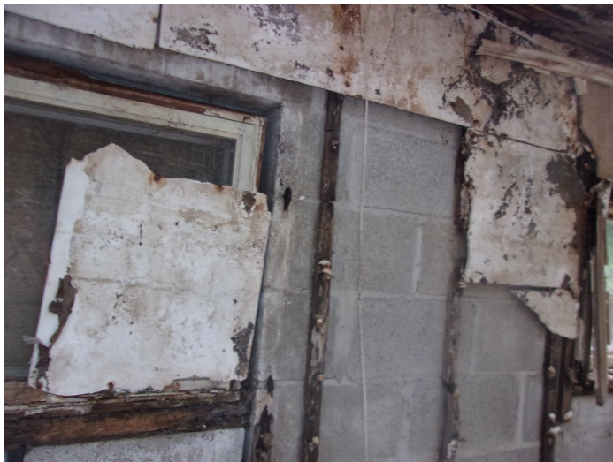
Photo 9 – Unfinished hard white wall beneath the plaster walls throughout
