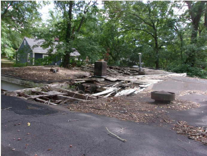
Photo 3 – Tar on 2 chimney's & 4 vents & roll roof shingles with felt & tar on the house roof
