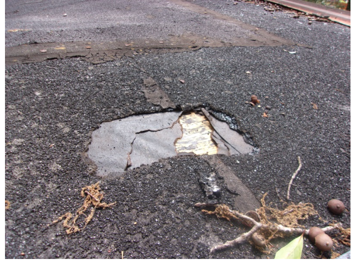
Photo 2 – Roll roof shingles with felt & tar on the house roof
