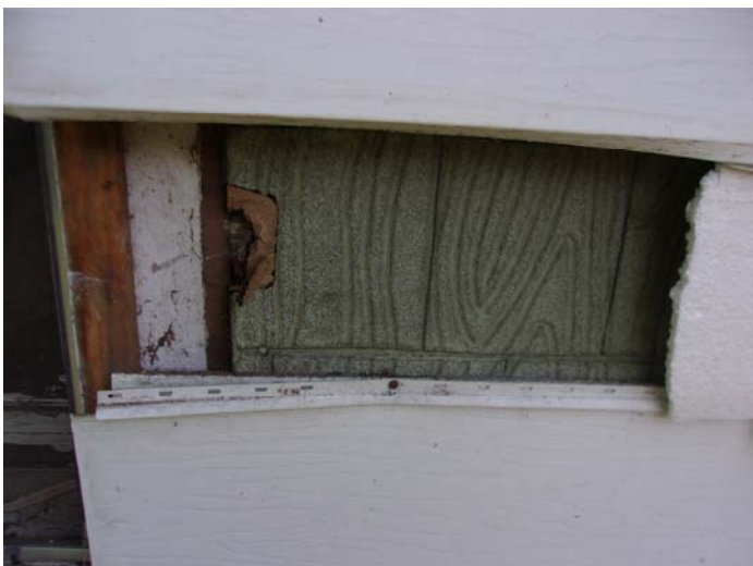
Photo 5 – Pressboard siding with shingle layer under metal
