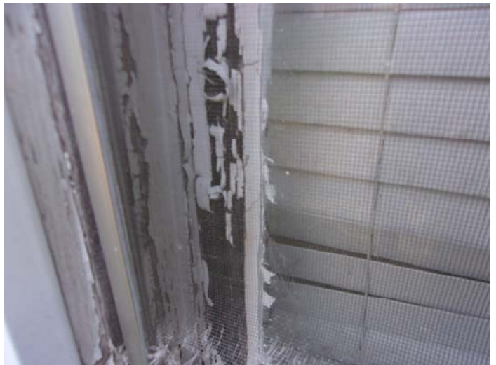
Photo 4 – Wooden window glazing
