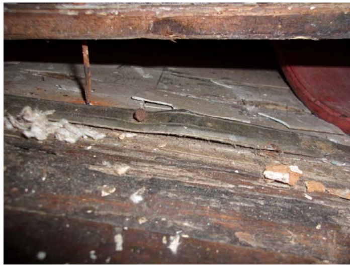
Photo 13 – White floor tiles & mastic in the bathroom under wooden flooring
