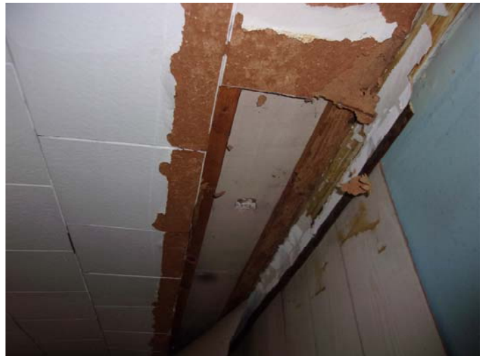
Photo 10 – Drywall with joint compound & tape under 12" x 12" wooden ceiling tiles
