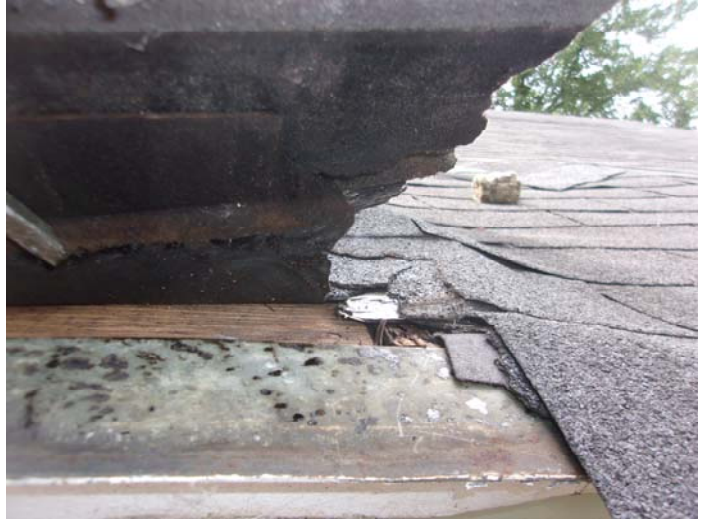
Photo 2 – Roof shingles & felt
