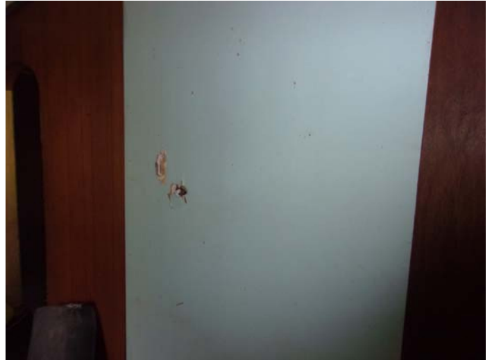
Photo 8 – Drywall with joint compound & tape under wooden wall panels
