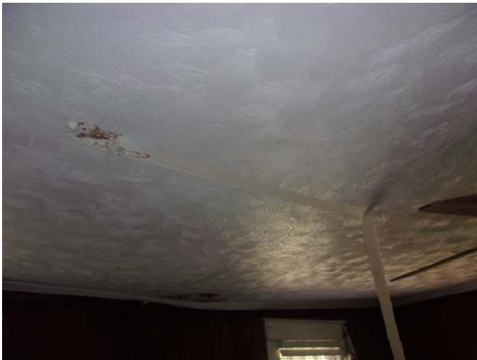
Photo 9 – Drywall with joint compound & tape
