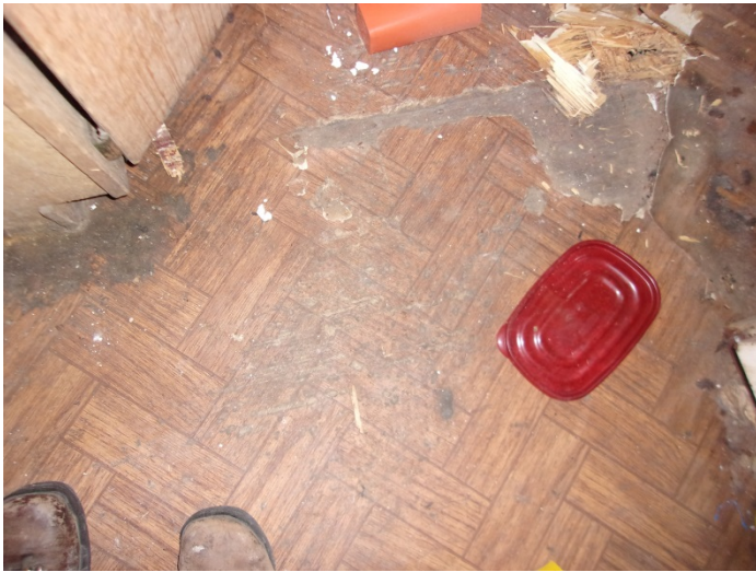
Photo 19 – Brown wooden pattern vinyl floor & mastic in the kitchen
