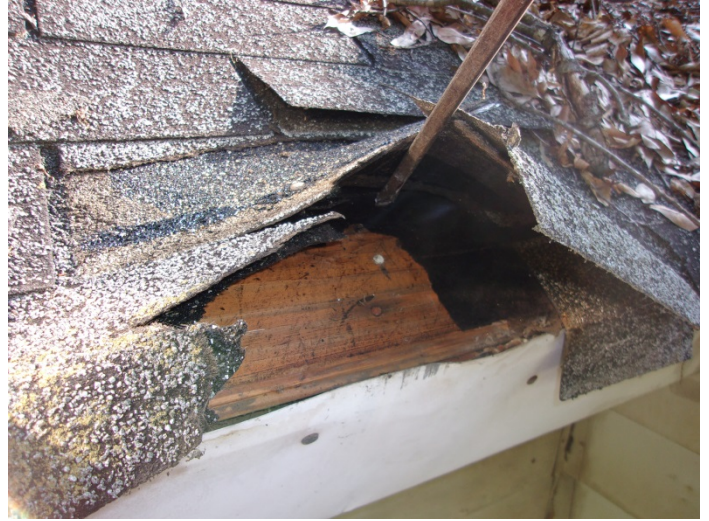
Photo 2 – Roof shingles & felt
