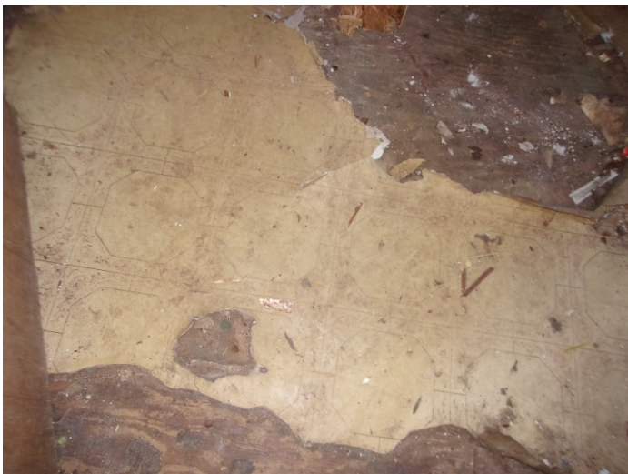
Photo 17 – Yellow square & floral pattern vinyl floor with no mastic in the back hallway
