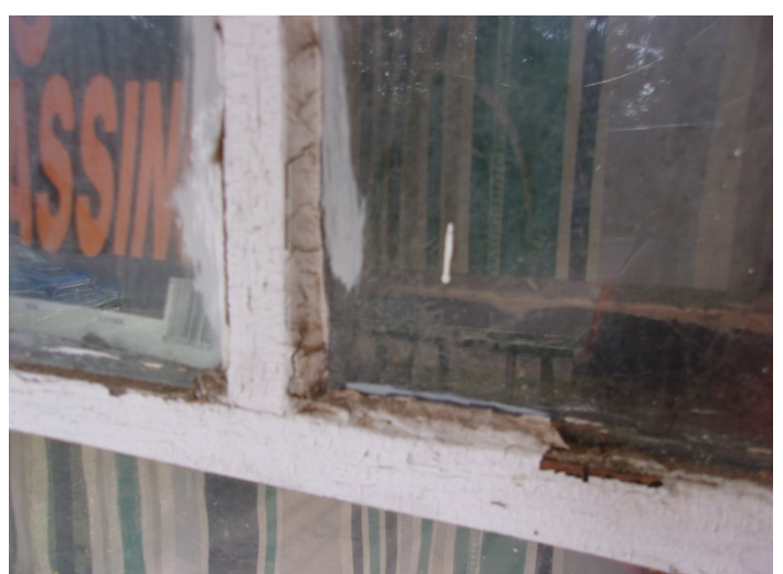
Photo 6 – Wooden window glazing
