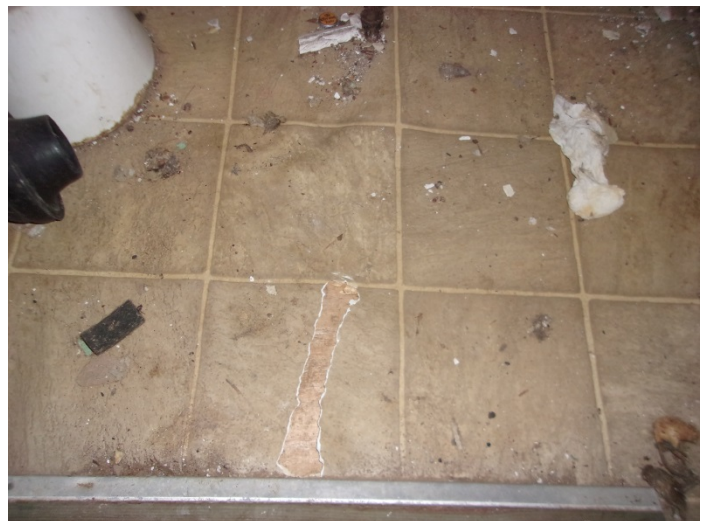
Photo 18 – Tan square pattern vinyl floor with no mastic in the bathroom
