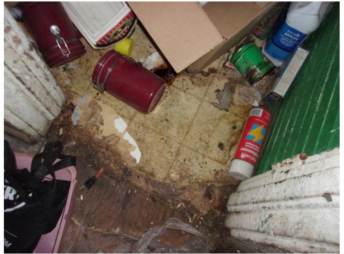
Photo 20 – Beige square pattern vinyl floor & mastic in the kitchen pantry
