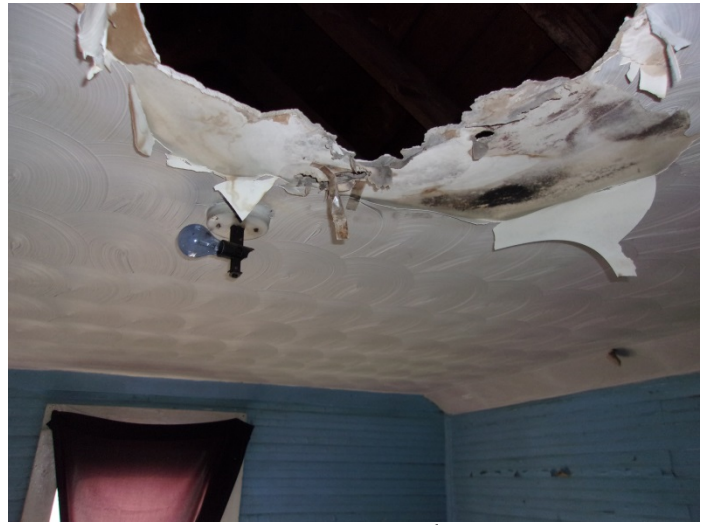
Photo 8 – Swirl ceiling texture in the 2 nd floor front bedroom
