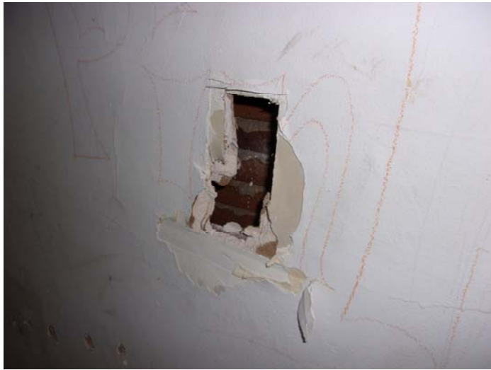
Photo 7 – Drywall with joint compound & tape throughout
