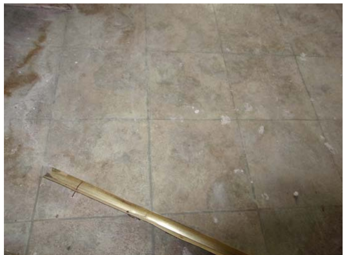
Photo 12 – Beige square pattern vinyl floor & mastic in the main level - kitchen
