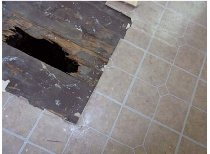
Photo 10 – Gray square diamond pattern self-stick floor tile & mastic in the main level – front left room
