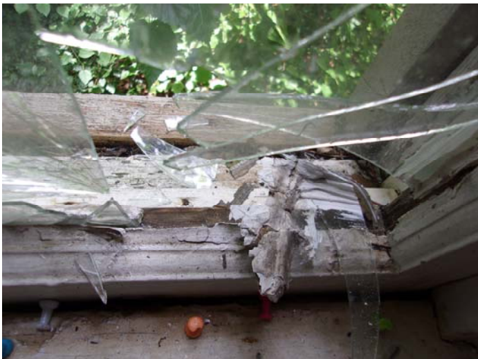
Photo 5 – Caulk on the glass panes on the wooden windows
