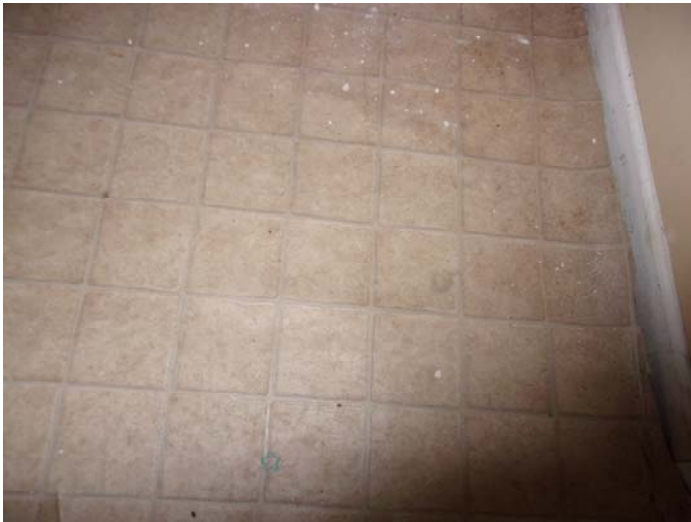
Photo 15 – Beige small square vinyl floor & leveling compound in the basement - hallway
