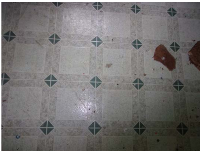
Photo 11 – Gray square blue diamond pattern vinyl floor & mastic in the main level – laundry room & bathroom
