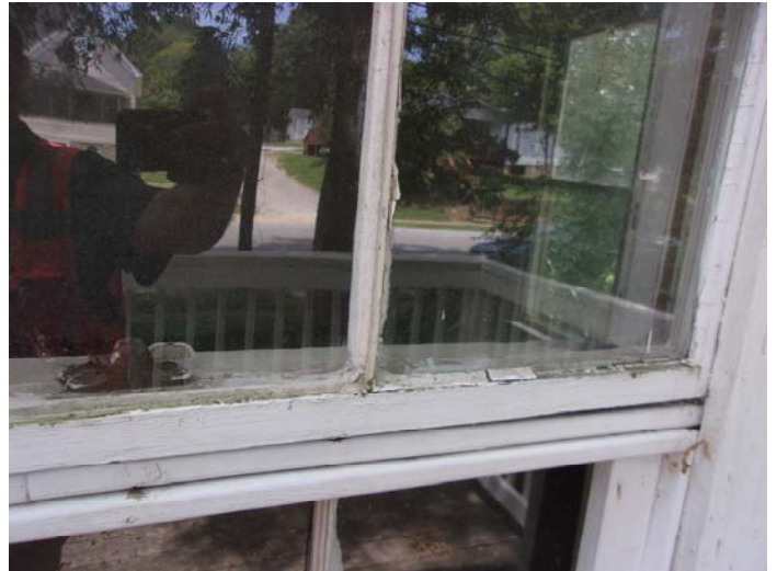
Photo 4 – Wooden window glazing
