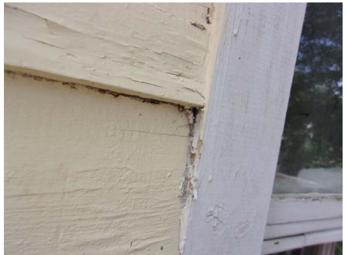
Photo 6 – Caulk on the wooden window casings
