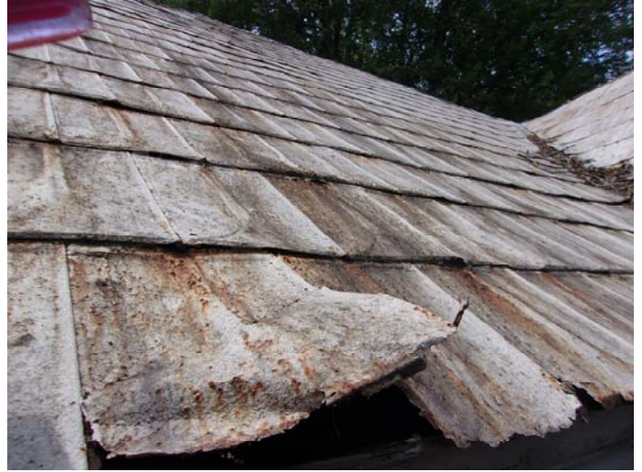
Photo 2 – Metal roof sealant
