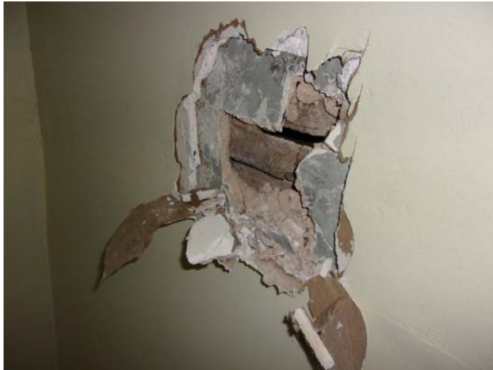
Photo 9 – Drywall with joint compound & tape over plaster with finish
