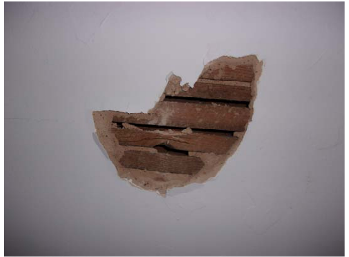
Photo 8 – Plaster with finish throughout
