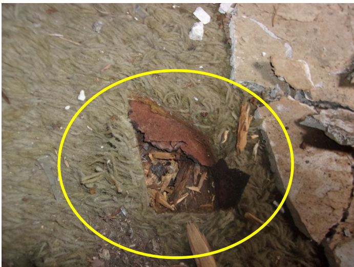
Photo 11 – Black pattern vinyl floor with felt backing in the front right bedroom under carpet
