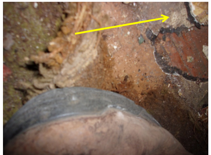
Photo 12 – Brown pattern vinyl floor with felt backing in the living room (under carpet) & dining room (3rd layer)
