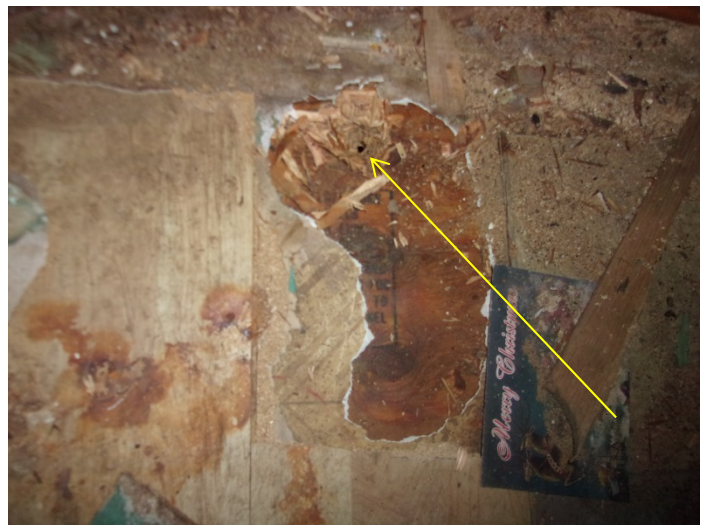
Photo 14 – Yellow pattern vinyl floor & mastic in the kitchen under wood
