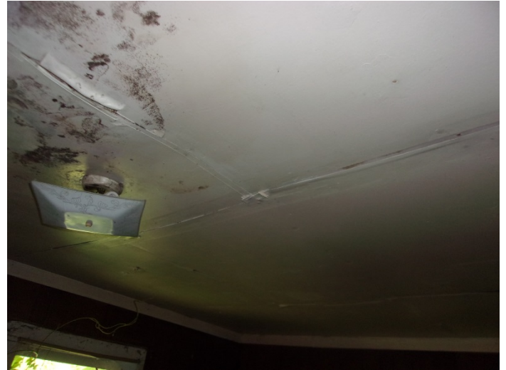
Photo 10 – Drywall with joint compound & tape throughout
