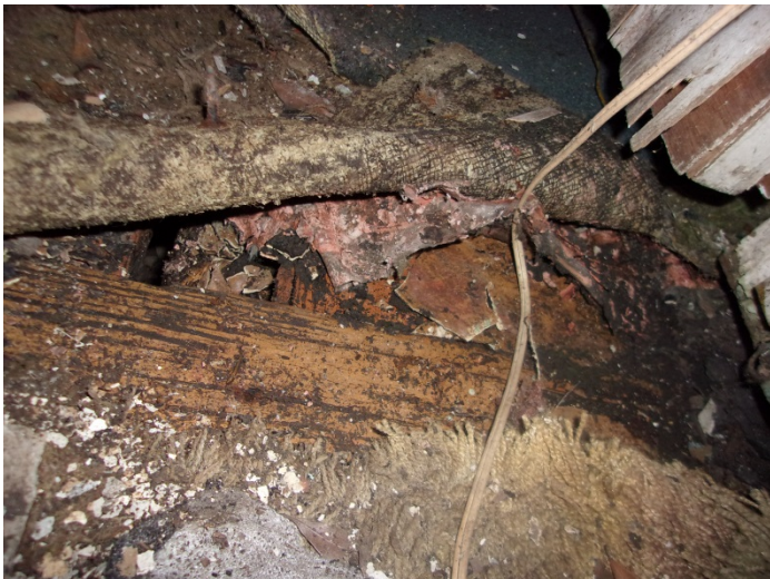
Photo 15 – Brown/black pattern vinyl floor with felt backing in the middle left bedroom under carpet
