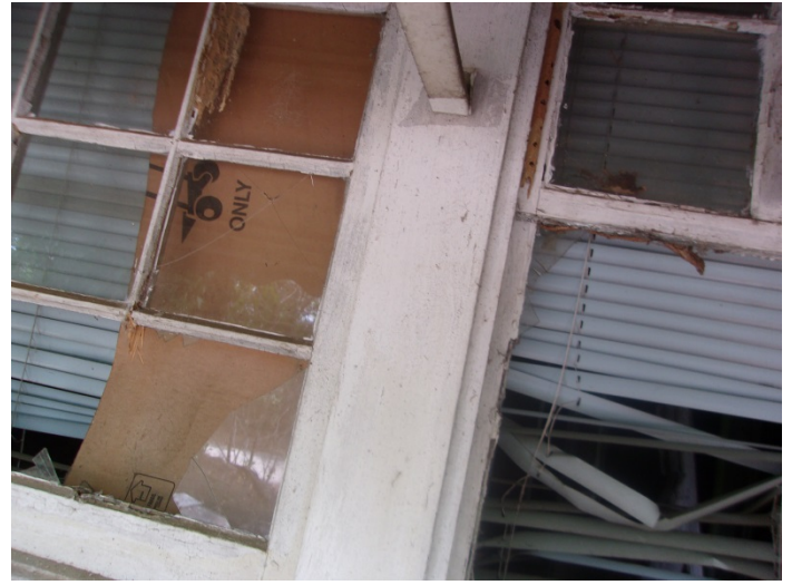
Photo 8 – Wooden window glazing & caulk on glass panes
