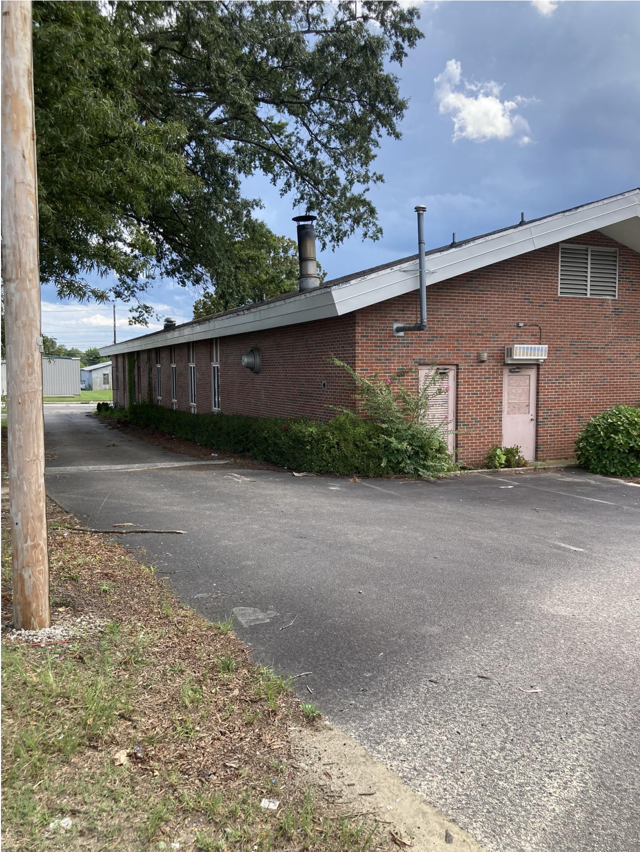
316 Tarboro Street – Salvation Army Main Bldg. Pictures
