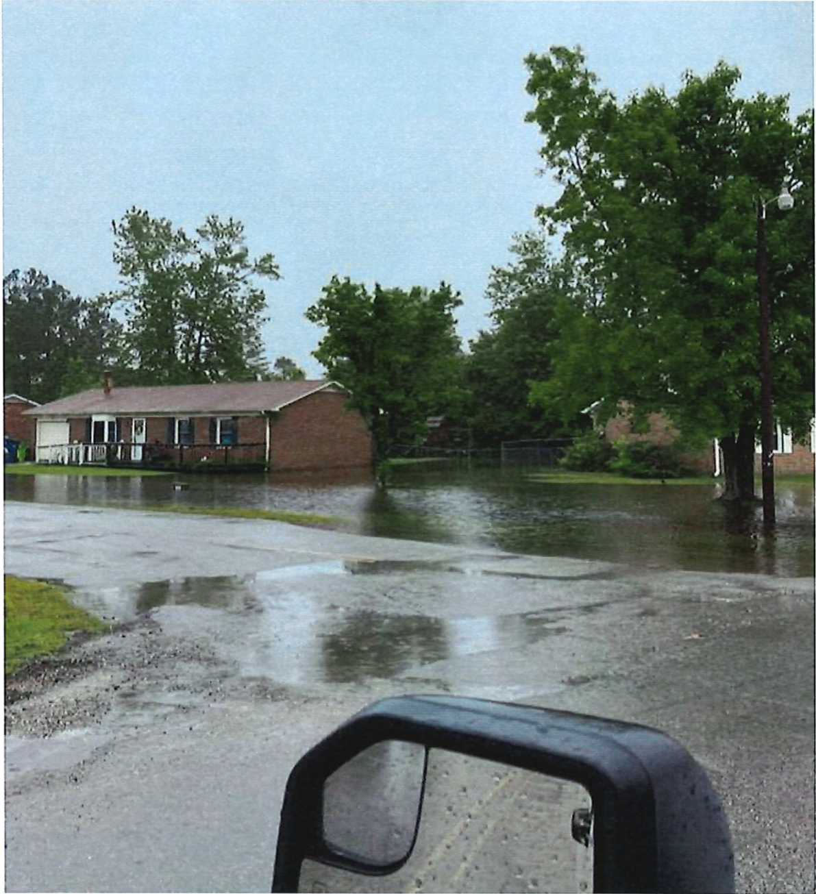
Yard and structure flooding in a residential area of Havelock during a normal heavy rain event
