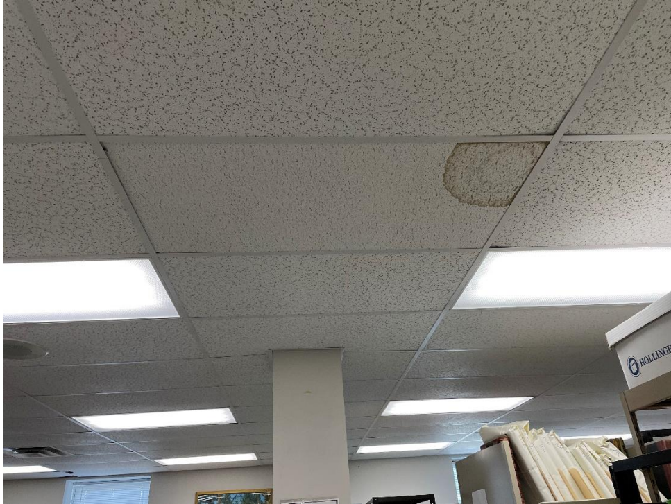
Photograph 11: View of ceiling in the archivist floor.
