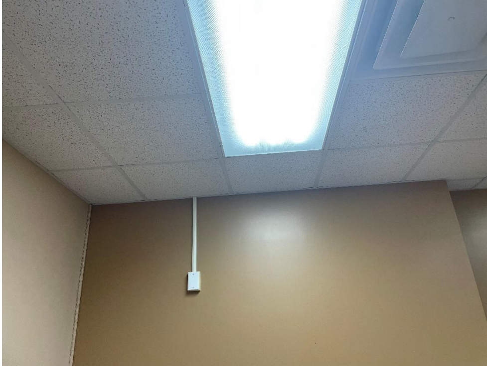
Photograph 9: View of ceiling.
