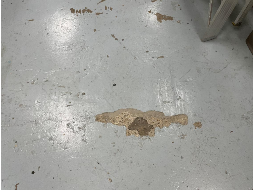
Photograph 5: Additional view of concrete floor in the archivist room.
