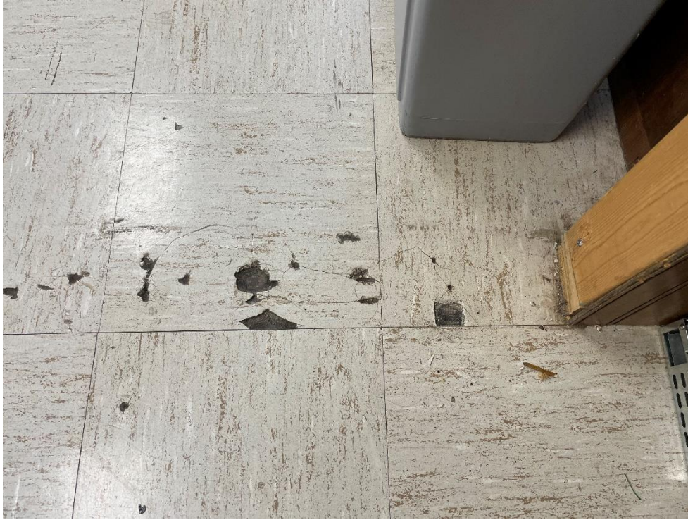
Photograph 3: Additional view of tile floor in the breakroom.
