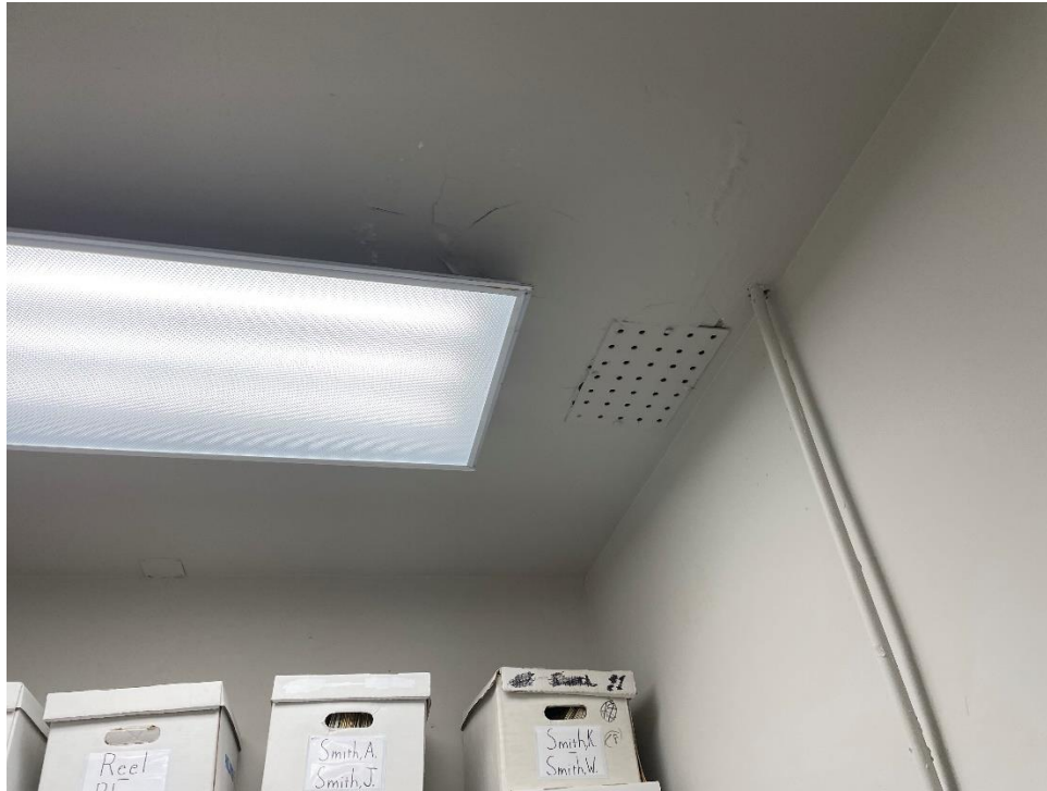
Photograph 10: View of ceiling in the archivist floor.
