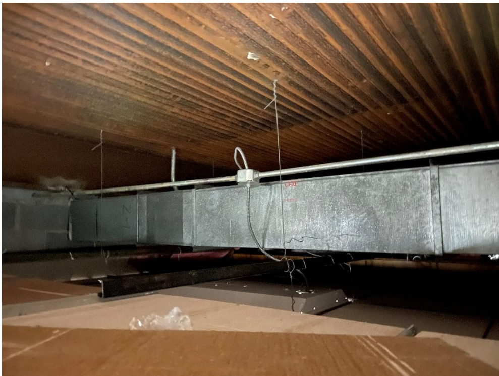
Photograph 8: Additional view of the airduct.
