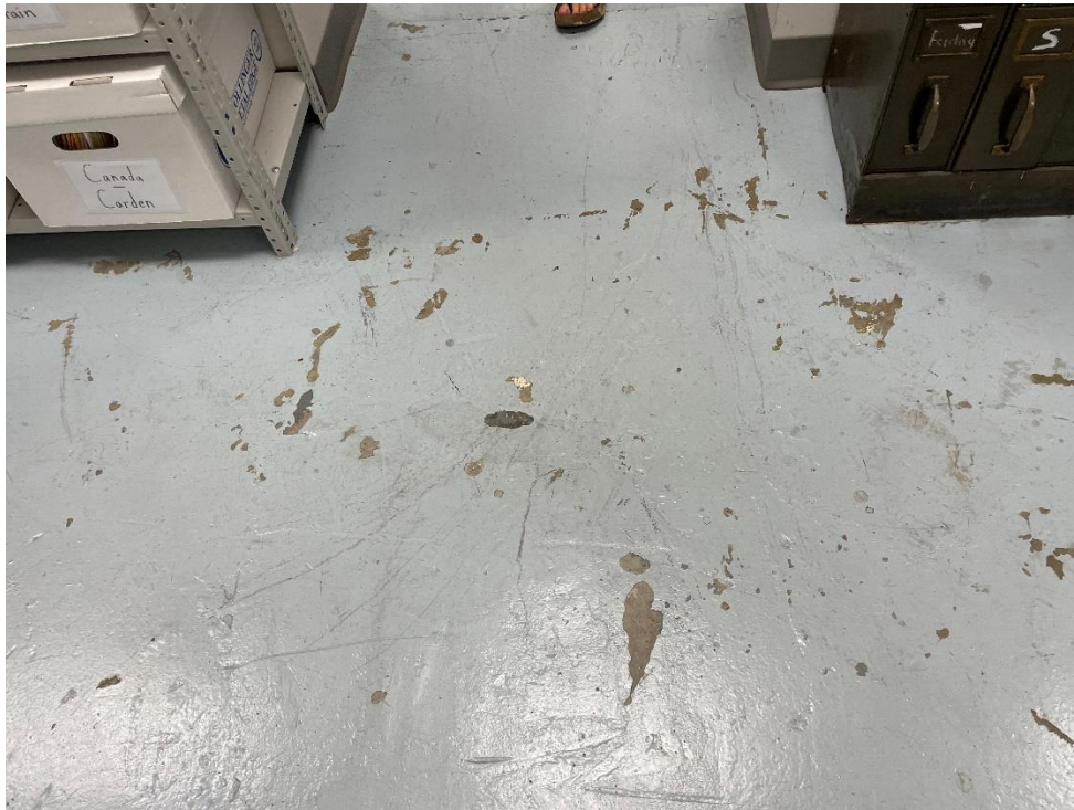
Photograph 4: View of concrete floor in archivist room.
