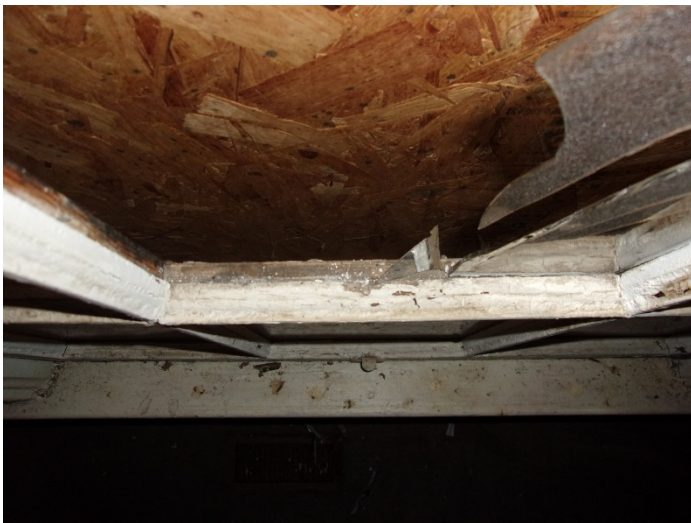
Photo 3 – Wooden window glazing.
