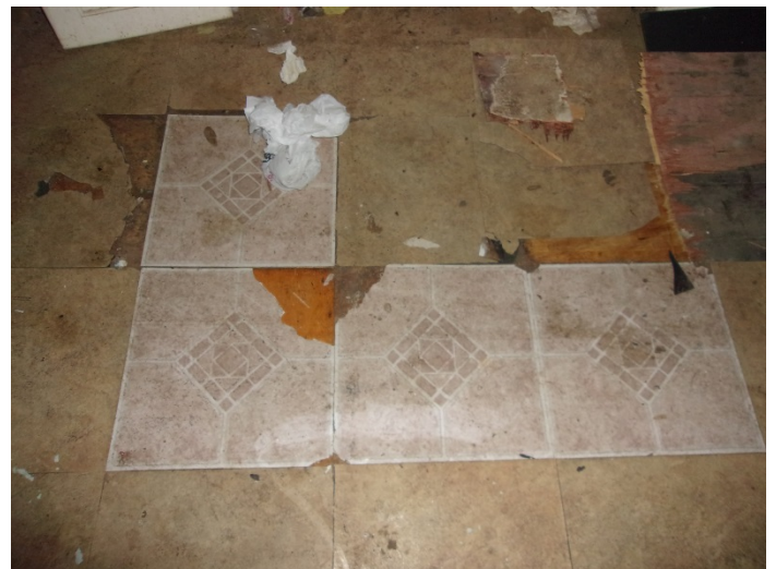
Photo 12 – 12" x 12" tan self-stick floor tile with mastic in the kitchen over wood (patch).
