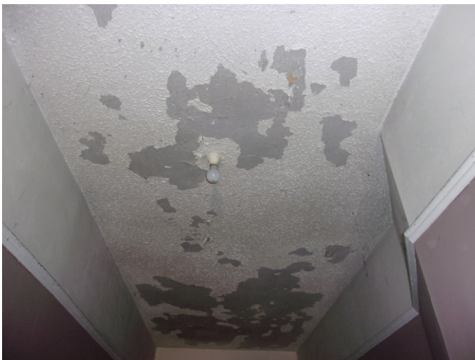
Photo 9 – Popcorn ceiling texture in the front hallway, front left bedroom & dining room.
