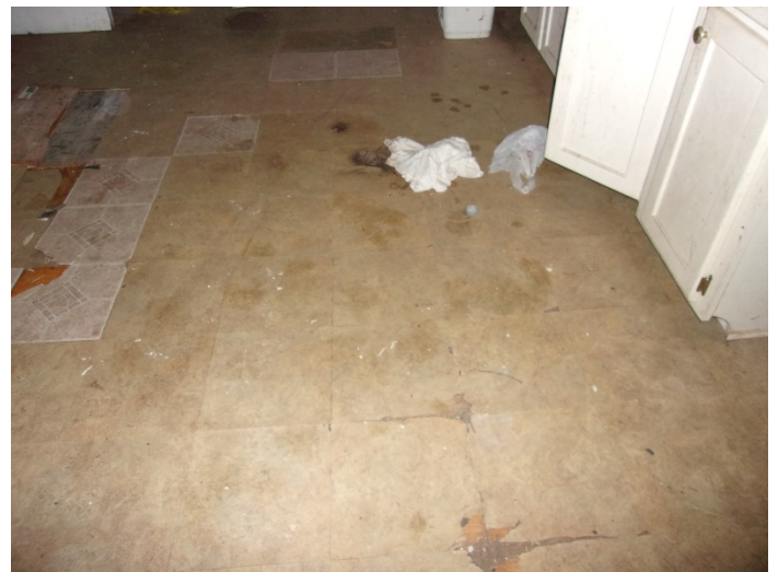
Photo 10 – 12" x 12" brown self-stick floor tile with no mastic in the kitchen over wood.
