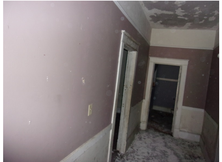
Photo 8 – Plaster with finish throughout
