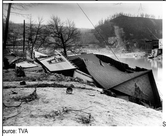
Figure 5.11 Historic Flooding in Anderson County
