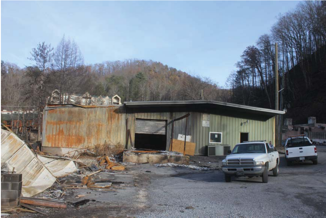
Photograph #1 – West Exterior Wall
