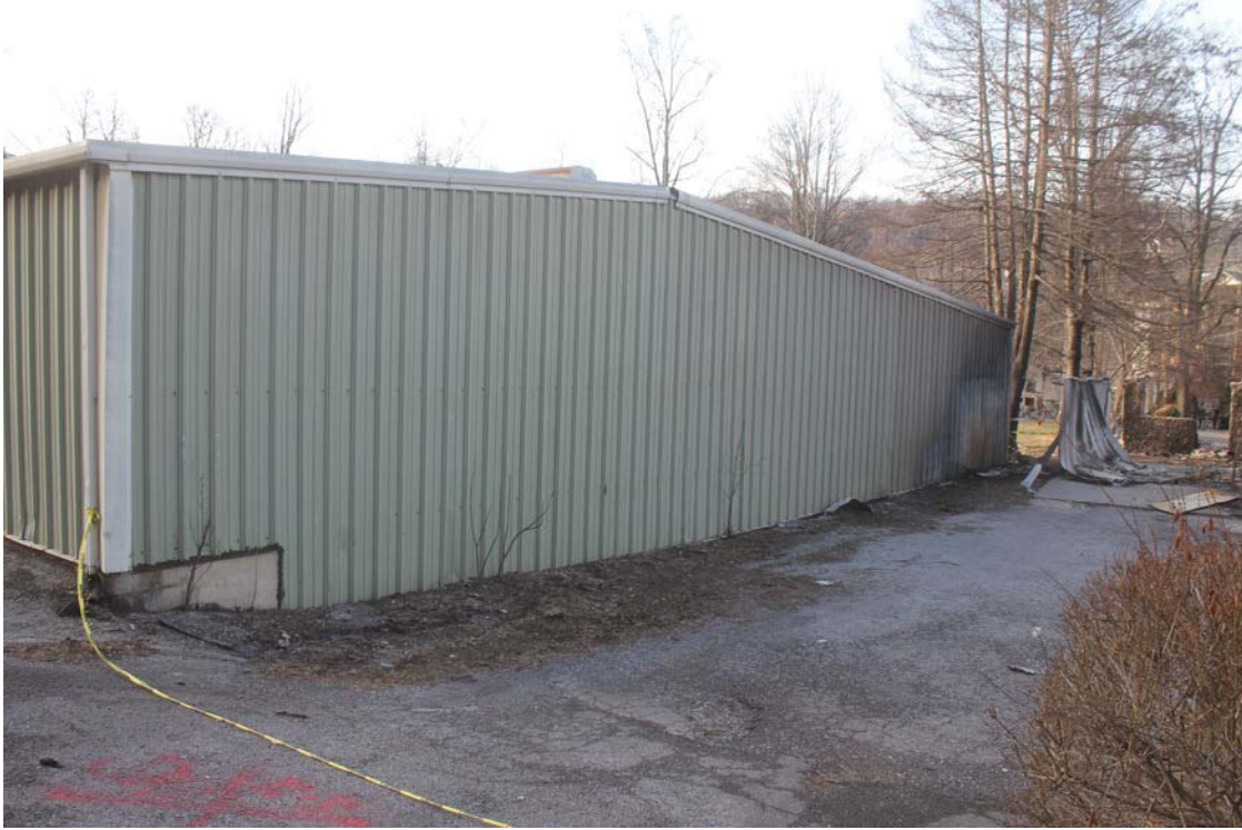
Photograph #3 – East Exterior Wall
