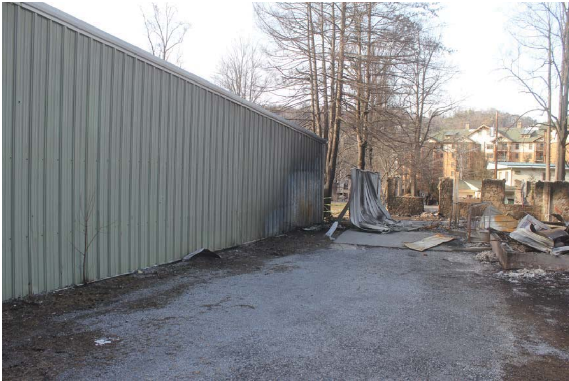
Photograph #4 – East Exterior Wall
