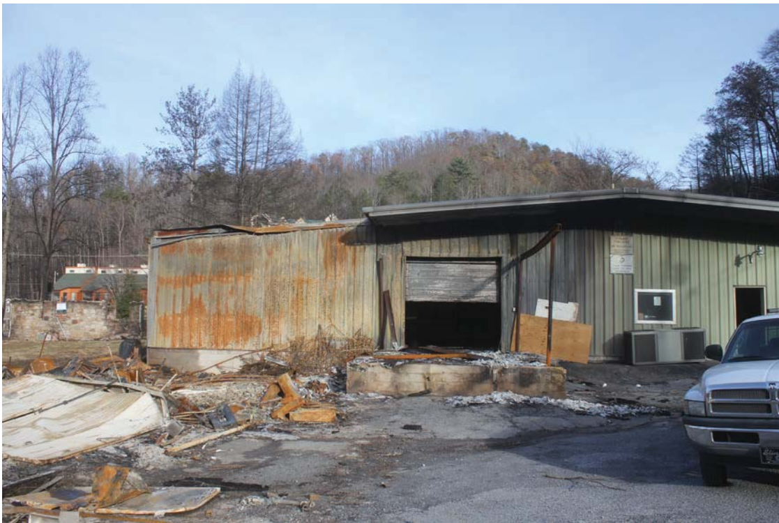
Photograph #2 – West Exterior Wall
