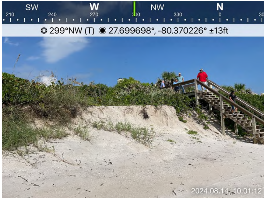
Photo 3. Taken from the beach looking west at potential access route. Note the beach access stairs remain open to pedestrian access throughout construction and the sea grape trees to be trimmed by the Contractor.
