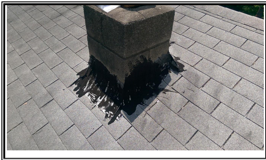
12. View of the chimney mastic at 650 California Blvd.
