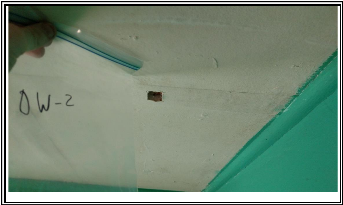
2. View of the drywall sample in kitchen at 650 California Blvd.
