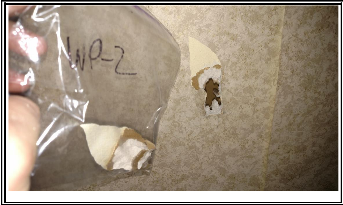
9. View of the wallpaper sample in the bedroom at 650 California Blvd.
