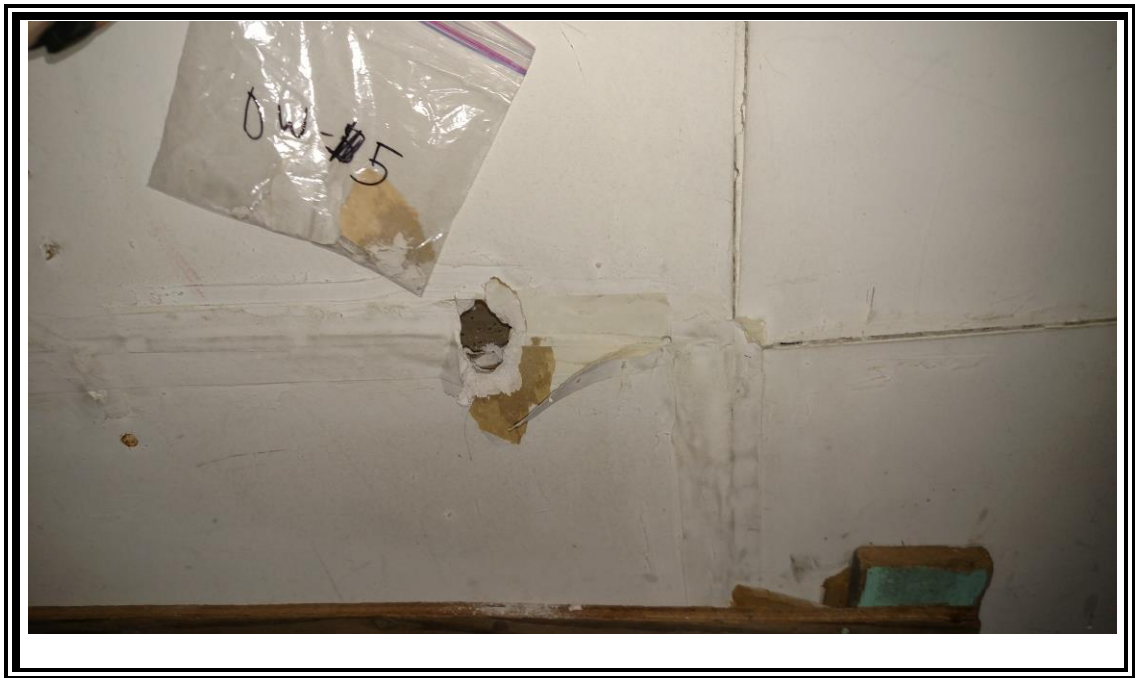
4. View of the drywall sample in the bedroom at 650 California Blvd.
