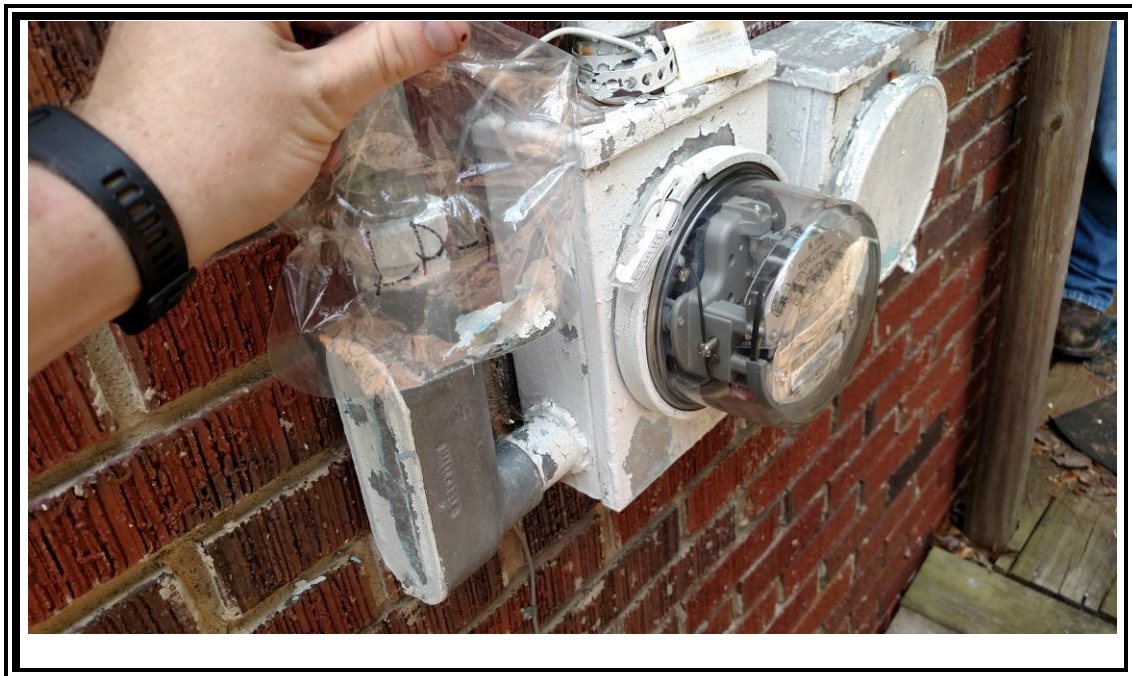
10. View of the lead-paint outside of 650 California Blvd.
