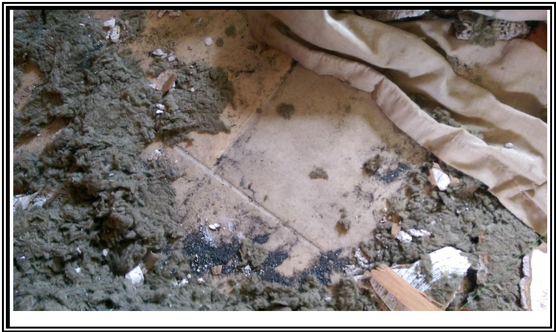
10. View of the bathroom flooring and insulation in 880 California Blvd.
