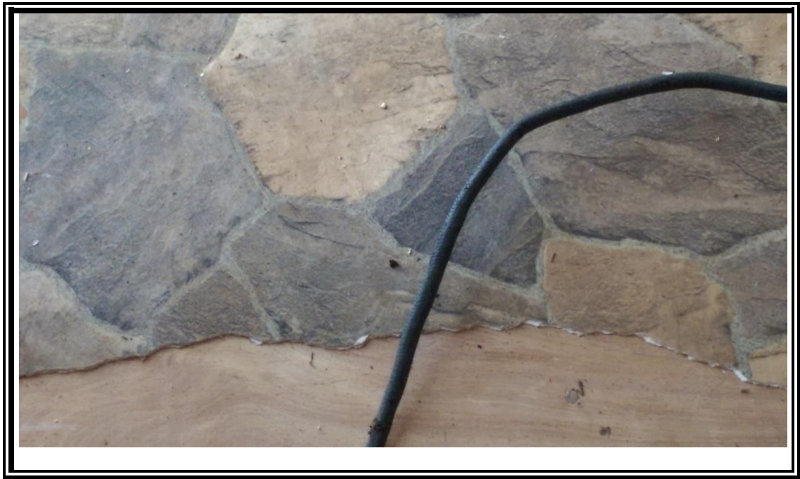
8. View of the kitchen flooring in 880 California Blvd.
