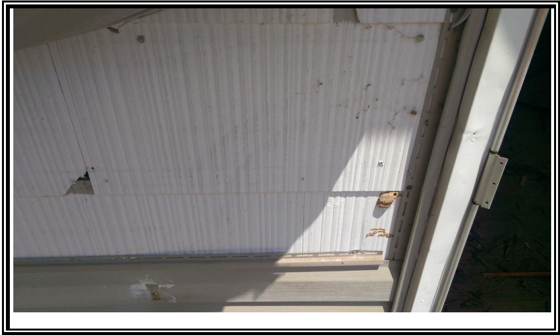
9. View of the Transite siding concealed by vinyl on 880 California Blvd.
