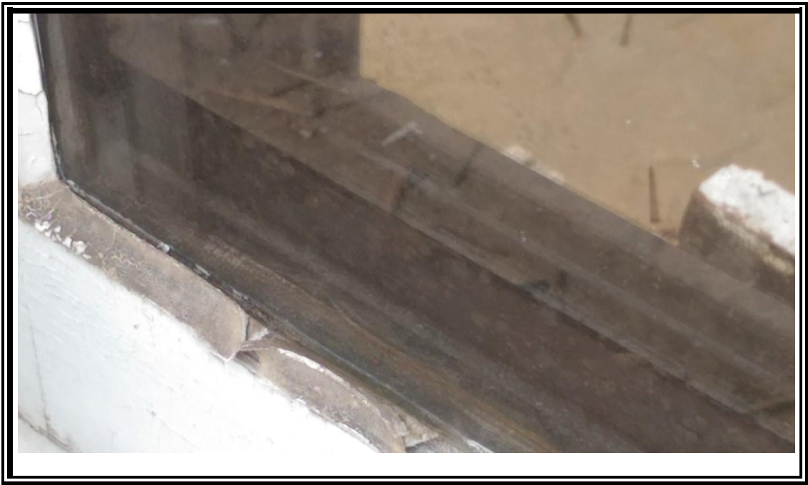
6. View of window glazing on the exterior of the 880 California Blvd. windows.
