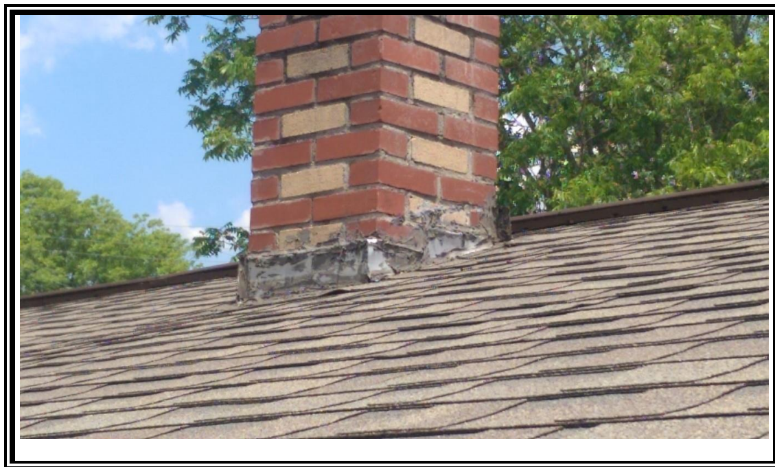
4. View of the chimney mastic at 880 California Blvd.
