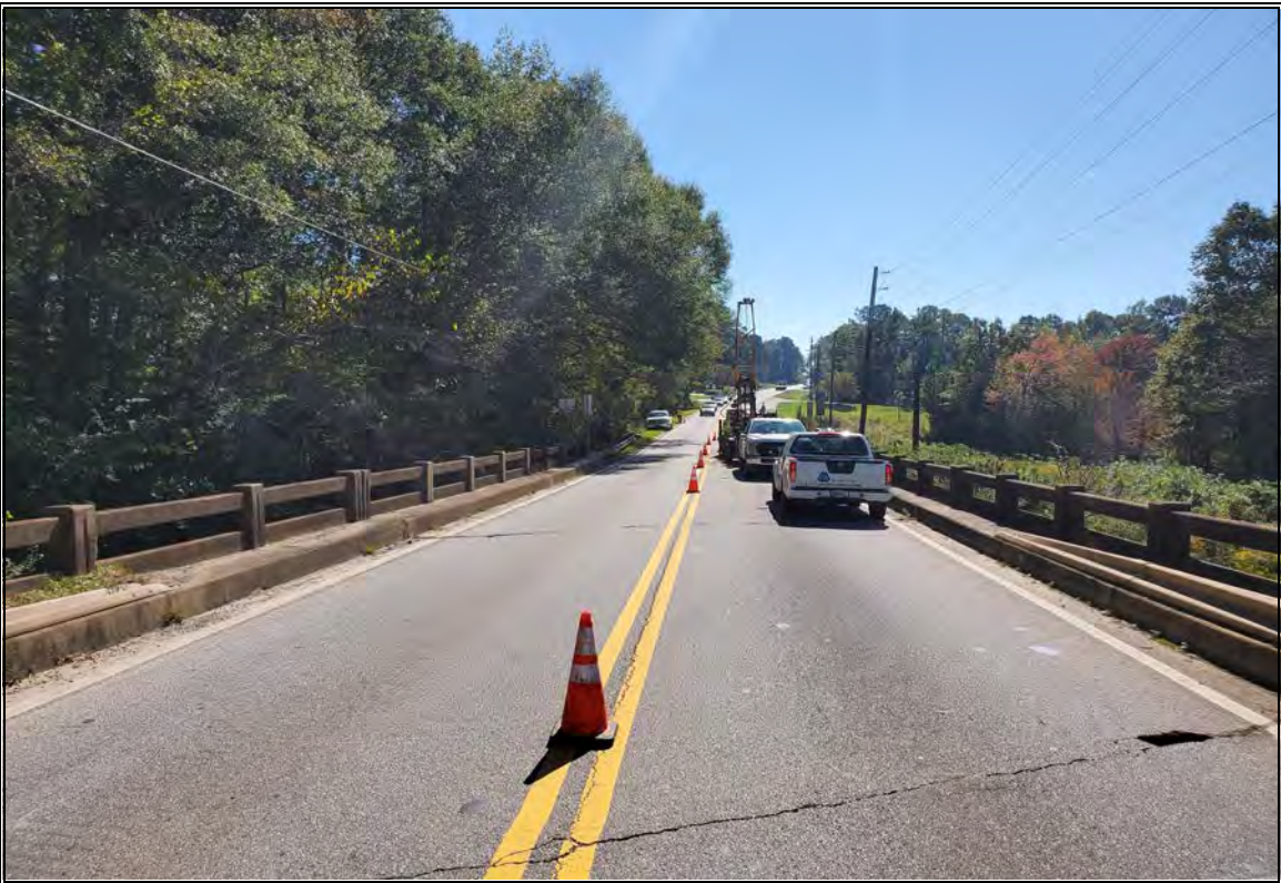
Looking in increasing station from proposed Bent 1, Sta. 108+00±, centerline
