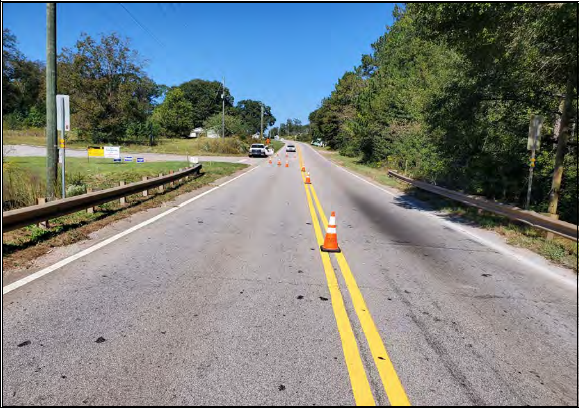
Looking in decreasing station from proposed Bent 1, Sta. 108+00±, centerline
