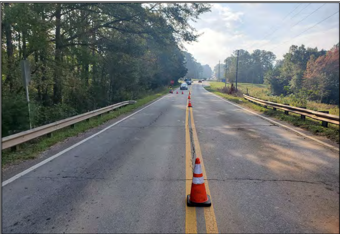
Looking in increasing station from proposed Bent 2, Sta. 109+50±, centerline
