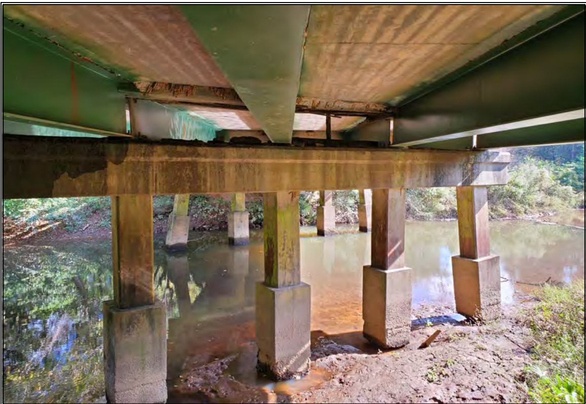
Looking in increasing station along existing bridge from Sta. 108+25±, centerline
