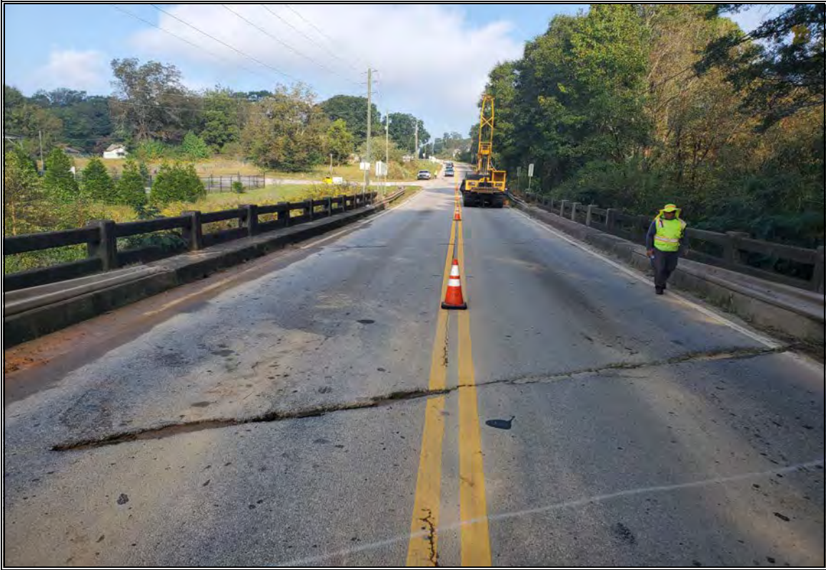
Looking in decreasing station from proposed Bent 2, Sta. 109+50±, centerline
