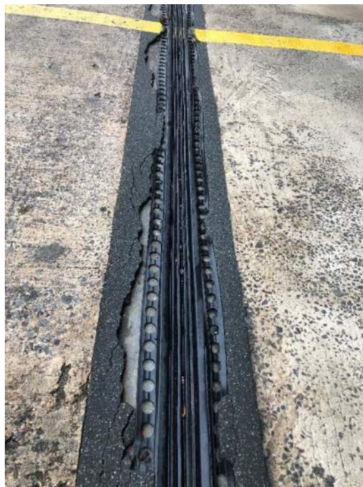
Photo 1A Closeup of Expansion Joint
