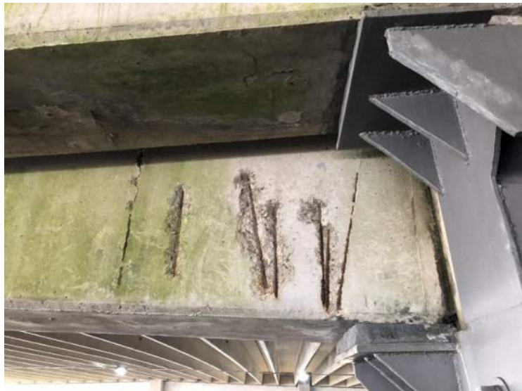
Photo 5C Beam Spalling
