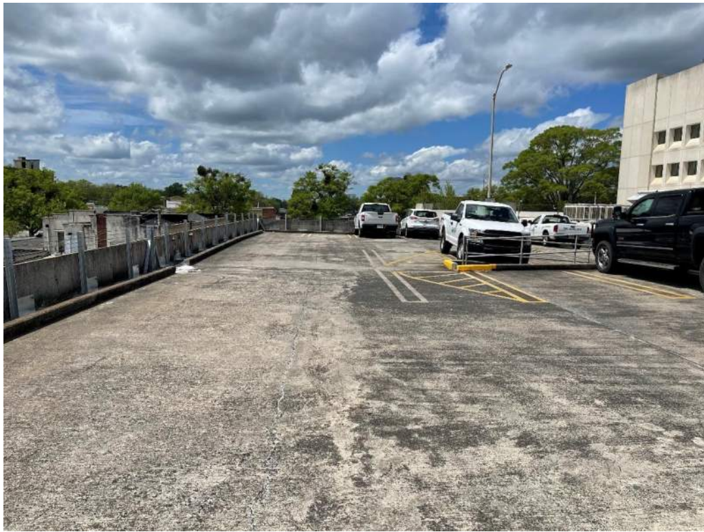
Photo No. 5: South end of Level 3 (view facing west)
