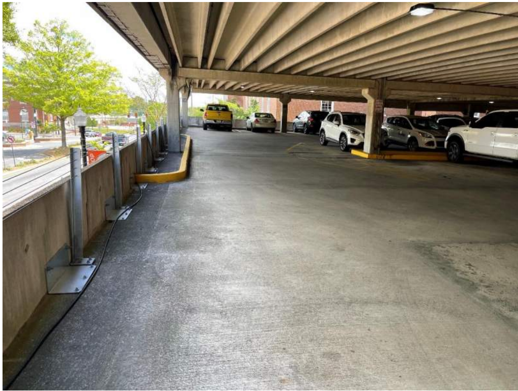
Photo No. 21: Level 2A facing east toward Level 1B
