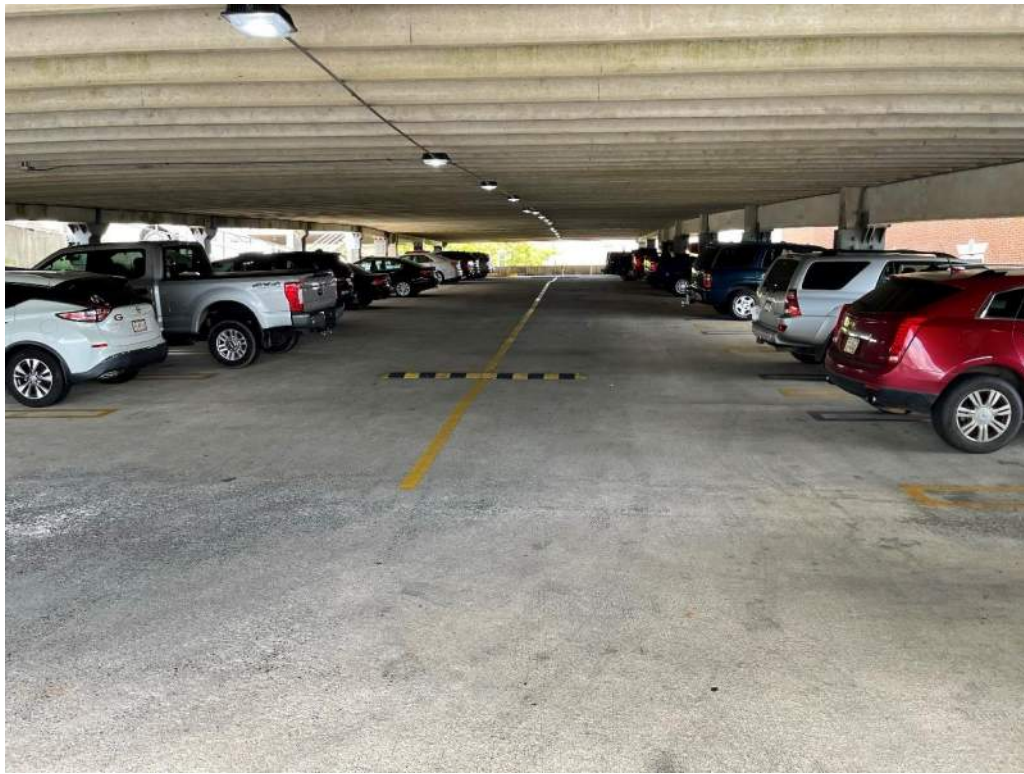
Photo No. 15: Level 2B ramp up – view facing north
