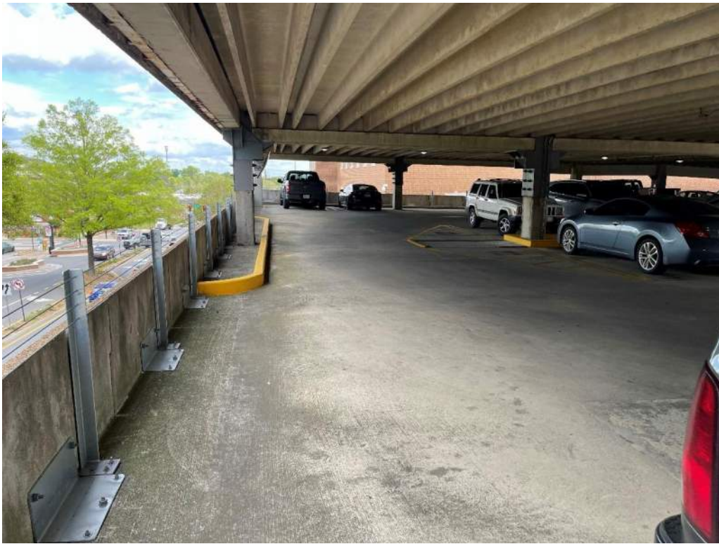
Photo No. 13: North end of Level 3A looking toward Level 2B
