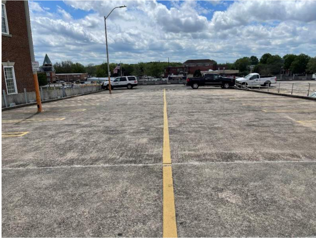
Photo No. 3: Overview of Level 3B (view facing south down ramp)
