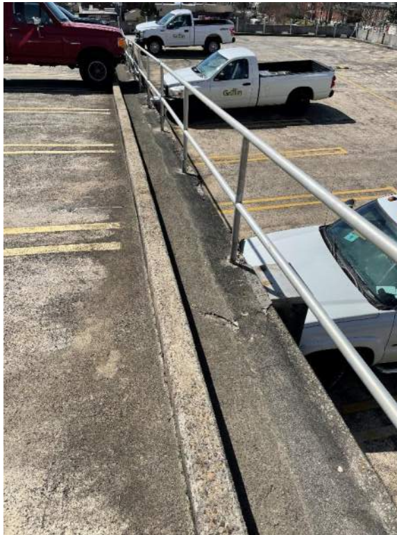
Photo No. 30: Aluminum guardrail along west edge of Level 3B
