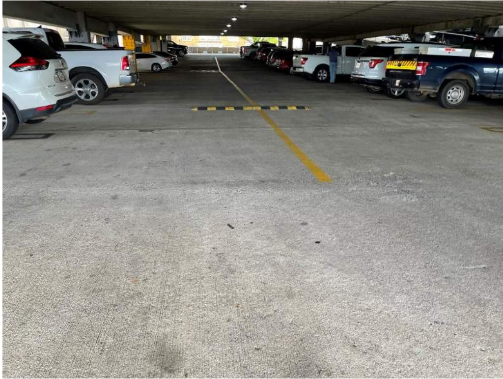
Photo No. 17: Level 2A ramp (view facing north)
