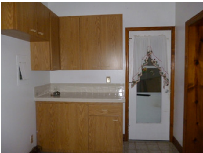
Kitchen and door to one-car enclosed carport
