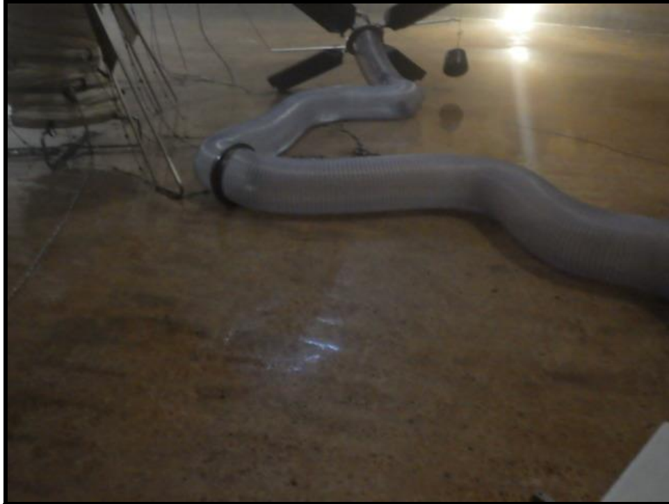
Photo 18. Interior – After Washout
