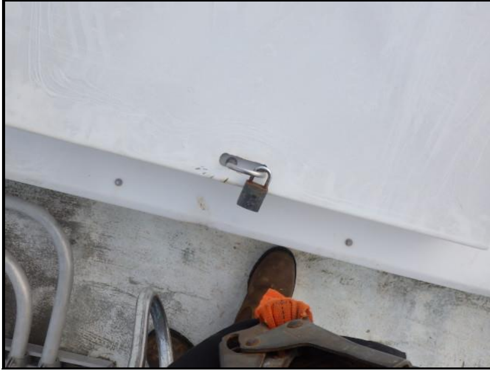
Photo 6. Locked top hatch
