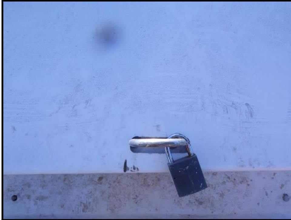
Photo 6. Locked top hatch
