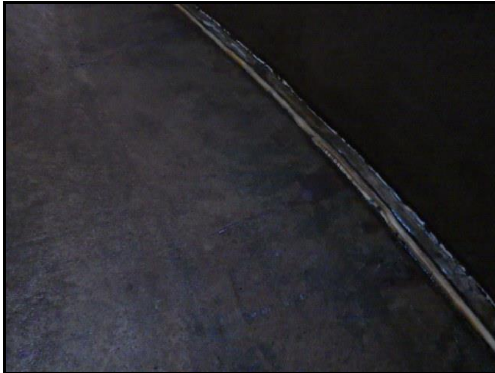
Photo 19. Interior Floor/Wall– After Washout
