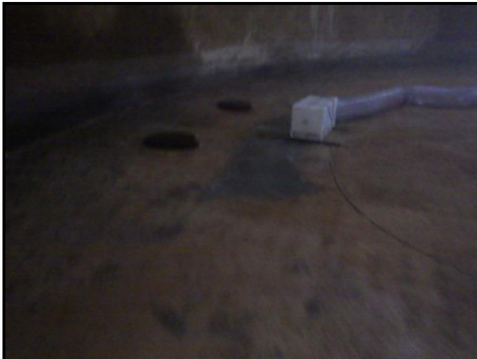
Photo 19. Interior Floor/Wall– After Washout
