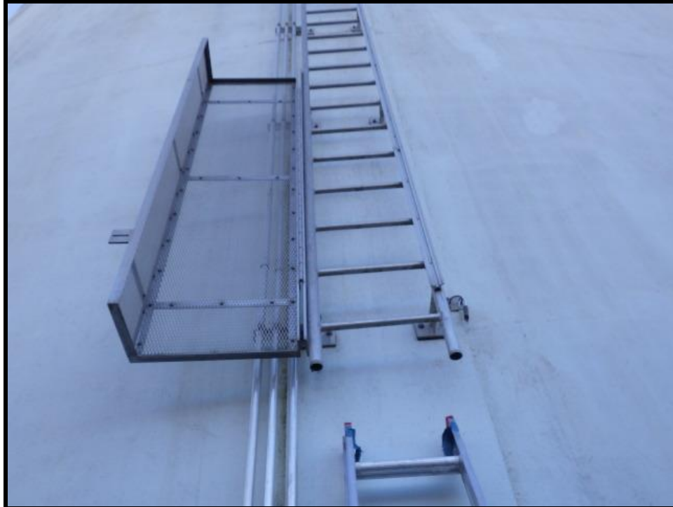
Photo 4. Access ladder & ladder gate
