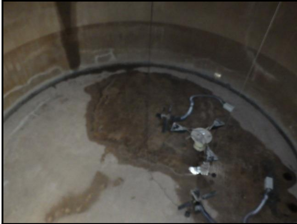
Photo 8. Interior before washout
