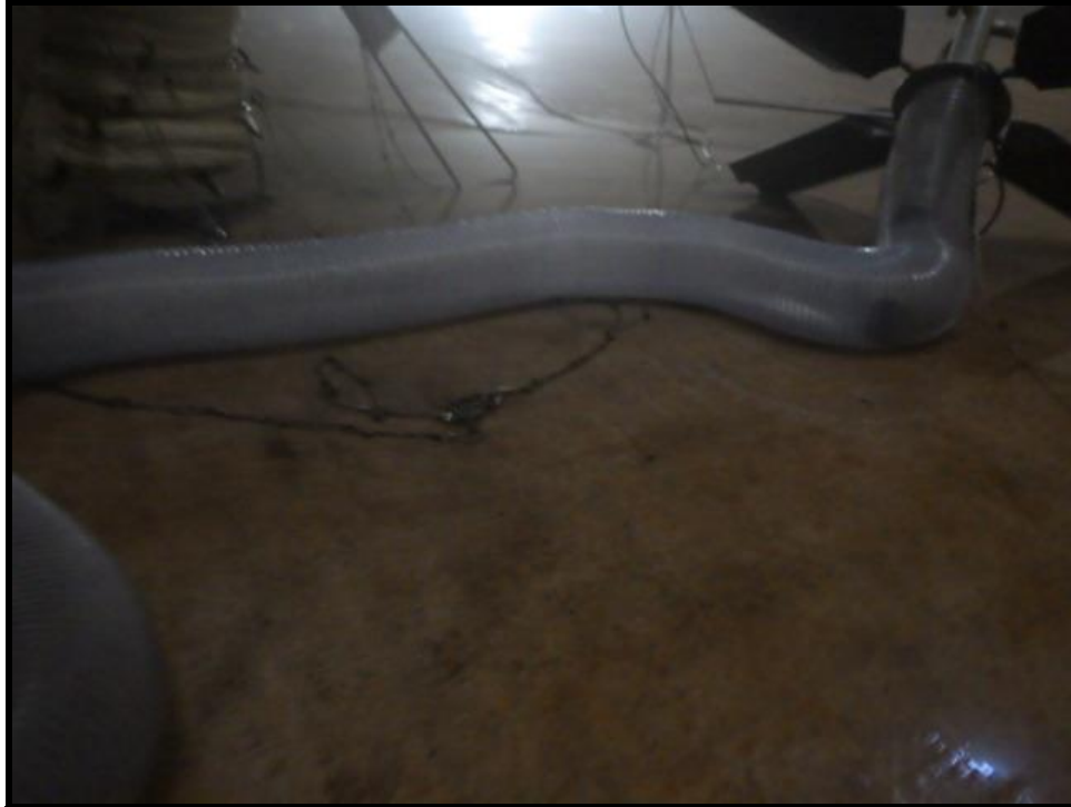
Photo 20. Interior – After Washout
