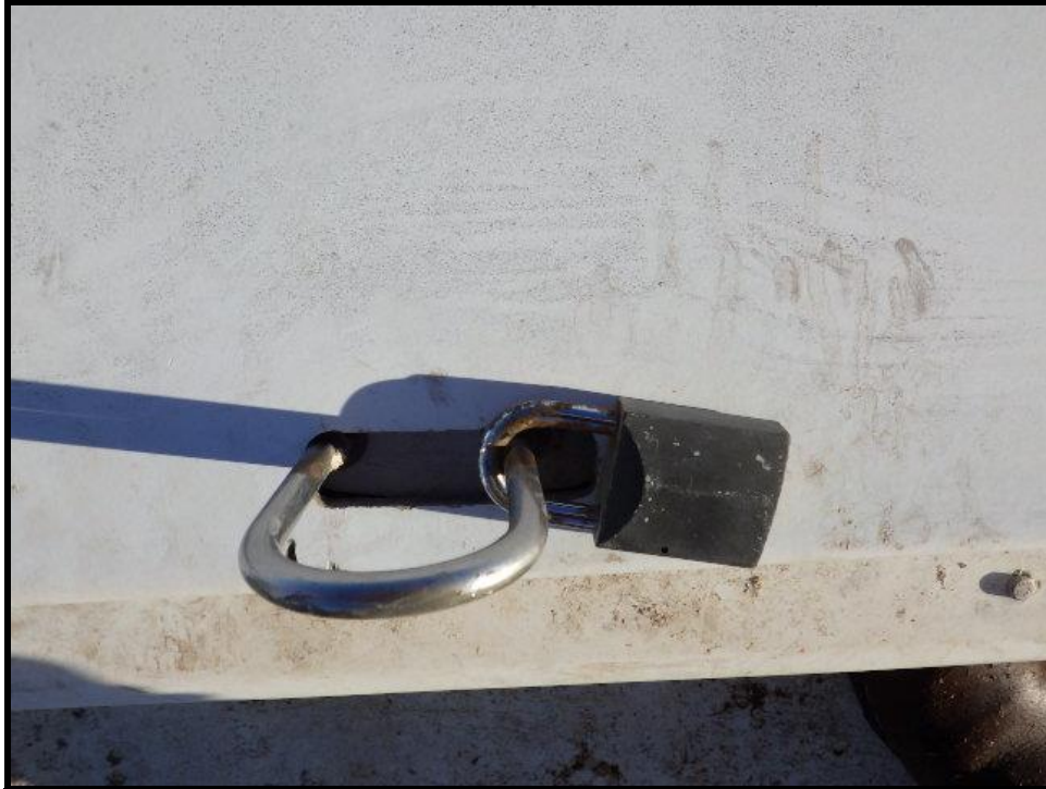
Photo 22. Top Hatch Locked
