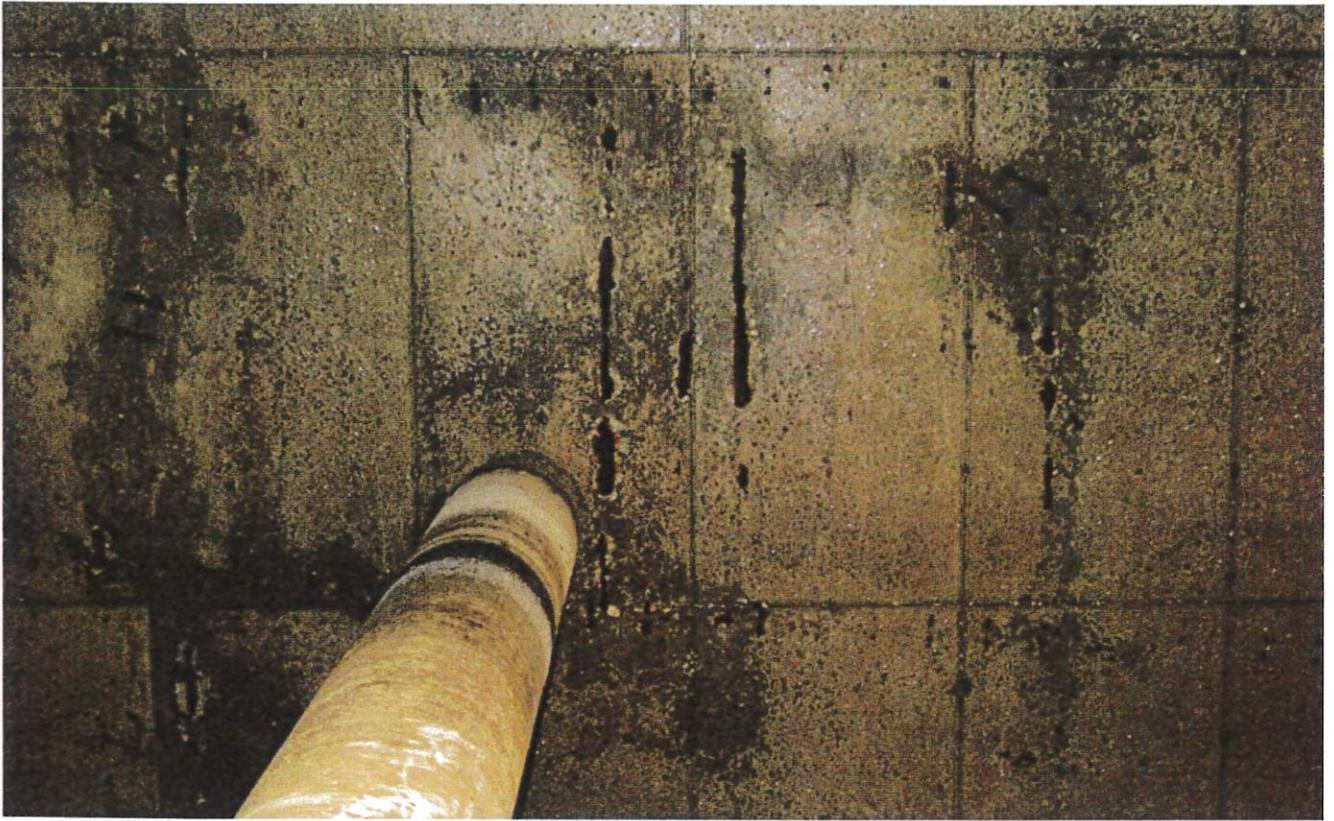
55. Exposed reinforcing bars in interior roof.
