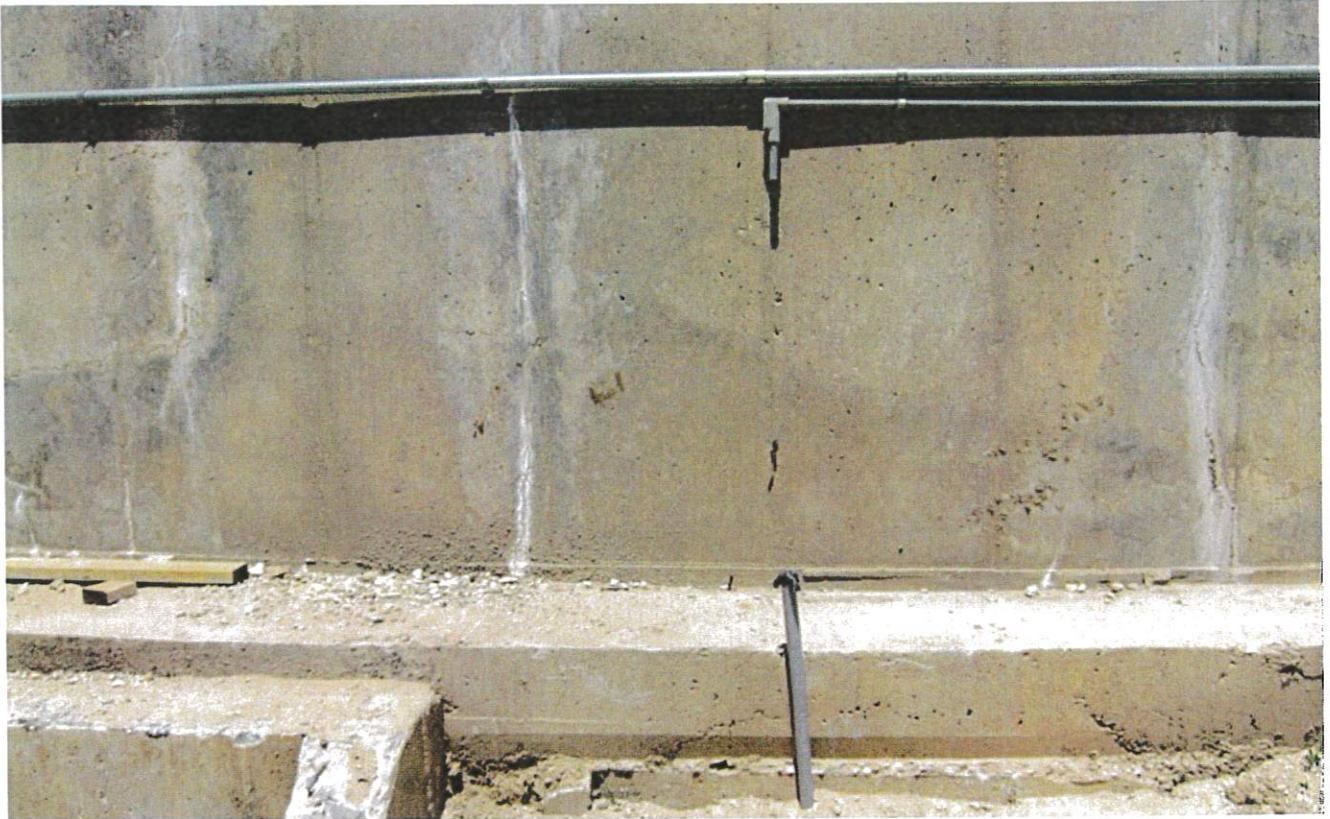
17. Concrete tank foundation and conduits on concrete shell.
