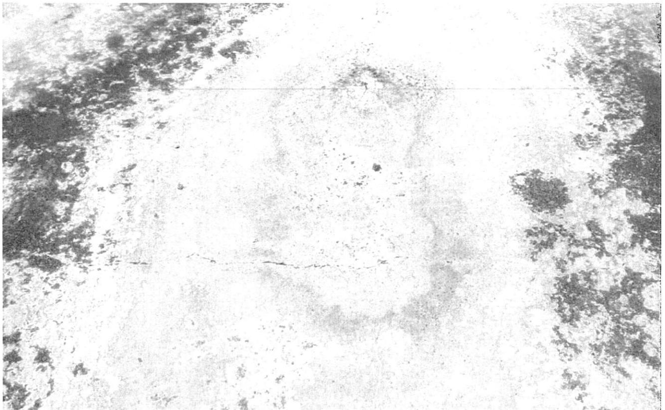
34. Evidence of ponding water on roof.
