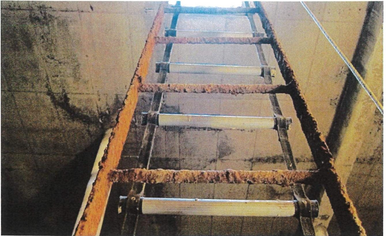
53. Corrosion and metal loss on interior ladder.
