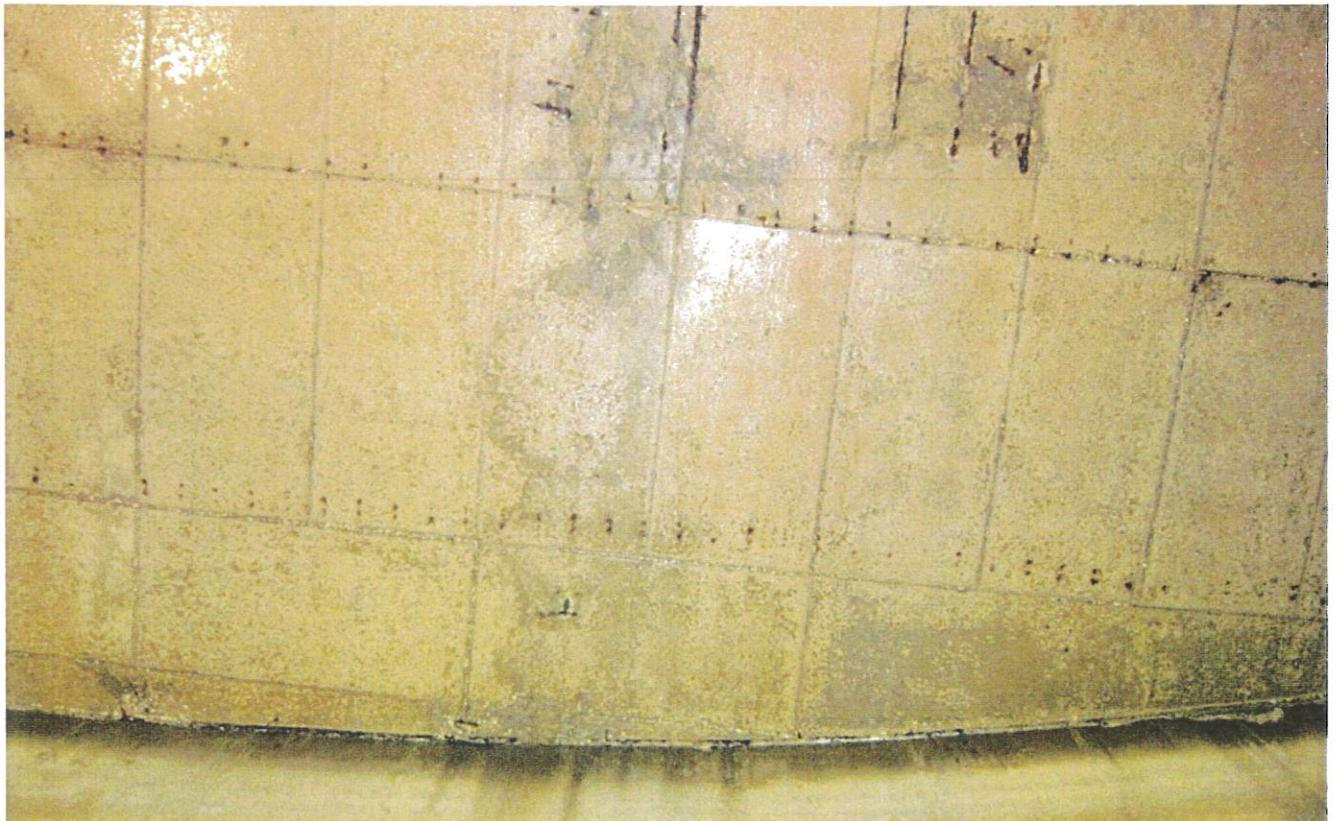
60. Exposed reinforcing bars and tie wires in interior roof.
