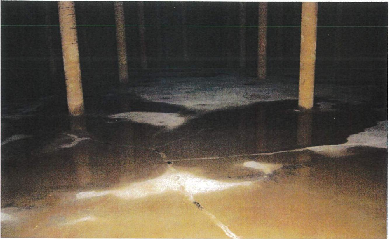
69. Interior floor and columns. Note cracking in floor.
