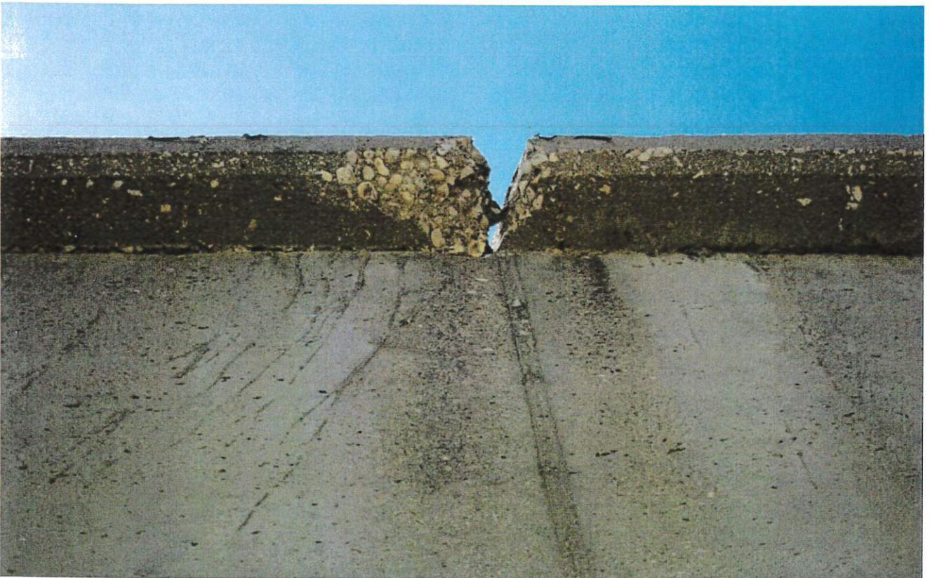
30. Chipped concrete at end of construction joint at roof perimeter.
