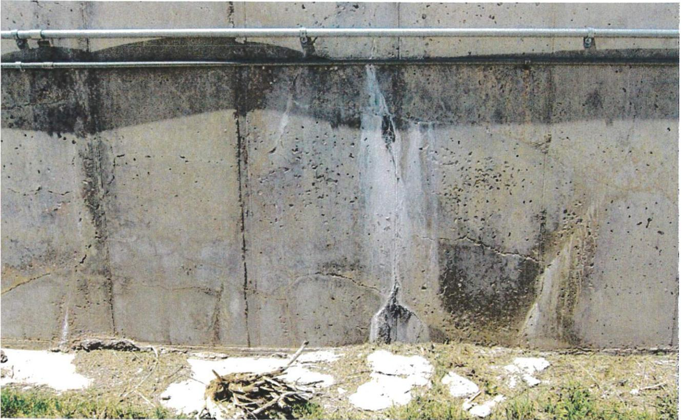
21. Cracks and efflorescence at bottom of shell.
